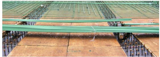
Figure 6 Photo showing temporary wood formwork installed on a steel plate I-girder bridge.
