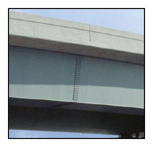
Figure 21 Photograph of a Box Girder Field Splice
