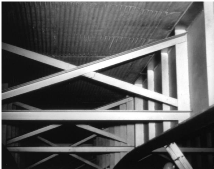
Figure 14 X-Bracing and Girders
