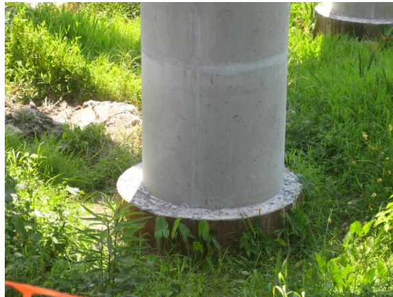
Figure 8 Single round column with an oversized, steel cased, drilled shaft.
