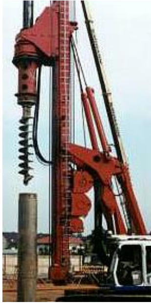
Figure 9 Drilled shaft drilling rig. Note the steel casing projecting above ground.
