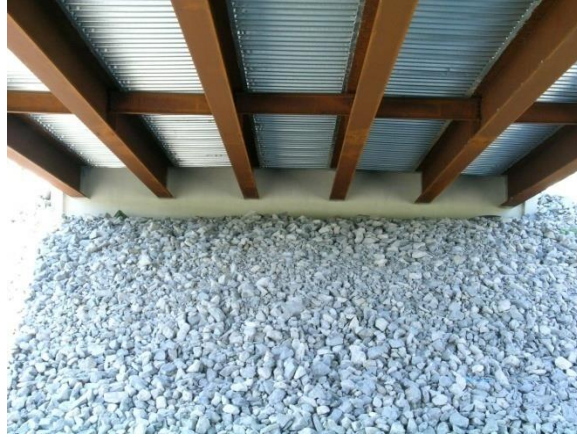
Figure 14 Photograph of a completed integral abutment.
