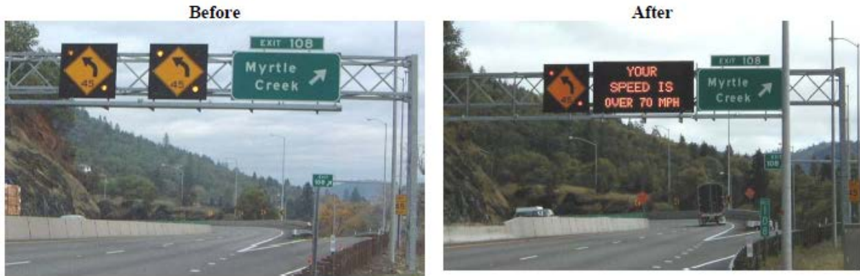
Figure 1. Photo. Northbound Interstate 5 DSFS systems in Oregon. (22)
