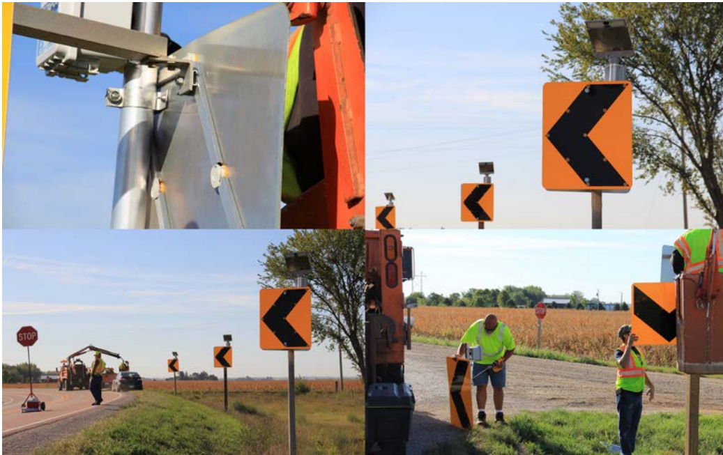
Figure 13. Photos. Installation of the SDCWS.
