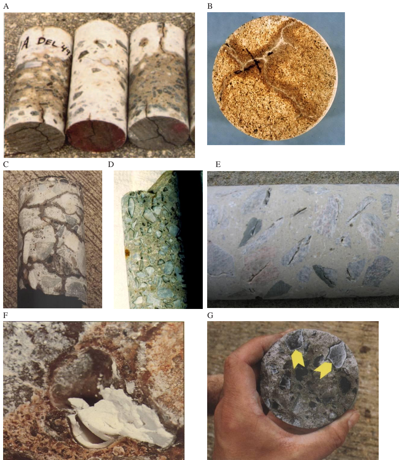
Figure C1. (A). Cores extracted from a concrete pavement affected by ASR and showing macrocracks penetrating from the upper and lower parts of the pavement. (B). Gel staining surrounding cracks and gel exudations at the surface of a core extracted from a sidewalk section affected by ASR (C). Fine cracking pattern showing up after rewetting of the core. (D). Dark rim around the periphery of reactive aggregate particles. (E). Macrocracks in reactive coarse aggregate particles. (F). Deposits of alkali-silica gel in a void on core surface. (G). Deposits of alkali-silica gel on the broken surface of a core extracted from a highway bridge structures affected by ASR.
