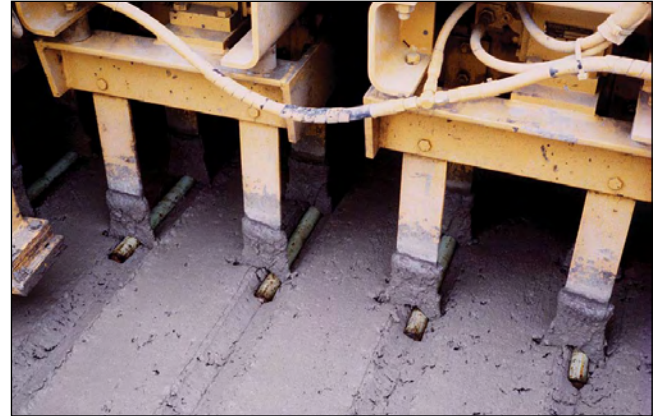
Figure 8-13. Dowel bar insertion equipment (ACPA)
