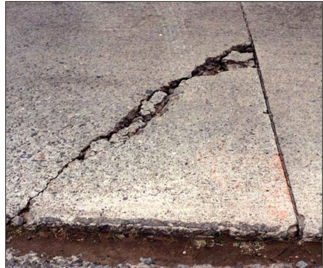
Figure 5-35. Corner break
