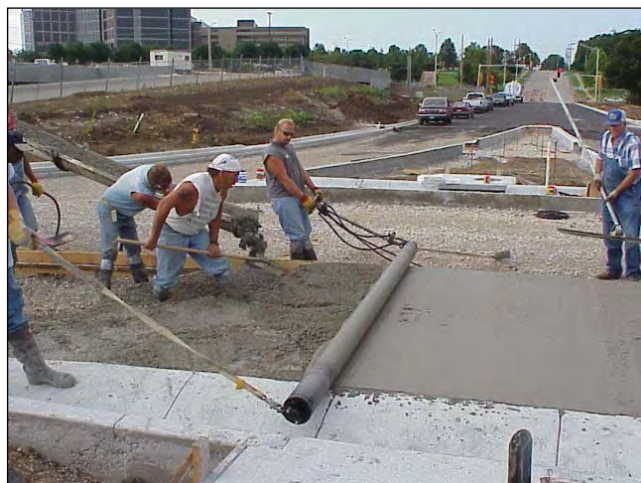
Figure 8-8. A roller screed (i.e., single-tube finisher) is one type of equipment that can be used to strike off the concrete in fixed-form placements. Others include vibratory screeds, form riders, and bridge deck finishers. (ACPA)
