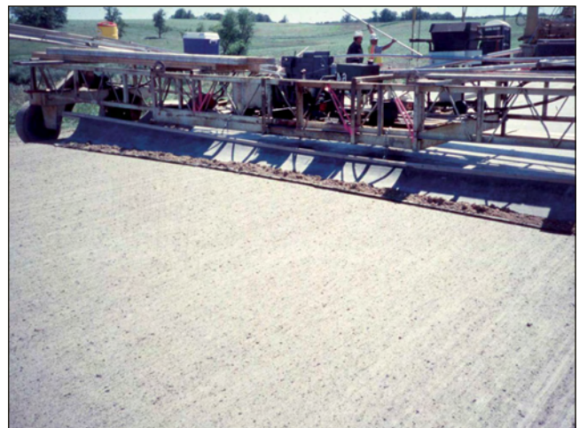
Figure 8-14. Artificial turf drag texturing rig, weighted with sand (ACPA)
