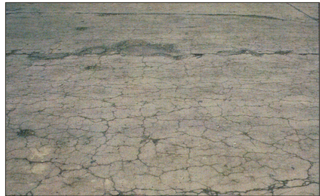
Figure 5-32. Map cracking
