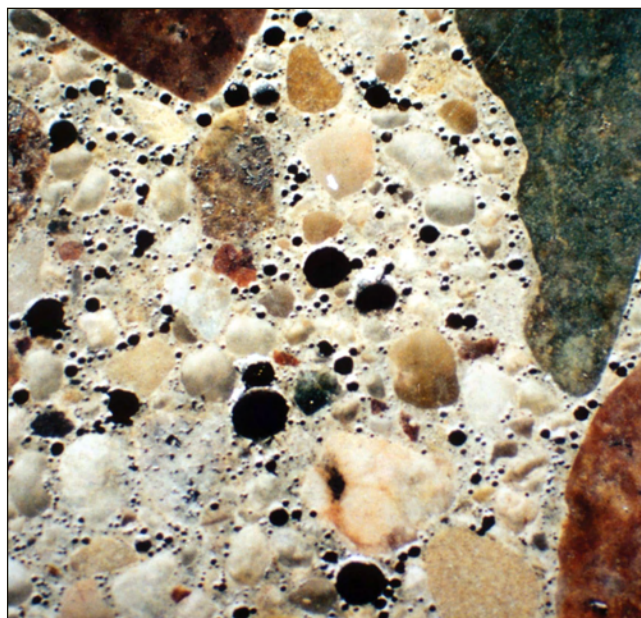
Figure 3-15. Entrained air bubbles in concrete (PCA)
