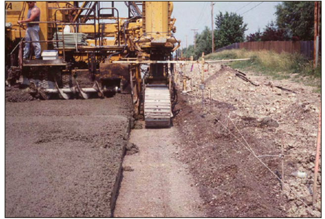
Figure 7-4. Trackline of slipform paving machine (ACPA)
