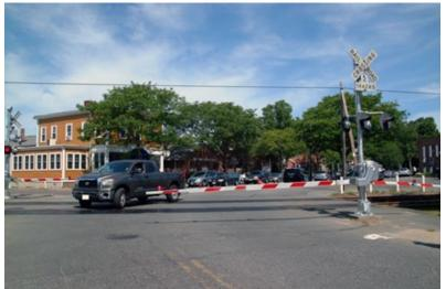
Figure 6. Photo. Highway-railway crossing and truck avoiding gate arms.
