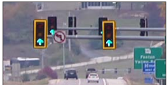
Exhibit 5: Signals at a displaced left-turn (DLT) intersection in Fenton, Missouri, have backplates with and without retroreflective borders. (Source: FHWA)
