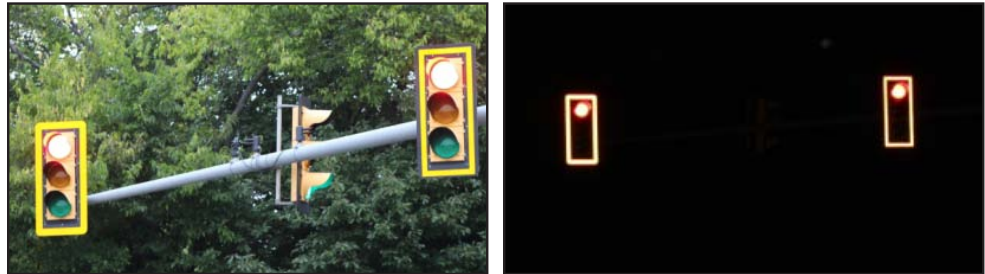
Exhibit 1: Retroreflective borders on backplates can provide a visual benefit during both daytime and nighttime conditions. (Source: VDOT)
