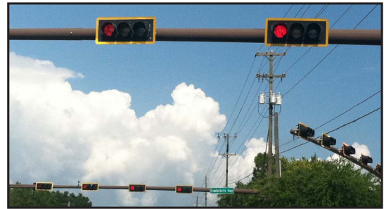
Exhibit 4: The retroreflective border provides a visual reference about the orientation of the signal, particularly during dark conditions. (Source: VHB)
