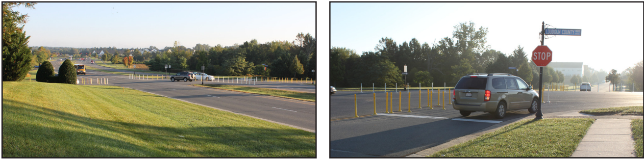
Exhibit 2: At this location, corridor access management measures were implemented to reduce crashes at median crossovers. Flexible post-mounted delineators were installed to restrict direct left turns from the side street. The photo on the left shows the main street and two vehicles in the median turning left onto the side street. The photo on the right shows how the delineators were placed to prevent vehicles from turning left through the median onto the main street. (Source: VHB)
