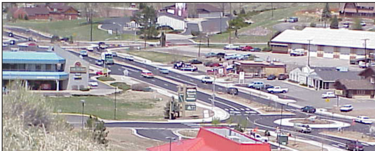
Exhibit 16: A series of roundabouts in Golden, Colorado. (Source: LSC Transportation Consultants, Inc.)
