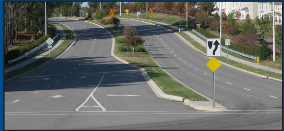
Exhibit 4: Raised median. (Source: VHB)
