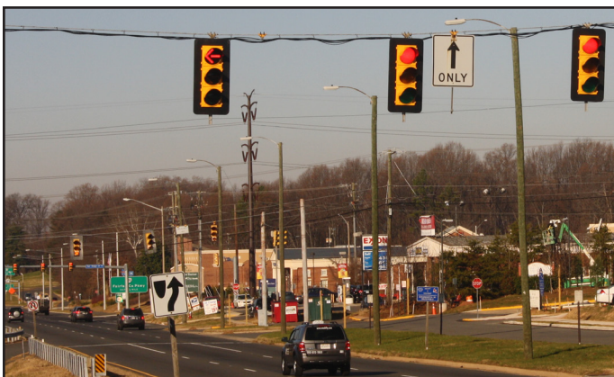
Exhibit 12: Example of closely spaced signals. (Source: VHB)
