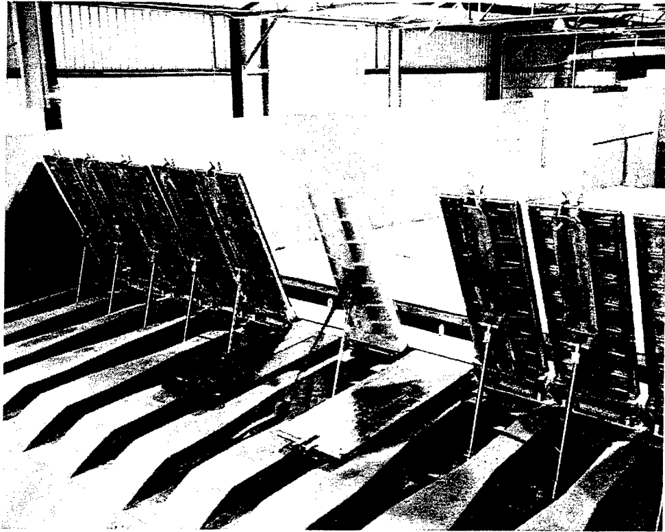
Figure 51. Completed gate installation in dry operation
