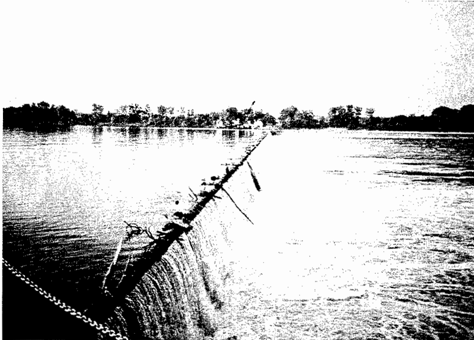
Figure 2. L&D 52 across the Ohio River
