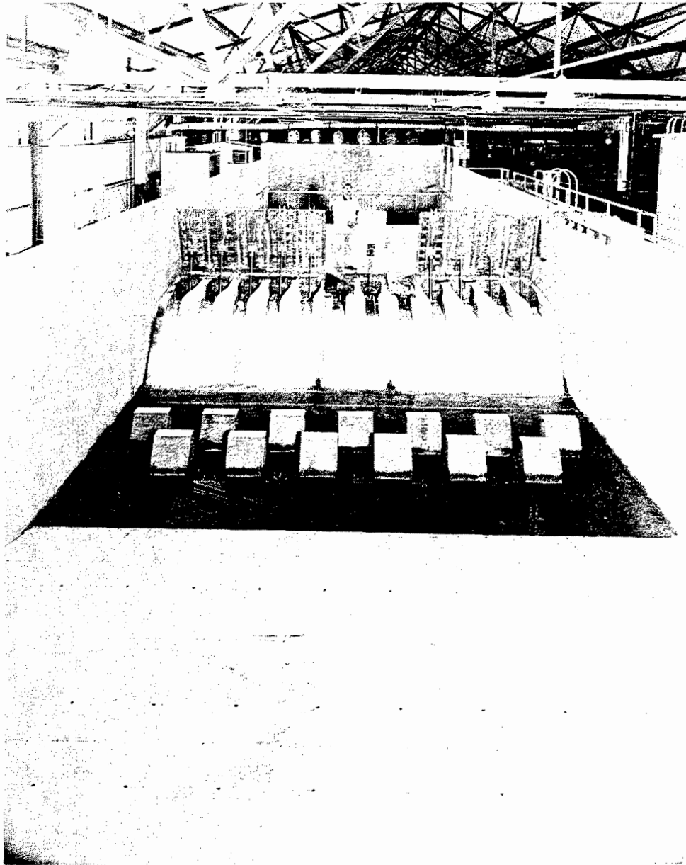
a. Dry bed looking upstream, general view
