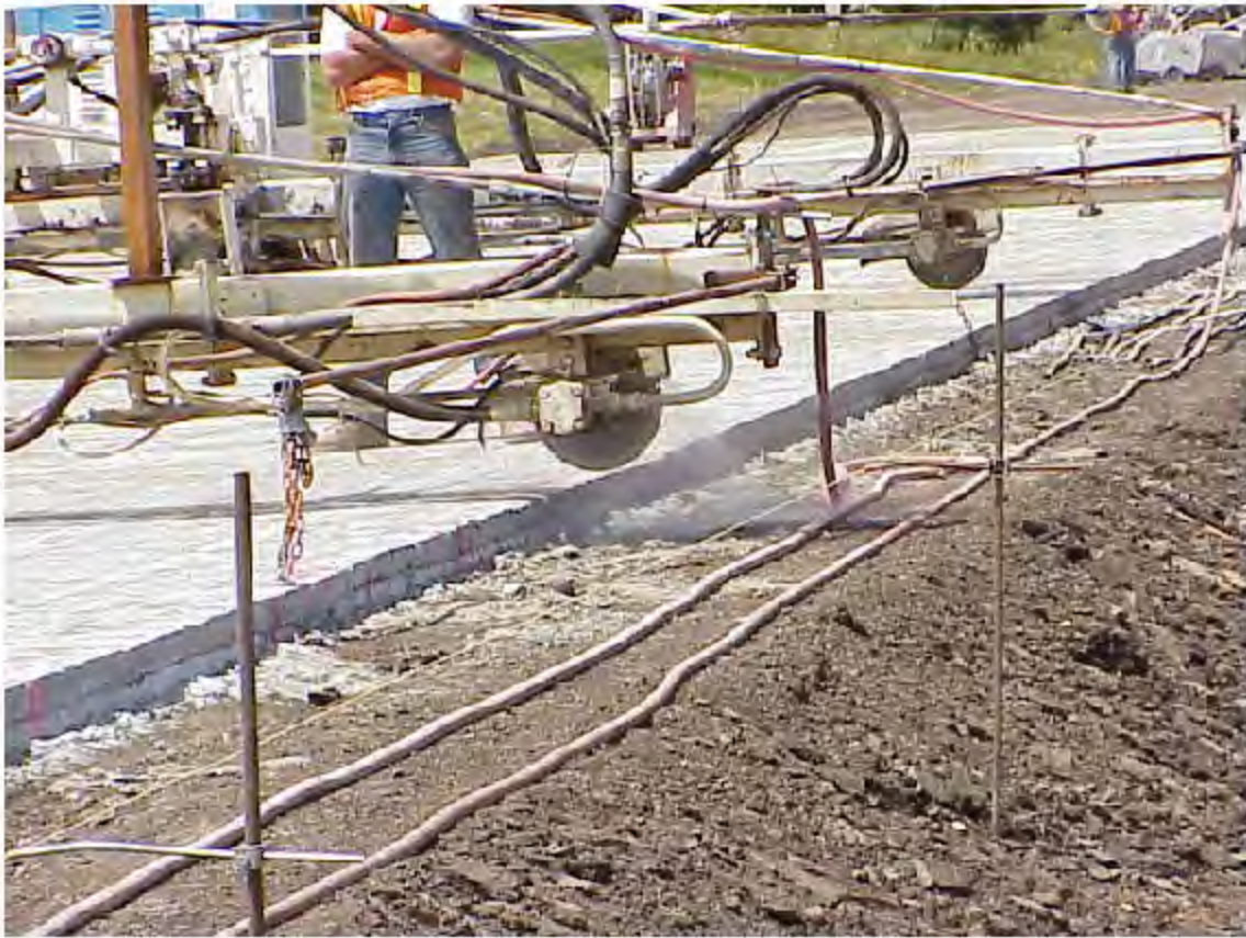
Whitetopping is a thin concrete overlay over asphalt pavement. It is used as a rehabilitation method.
