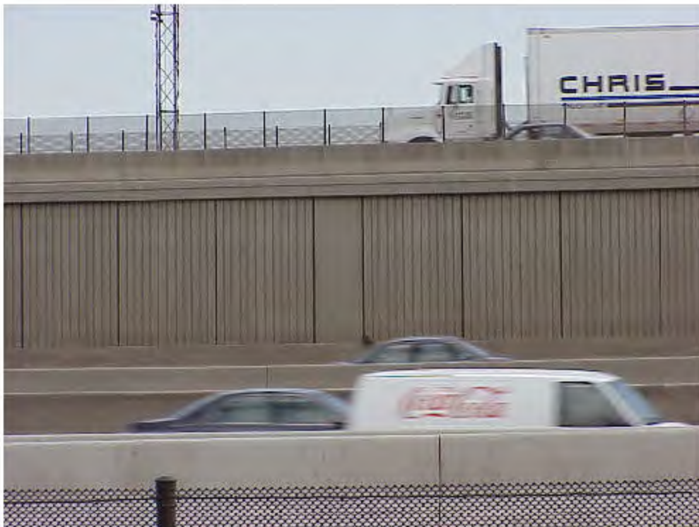
This mechanically stabilized earth wall, with independent full-height facing, is part of the ramp connecting N.B. I25 to I70 in Denver.
