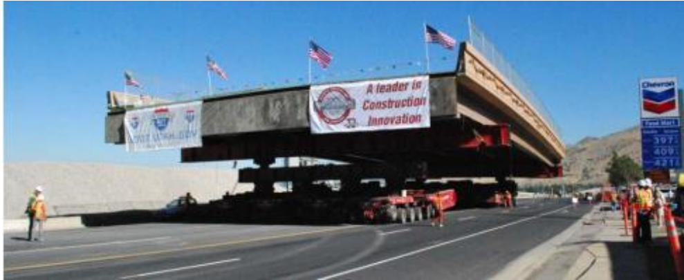
Figure 2: ABC superstructure positioning; bridges in Utah [5]
