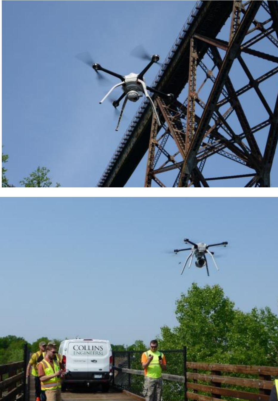
Figure 42: Drone used for bridge inspection by Minnesota Department of Transportation [110]
