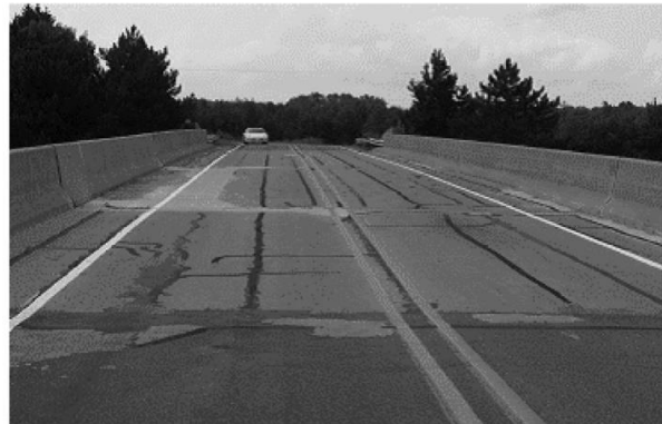
Figure 6: Longitude deck cracking of ABC closure joint [23]
