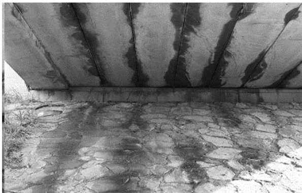
Figure 6: Longitude deck cracking of ABC closure joint [23]
