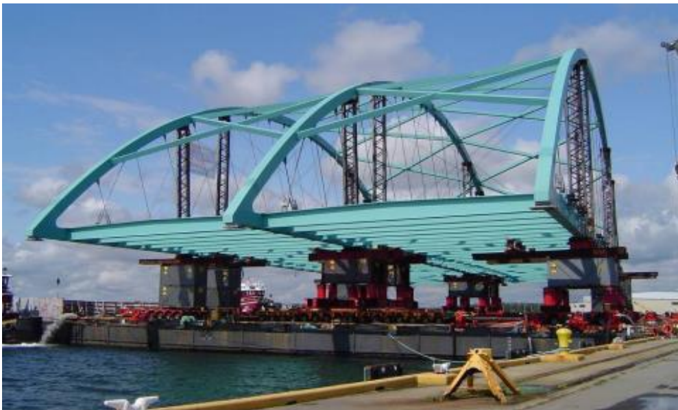
Figure 3: ABC superstructure positioning; Rhode Island (down) [5]
