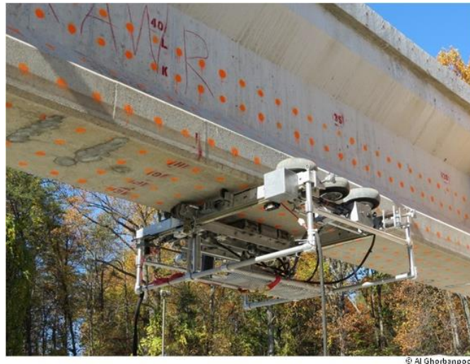
Figure 28: The Magnetic Flux Leakage testing for Bridge inspection [77]
