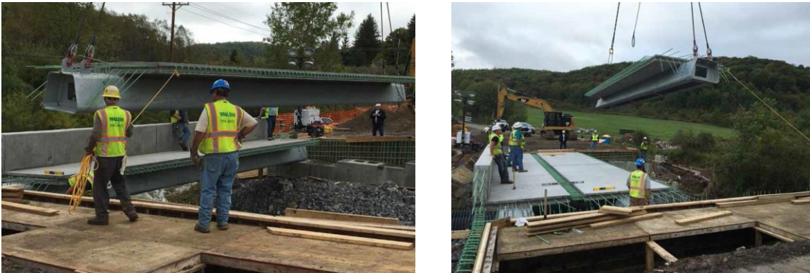
Figure 17. First FSPGBS constructed in Pennsylvania
