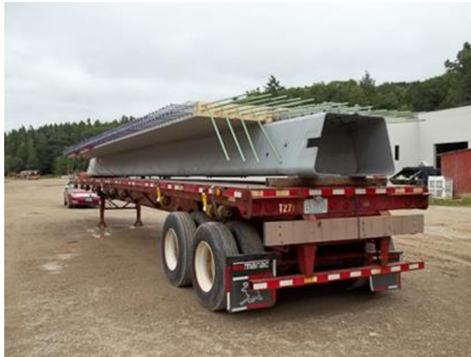
Figure 6. Pre-top folded plate girder.
