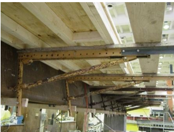
Figure 4. Conventional formwork for casting concrete deck.
