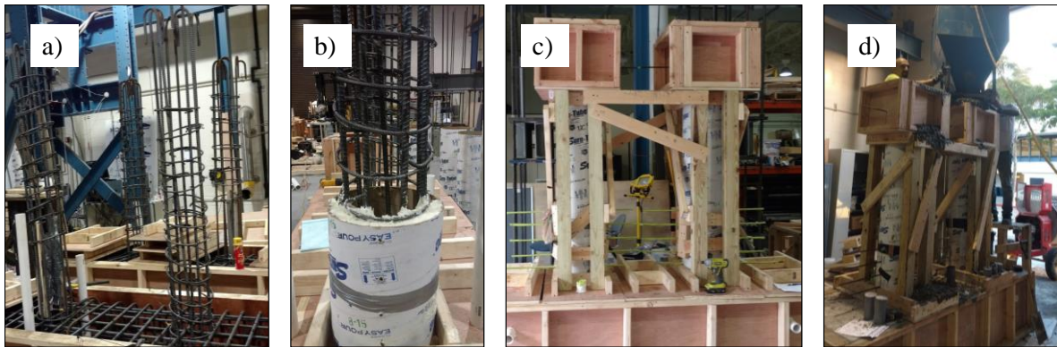
Figure 2. The construction process of a typical specimen: a) formwork and caging, b) simulating the damage, c) erecting the columns, and d) casting the concrete substrate.
