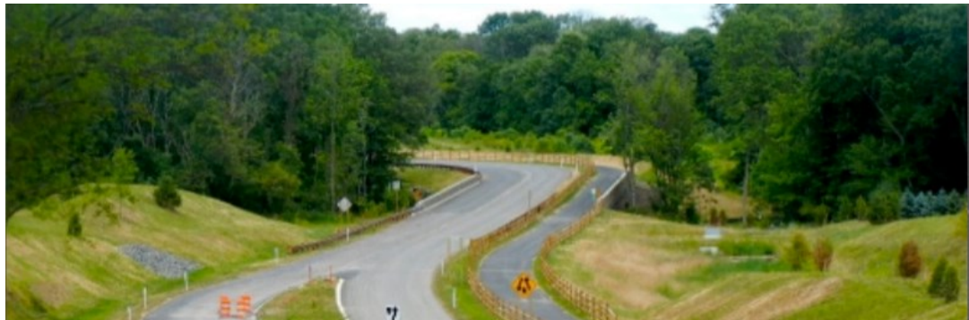
Figure 1: Pennsylvania DOT used the Smart Transportation process to rescope the Route 202 bypass from a four-lane controlled access freeway with a 65-mph design speed to a two-lane multimodal parkway with a 35-mph design speed. Lower speeds allowed for bending the road to fit into the surrounding context as well as eliminating the need to clear cut wide swaths of adjacent woodland. The design also eliminated large overpasses and reduced the number of lanes. Thus, the rescoping led to dramatically fewer impacts, and at less than one-half of the original project cost. Source: Al Biehler, Former Secretary, Pennsylvania DOT
