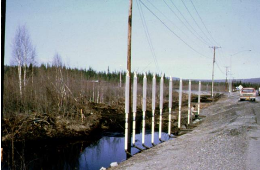
Figure 12: Thermosiphon Installation in Alaska. 31
