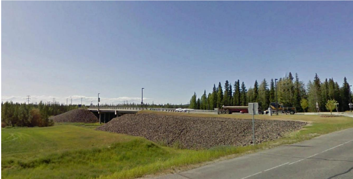
Figure 9: ACE on Thompson Drive embankment in Fairbanks, AK. 27
