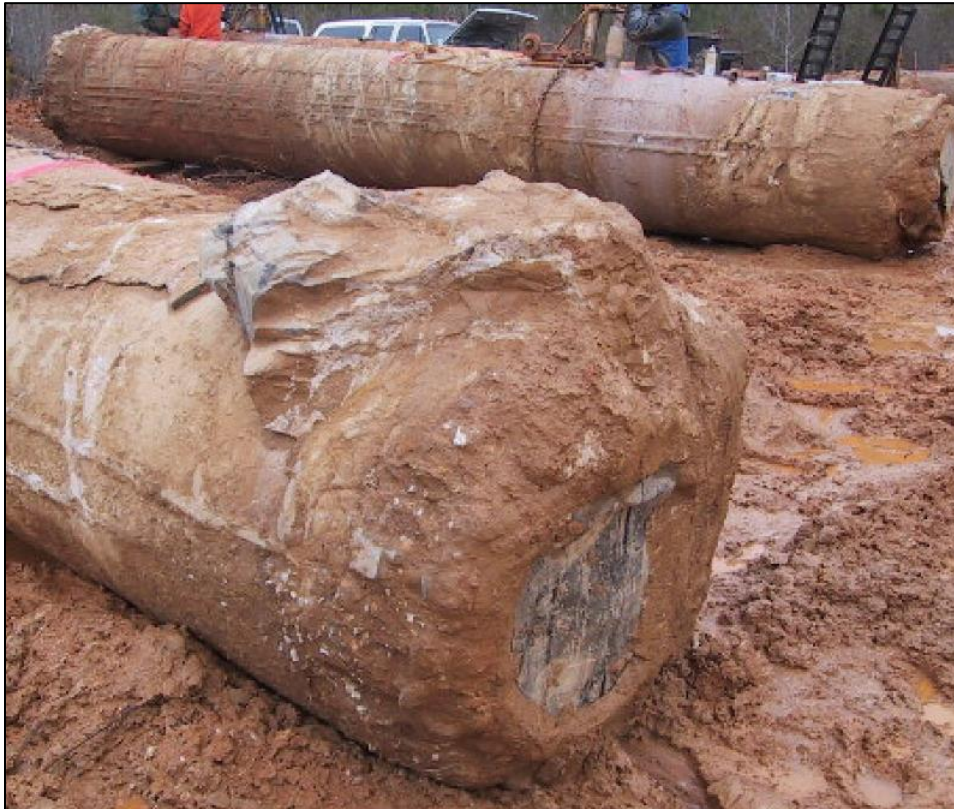
Figure 2.3: Photo of exhumed PGDS showing unintentional flow of grout up the side of the shaft (Brown et al., 2010).
