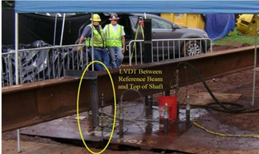
Figure 6.2: Photograph of an LVDT between the reference beam and the top of the shaft during grouting (courtesy of Applied Foundation Testing).
