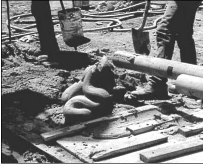
Figure 3.3: Limited mobility grout extruding from an injection pipe (Cadden et al., 2000).
