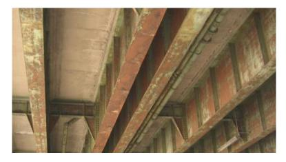
Figure 19. Photo. Closely spaced girders lead to difficult access for maintenance activities.
