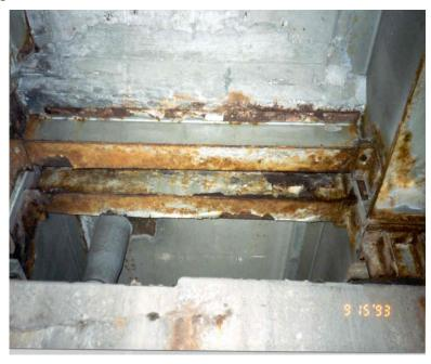
Figure 16. Photo. Steel directly beneath transverse expansion joints that have leaked corrosive runoff from the deck.
