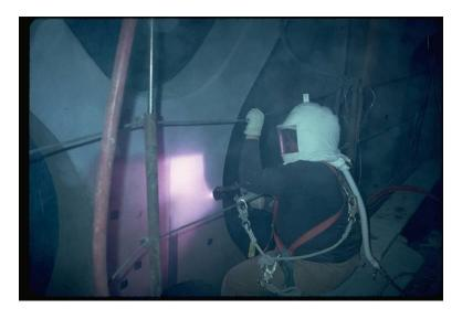
Figure 5. Photo. Metalizing of a bridge member in the field (photo courtesy of R. Kogler).
