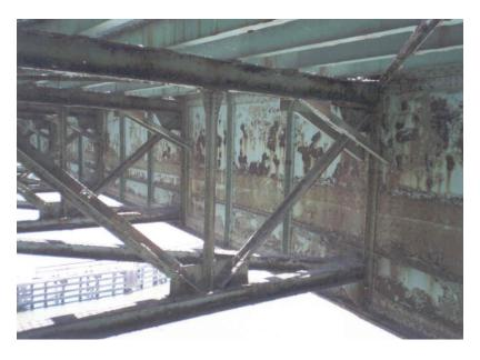
Figure 20. Photo. The area under an open grid deck acting as one large leaking joint.
