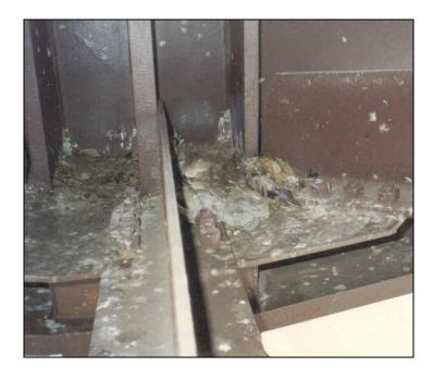
Figure 37. Photo. Debris accumulation at a lateral gusset plate detail.
