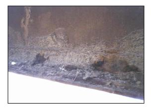
Figure 28. Photo. Heavy corrosion of bottom flange and web due to collection of poultice.
