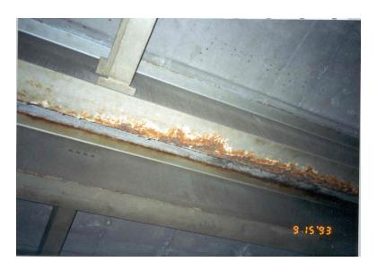
Figure 17. Photo. Steel directly beneath longitudinal expansion joints that have leaked corrosive runoff from the deck.
