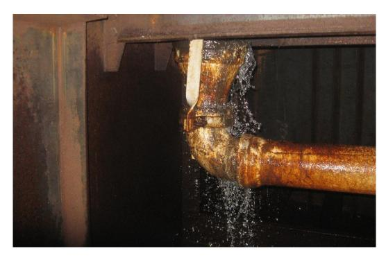
Figure 22. Photo. Clogged drain leaking water onto superstructure.
