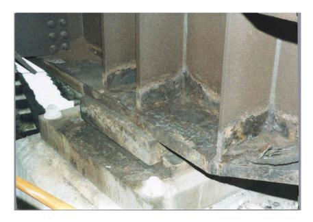
Figure 34. Photo. Girder end on a bearing below a leaking deck joint. Horizontal flange and vertical stiffeners create an excellent trap for debris and moisture.
