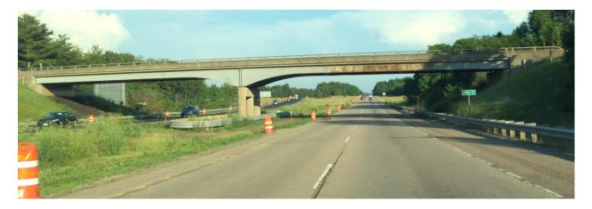
Figure 26. Photo. Accelerated corrosion on the inbound fascia girder of a grade separate structure, particularly over the right travel lane.
