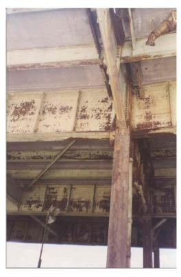
Figure 21. Photo. Missing portion of deck drain downspout.
