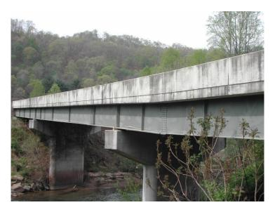
Figure 14. Photo. Bridge in West Virginia with a single-coat inorganic zinc-rich paint system after 25 years.
