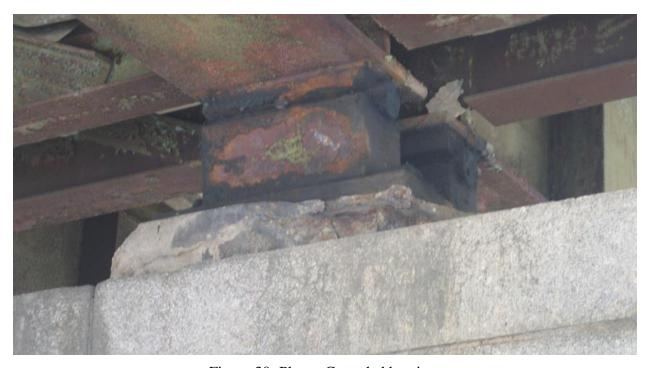
Figure 30. Photo. Corroded bearing.
