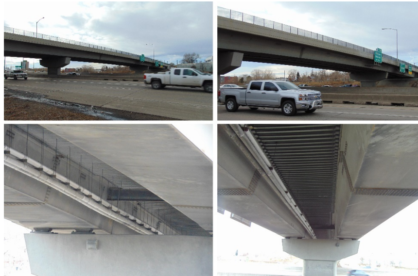
Figure 3.1 Pictures of the bridge used in this case study
