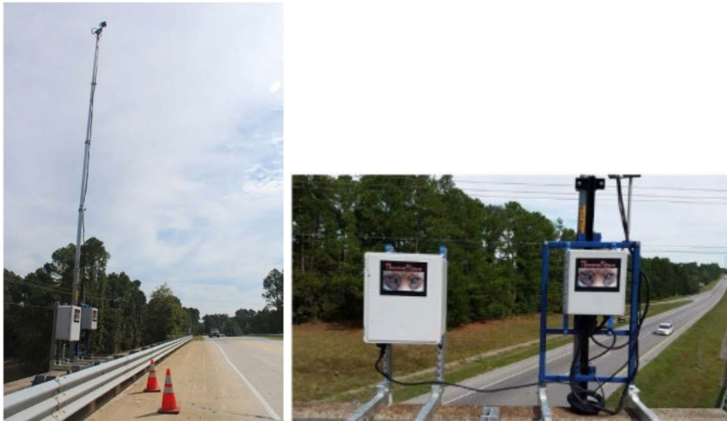
(b) view from bridge deck
