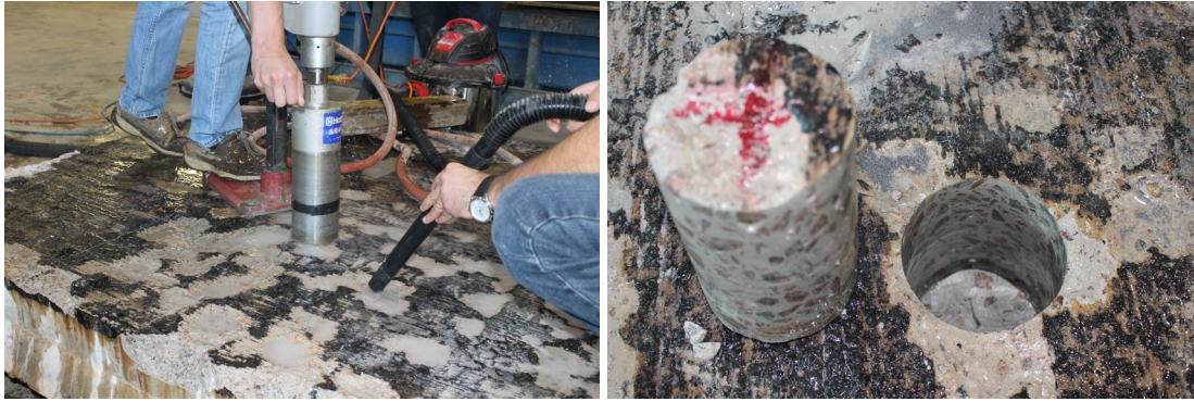
Figure 3.29: Extraction of cores
