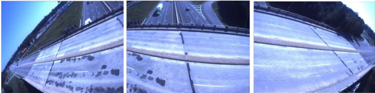
Figure 3.12: IR-UTD visual images at US-21, Wilson Blvd. over I-20 (ThermalStare, LLC., 2017) (figures reproduced with permission)
