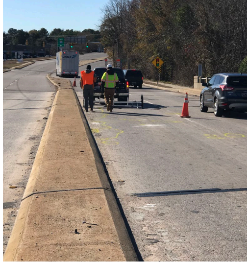
Figure 3.15: DAR ball-chain assembly in use on US-21, Wilson Blvd. over I-20
