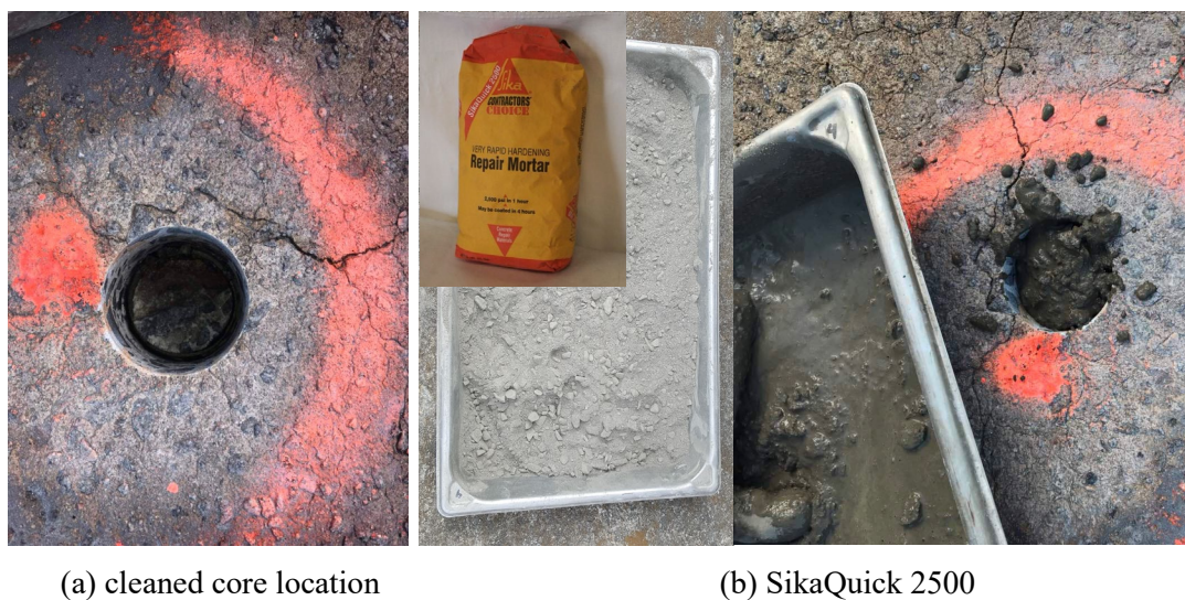
Figure 3.20: Repairing of core locations
