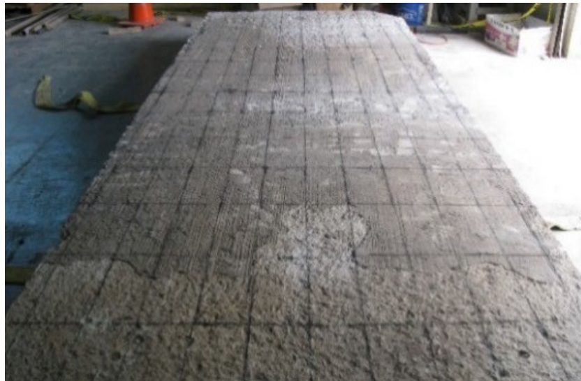
Figure 3.24: Marking positions of reinforcement
