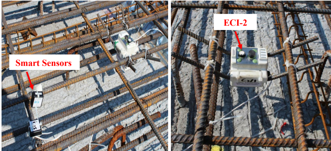
Figure 3.36: ECI-2 and smart sensors during installation and prior to casting
