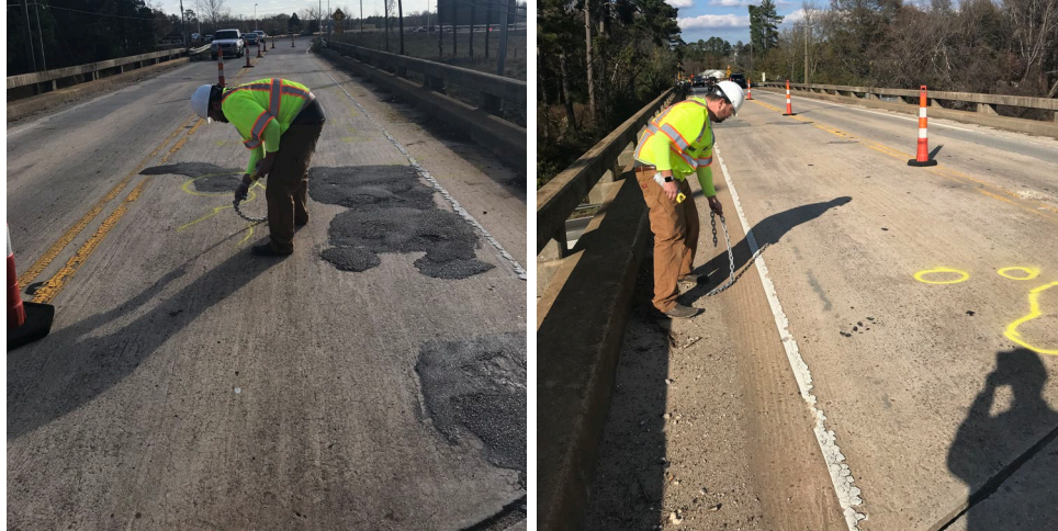
Figure 3.13: Chain dragging on S-106, Mineral Springs Road bridge over I-20
