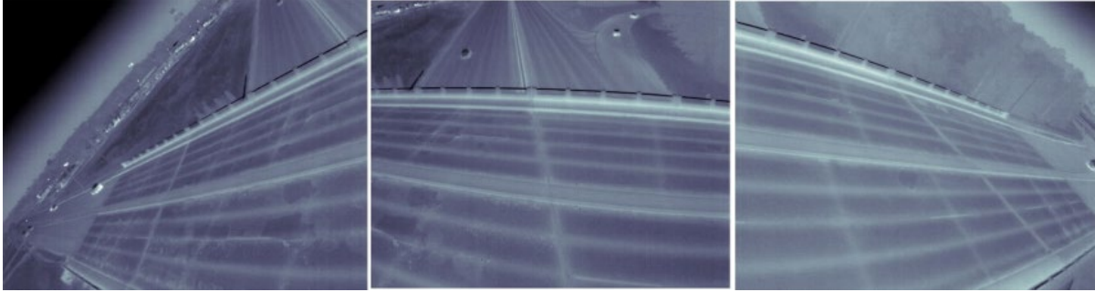
Figure 3.11: IR-UTD data showing structural features at US-21 Wilson Blvd. over I-20 (ThermalStare, LLC., 2017) (figures reproduced with permission)
