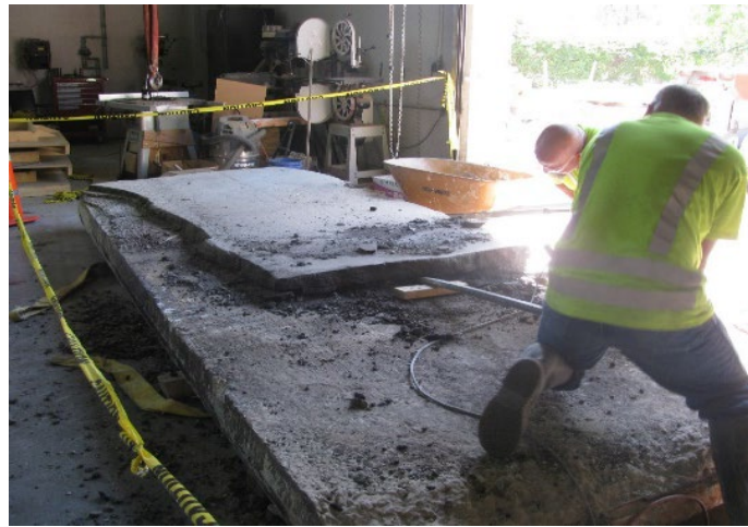
Figure 3.23: Removing the asphalt layer
