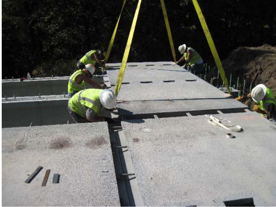
Figure 24. Photo. Close view of the deck panels.
