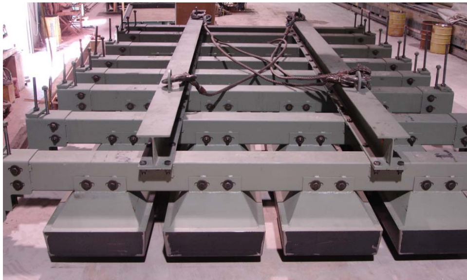
Figure 11. Photo. Void form.
