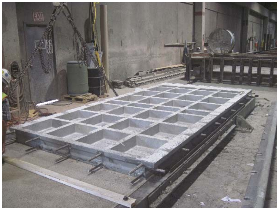
Figure 18. Photo. Formwork removed (panel upside down).
