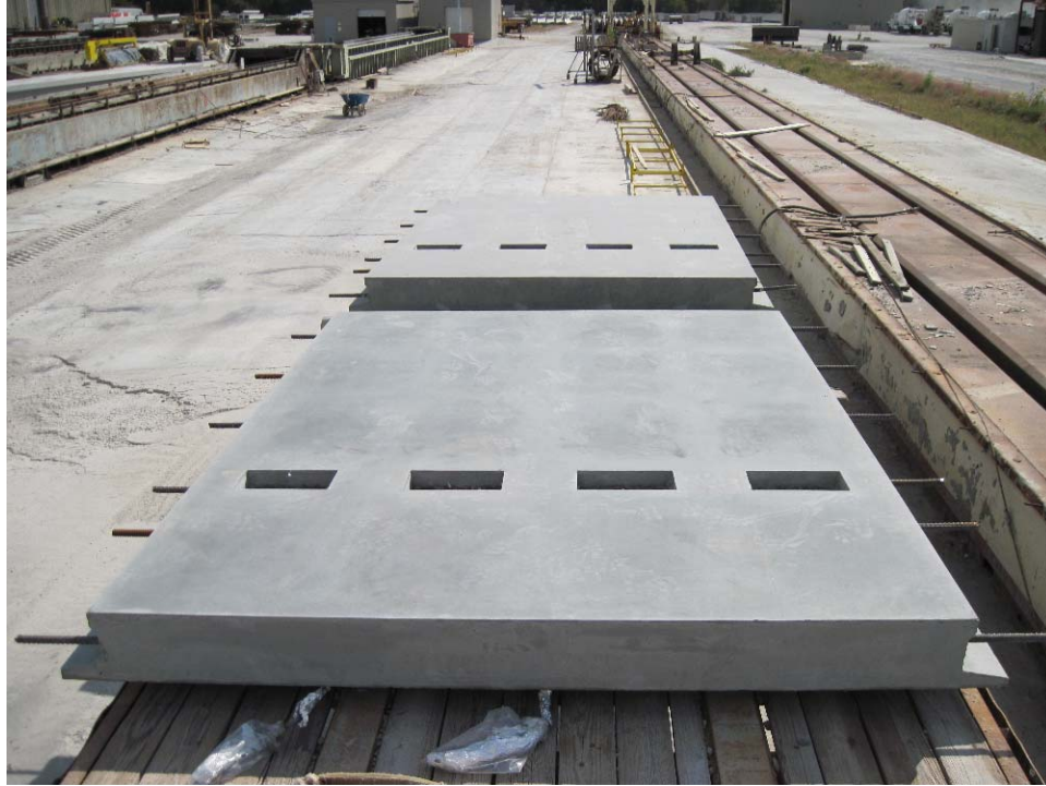
Figure 6. Photo. Completed prototype panels.
