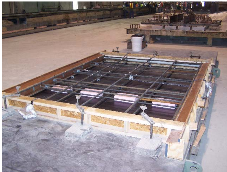
Figure 2. Photo. Prototype panel form setup.
