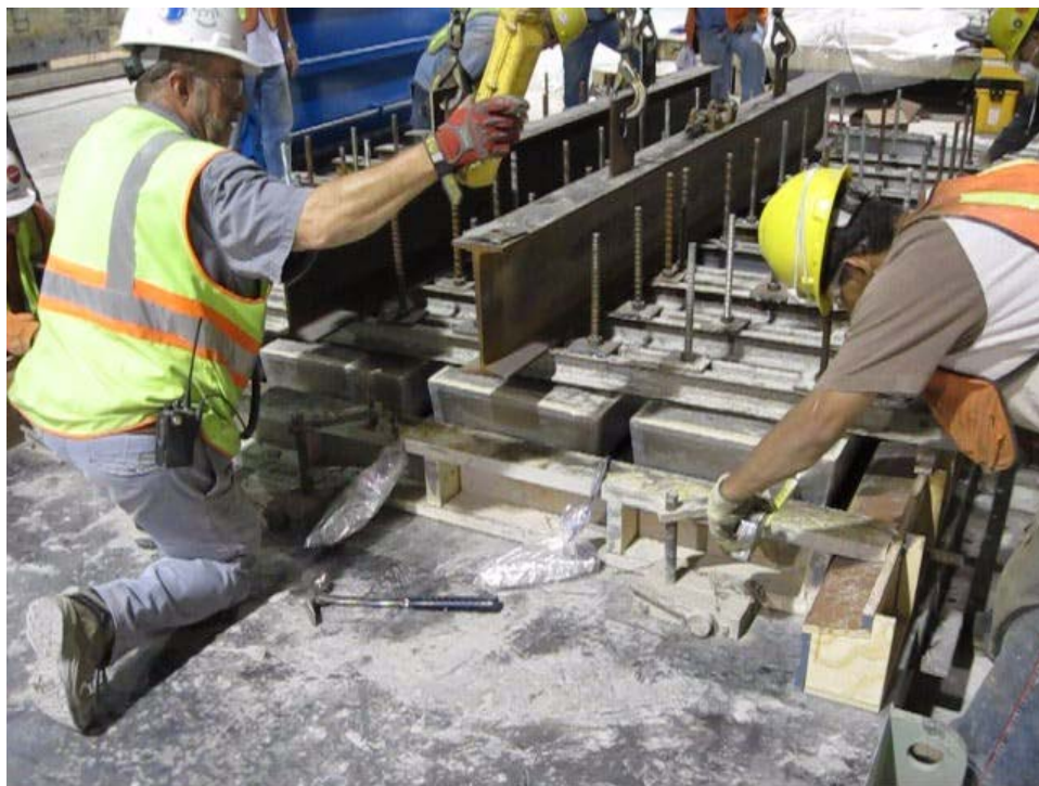
Figure 4. Photo. Placing the voids as they are lowered into position.
