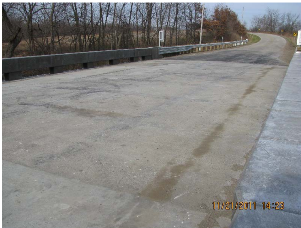
Figure 27. Photo. Completed demonstration bridge.
