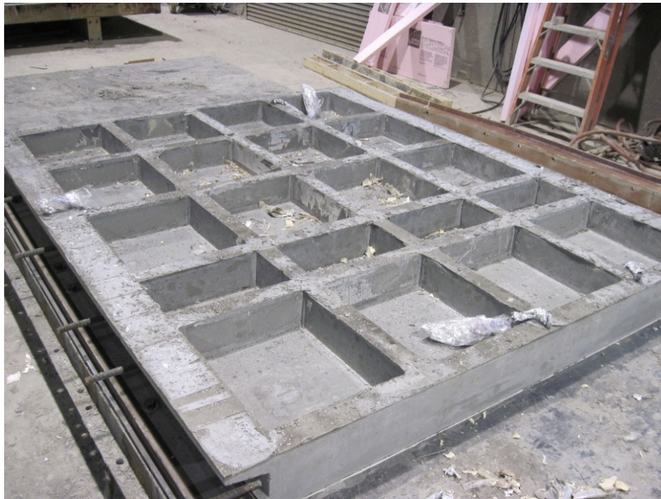
Figure 5. Photo. Formwork removed.
