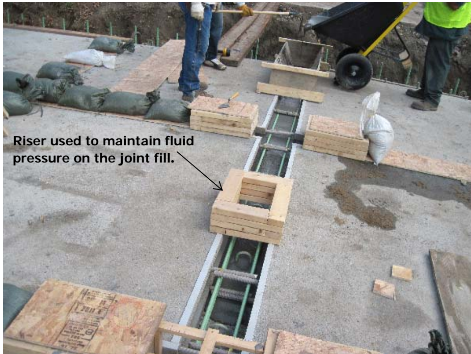
Figure 26. Photo. Transverse joint casting.
