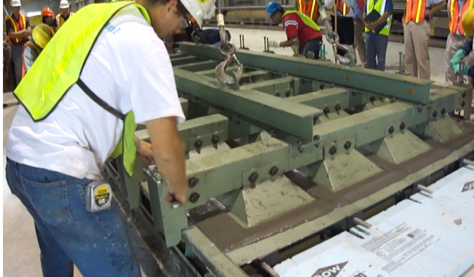
Figure 17. Photo. Placing the voids.
