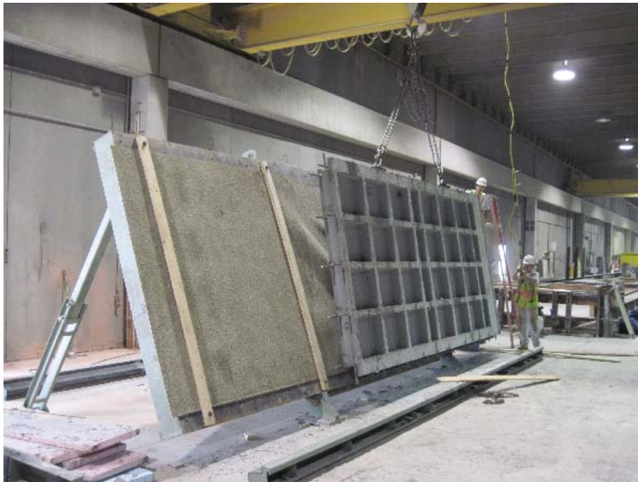
Figure 19. Photo. Lifting the panel to vertical.
