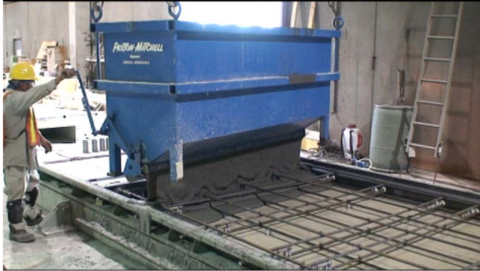
Figure 15. Photo. Placing UHPC.
