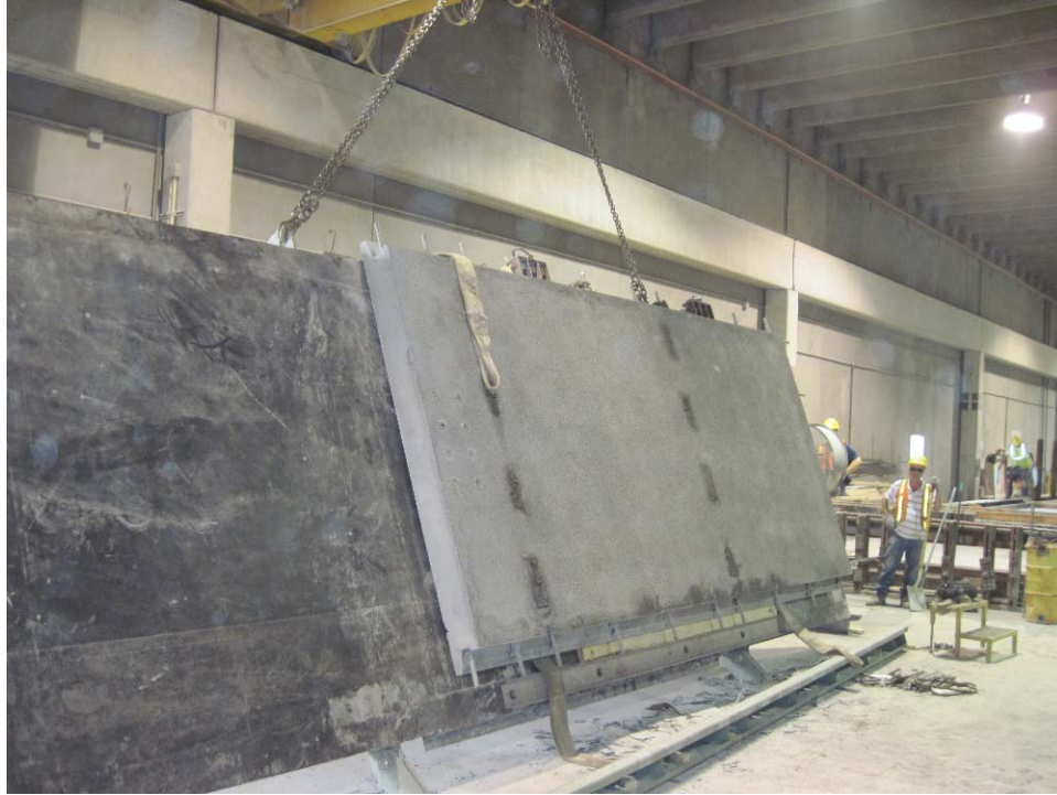
Figure 20. Photo. Panel rotated back to horizontal (panel right side up).
