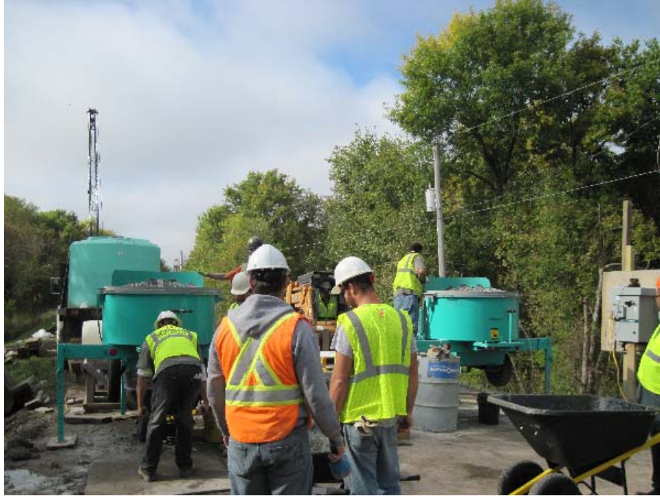
Figure 25. Photo. Portable mixers for batching joint fill UHPC.
