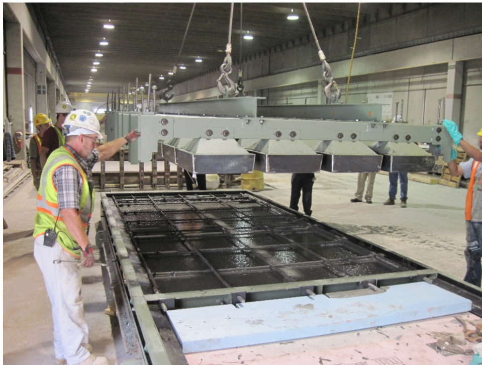
Figure 16. Photo. UHPC placed to correct level.
