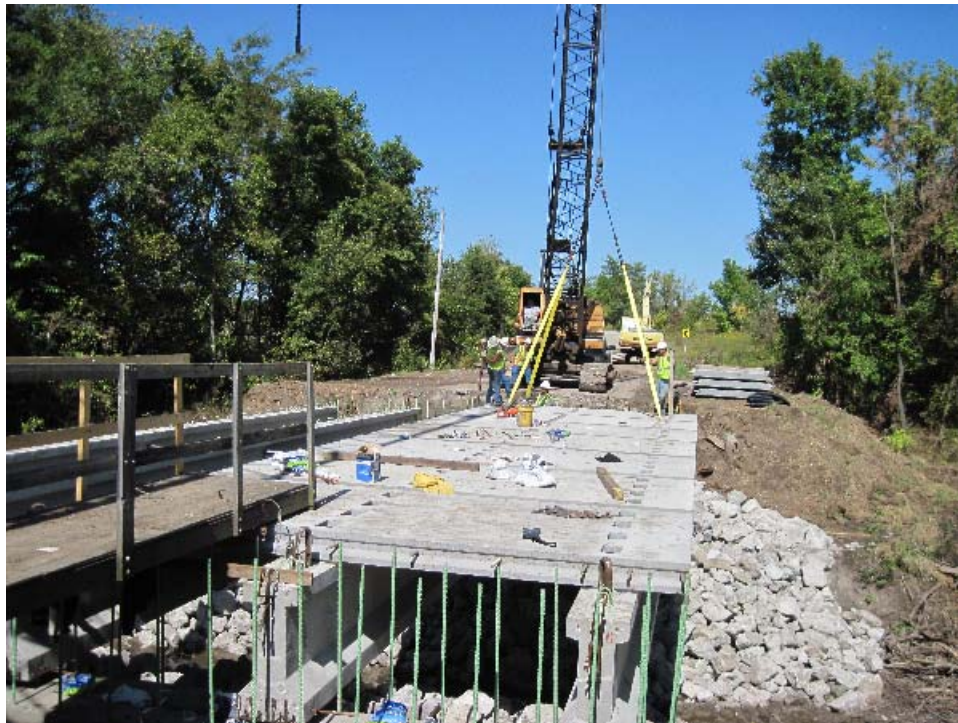
Figure 23. Photo. Setting the deck panels.
