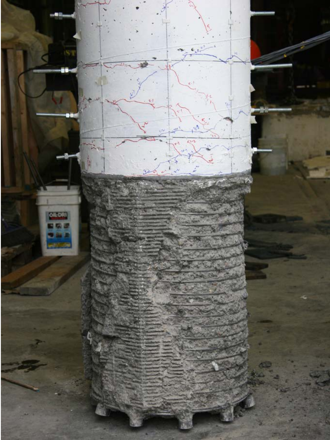
Figure 96. Photo. Specimen DS-2 column damage after cyclic testing.
