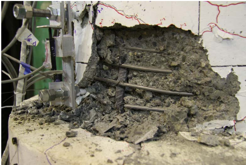
Figure 88. Photo. Specimen DS-1 – first column spiral fractured in cycle 10-1 (8.43/-8.27 percent drift).
