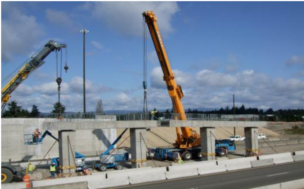
Figure 100. Photo. Precast cap beam placement.
