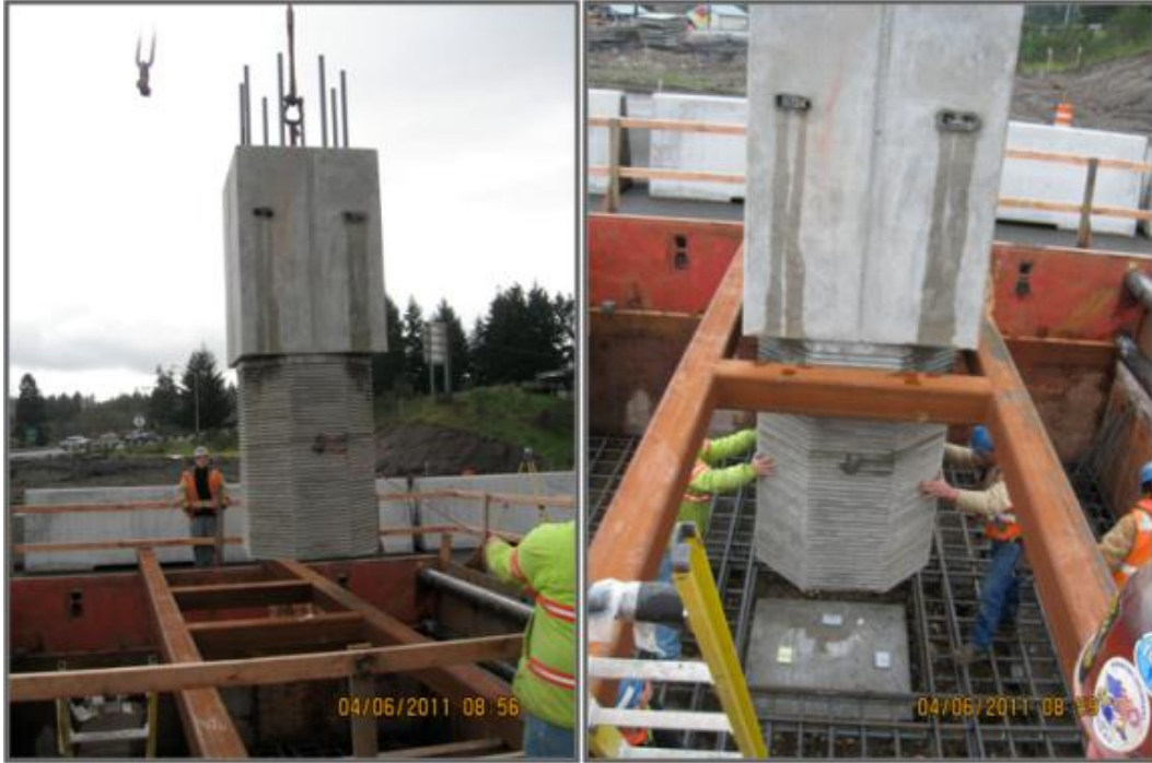
Figure 99. Photos. Construction sequence for placement of first precast column segment.
