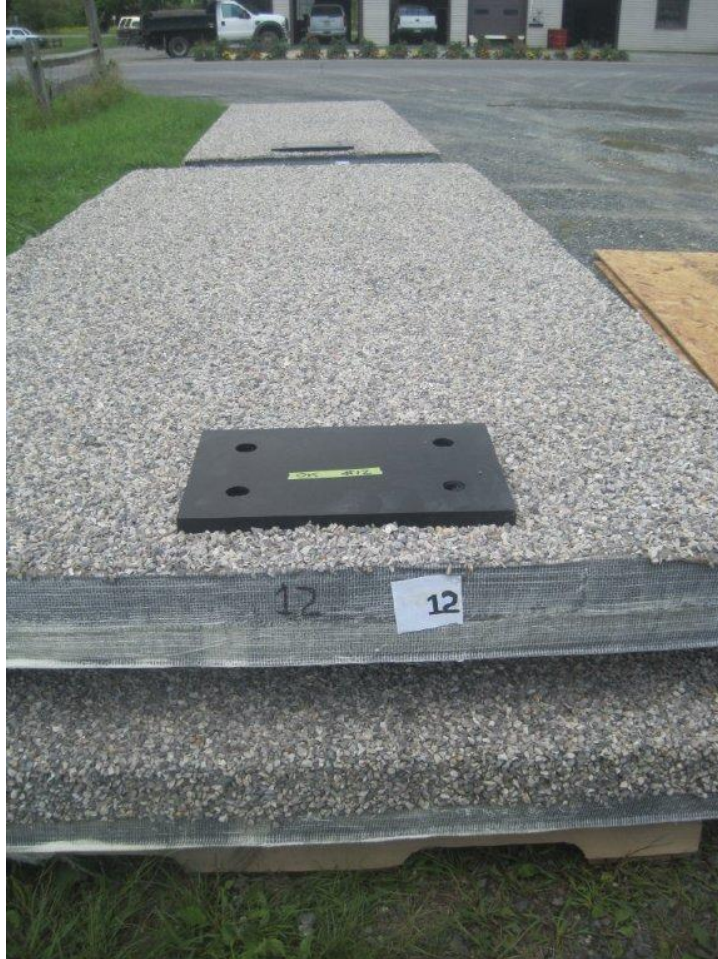
Figure 11. Photo. Panels labeled for shipping to the job site.
