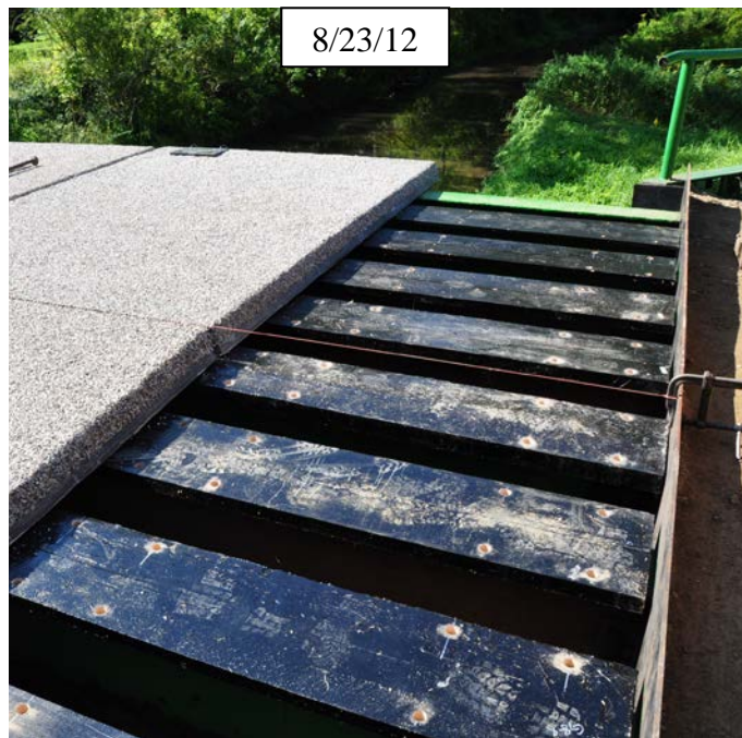
Figure 13. Photo. Place prefabricated haunches (black epoxy-coated red oak).
