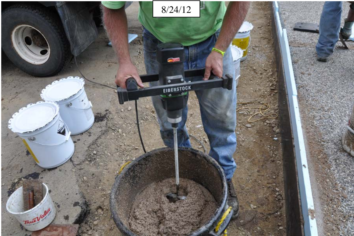
Figure 24. Photo. Mix epoxy grout for deck nosing at bridge joints.
