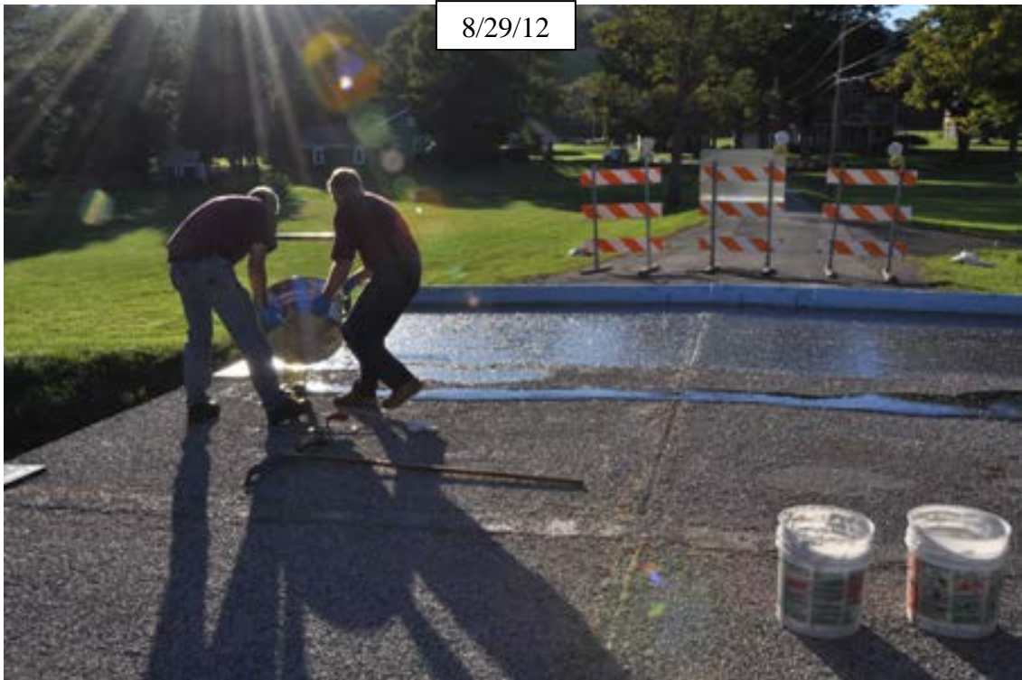
Figure 26. Photo. Apply resin for second course of wearing surface.
