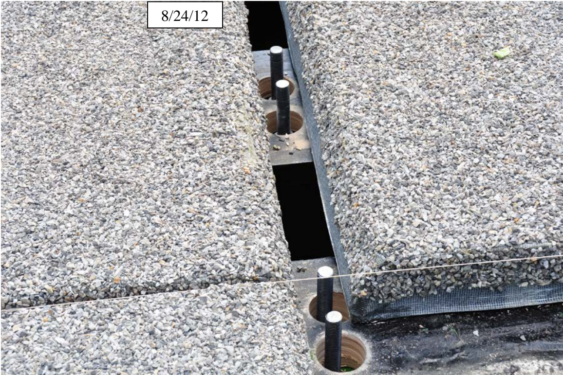
Figure 20. Photo. Install fixed connection between deck and steel stringers per plan.
