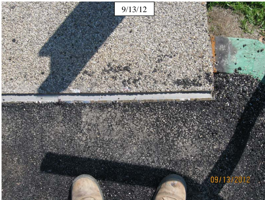
Figure 29. Photo. Install two-part pourable joint material per manufacturer's instructions.
