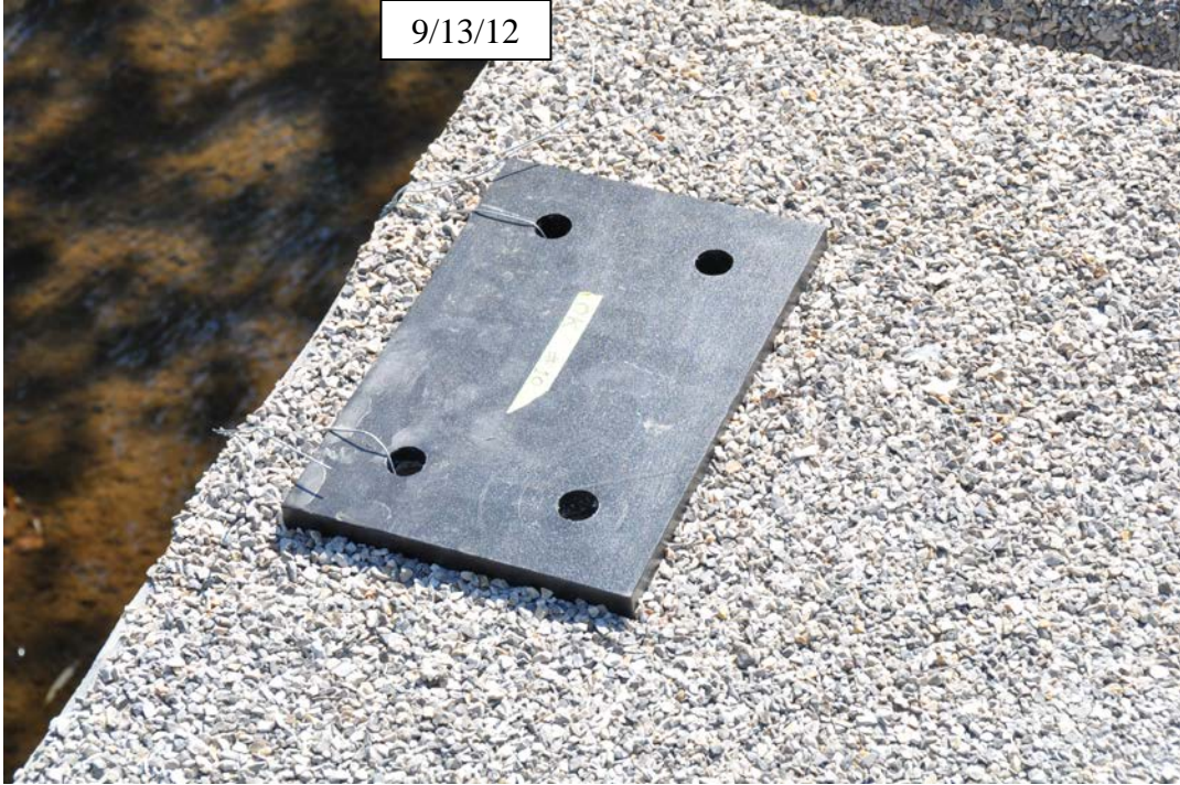
Figure 30. Photo. Align prefabricated high-density polyethylene pad for bridge railing posts.
