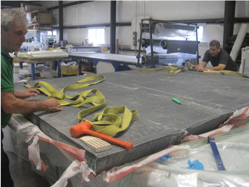
Figure 9. Photo. Infused deck panel is stripped and inspected for thorough wet-out.
