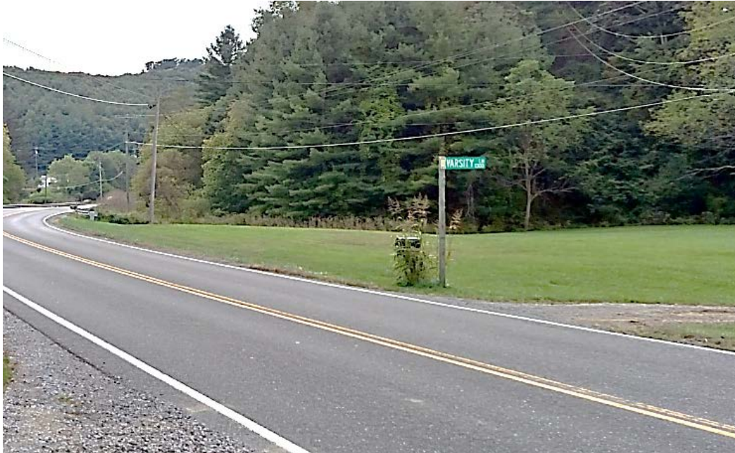
Figure 2. Test Site at Riner Rd. and Varsity Ln. (Driveway) Selected for Cable Installation.
