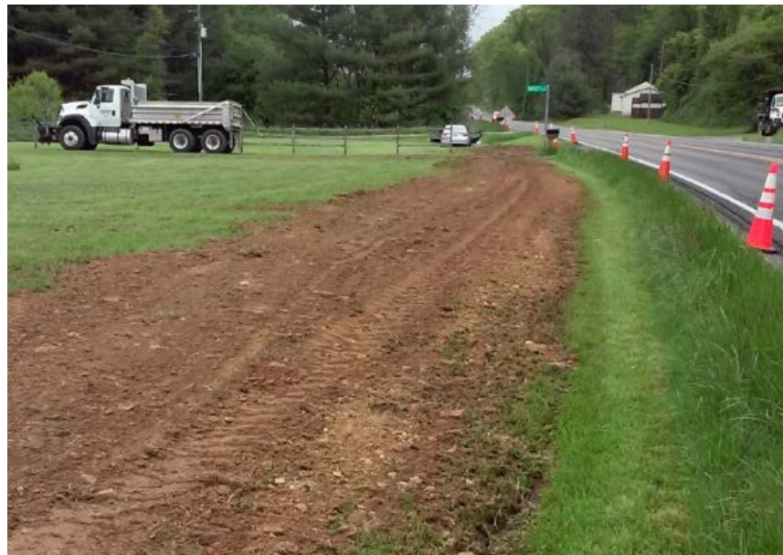
Figure 6. Trench Covered with Compacted Native Soil.
