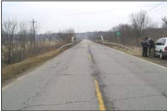
Buck Creek bridge (planned improvements include repaving, bridge improvements, and 8' paved shoulders)
