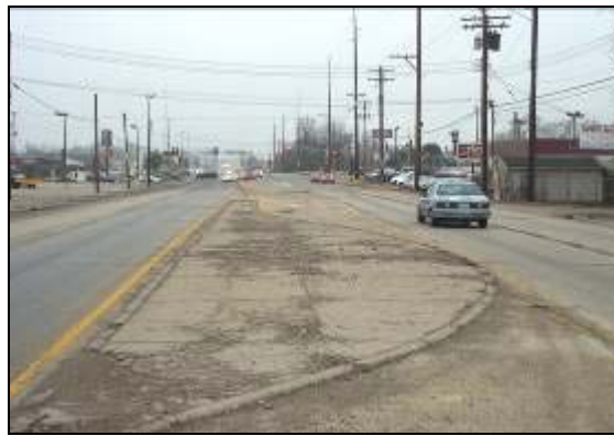
Dirksen Parkway (looking south toward intersection with Clear Lake Avenue)
