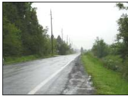
172 nd Avenue near Ward Road
