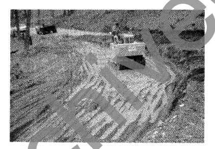
Figure 21. Highway embankment with fly ash structural fill.
