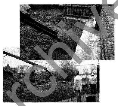
Figure 17. Bridge abutment backfill with flowable fill.
