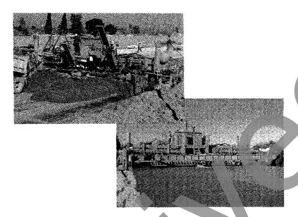
Figure 5. The addition of fly ash to concrete enhances workability even in very stiff mixes.
