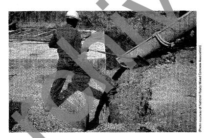
Figure 15. Flowable fill eliminates the need for workers to enter the trench to compact.
