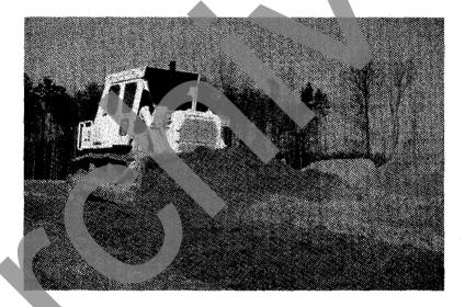
Figure 22. Spreading fly ash structural fill.
