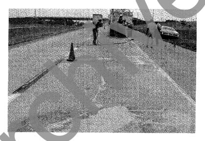
Figure 19. Fly ash grouts for pavement subsealing.
