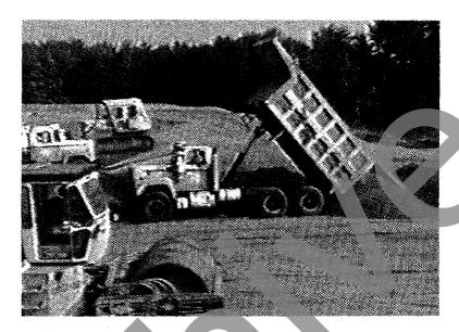
Figure 23. Compaction of fly ash structural fill is crucial, as with any backfill material.
