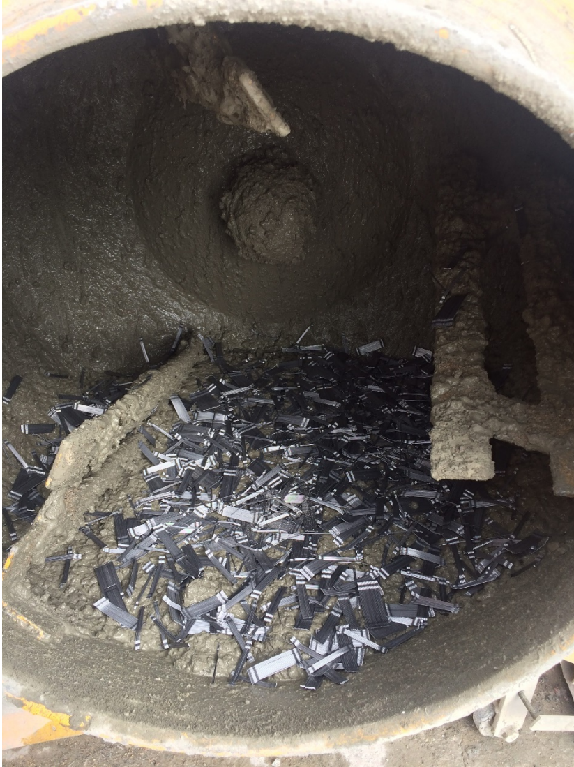
Figure 3.2 Distribution of fibers on the surface of the resting concrete, prior to the final five minutes of mixing
