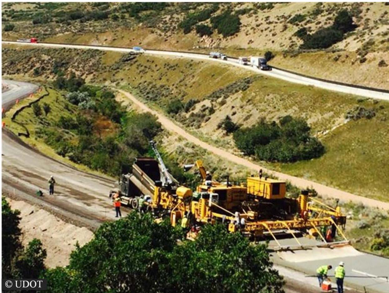
Figure 41: Photo. String line paving for the eastbound in 2014.
