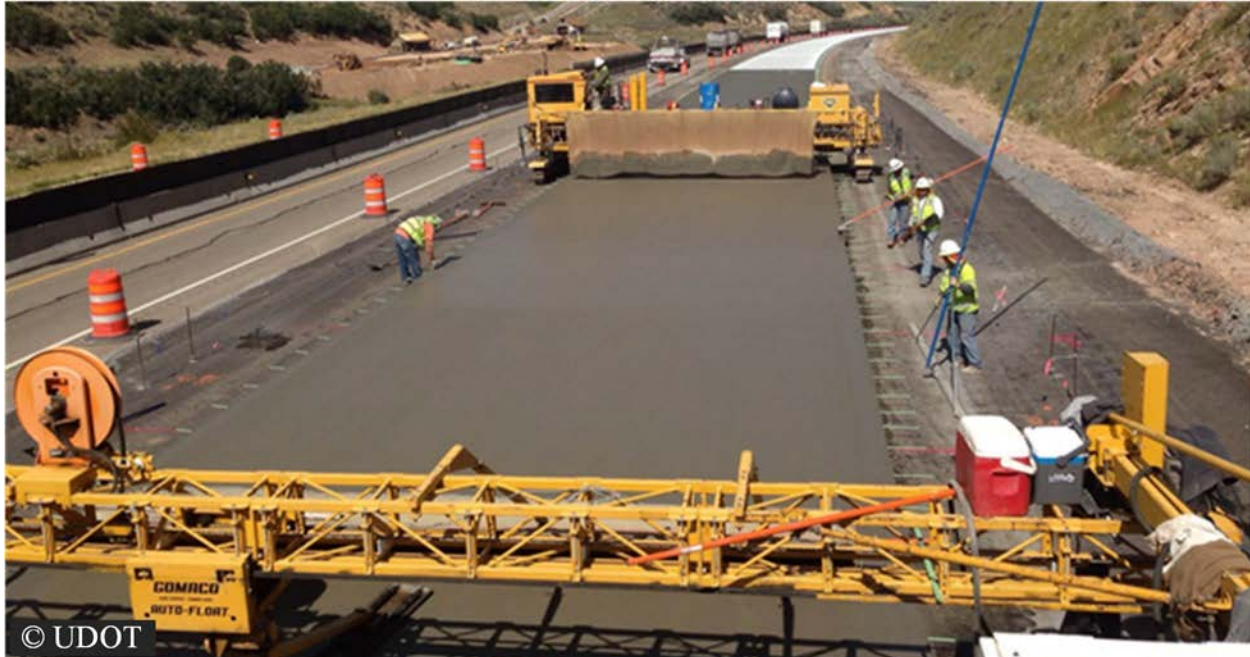
Figure 43: Photo. Hubs were set every 30 feet for string lines.
