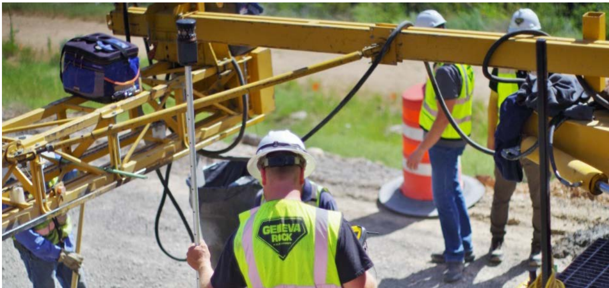
Figure 49: Photo. The contractor's surveyor checks grade behind the paver.
