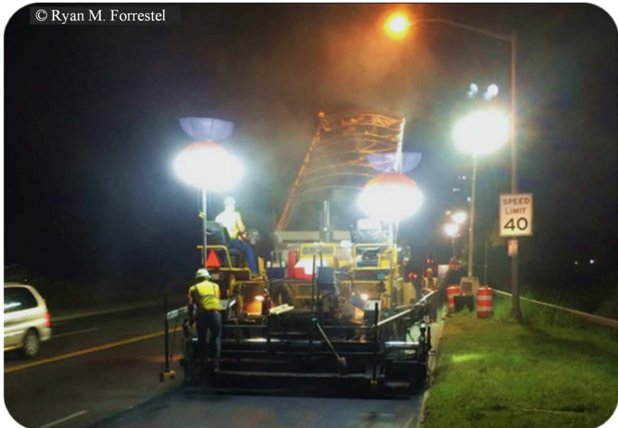
Figure 70: Photo. Asphalt overlay with sonic skis.
