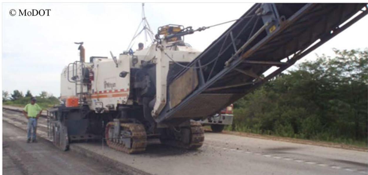
Figure 57: Photo. All asphalt was milled before survey could be collected. (19)
