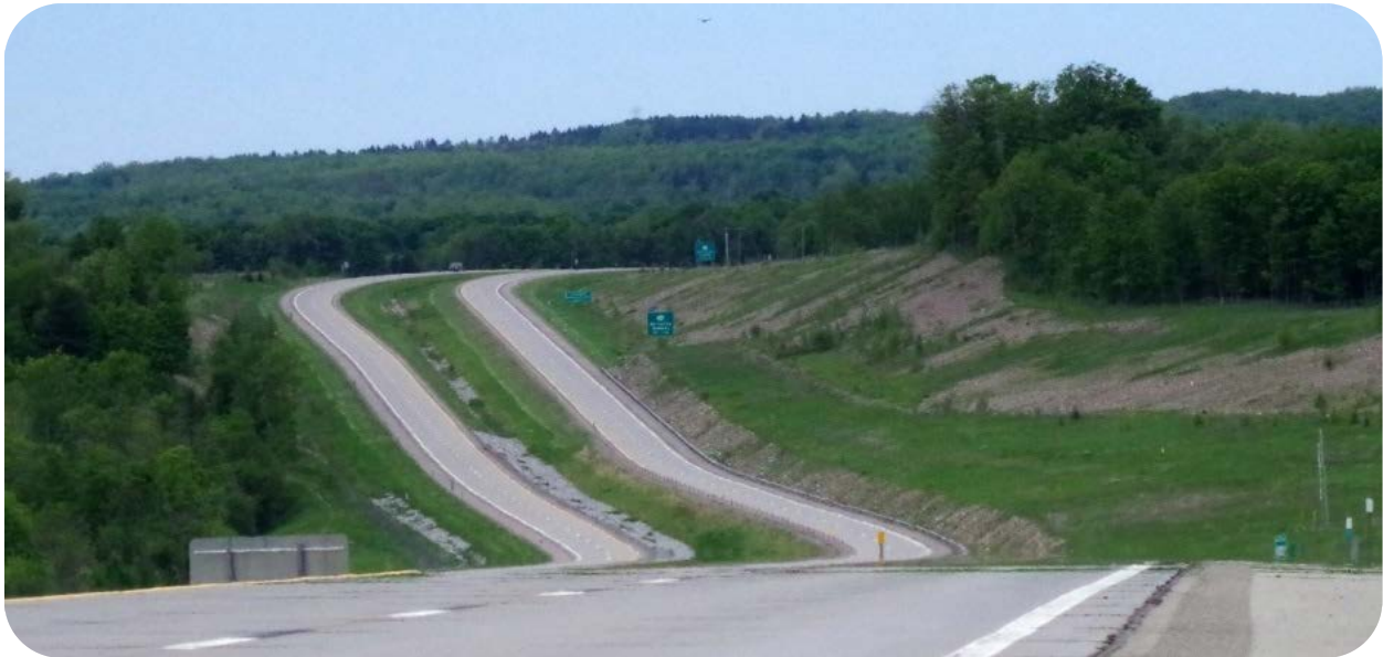
Figure 13: Photo. Looking north through the landslide area.
