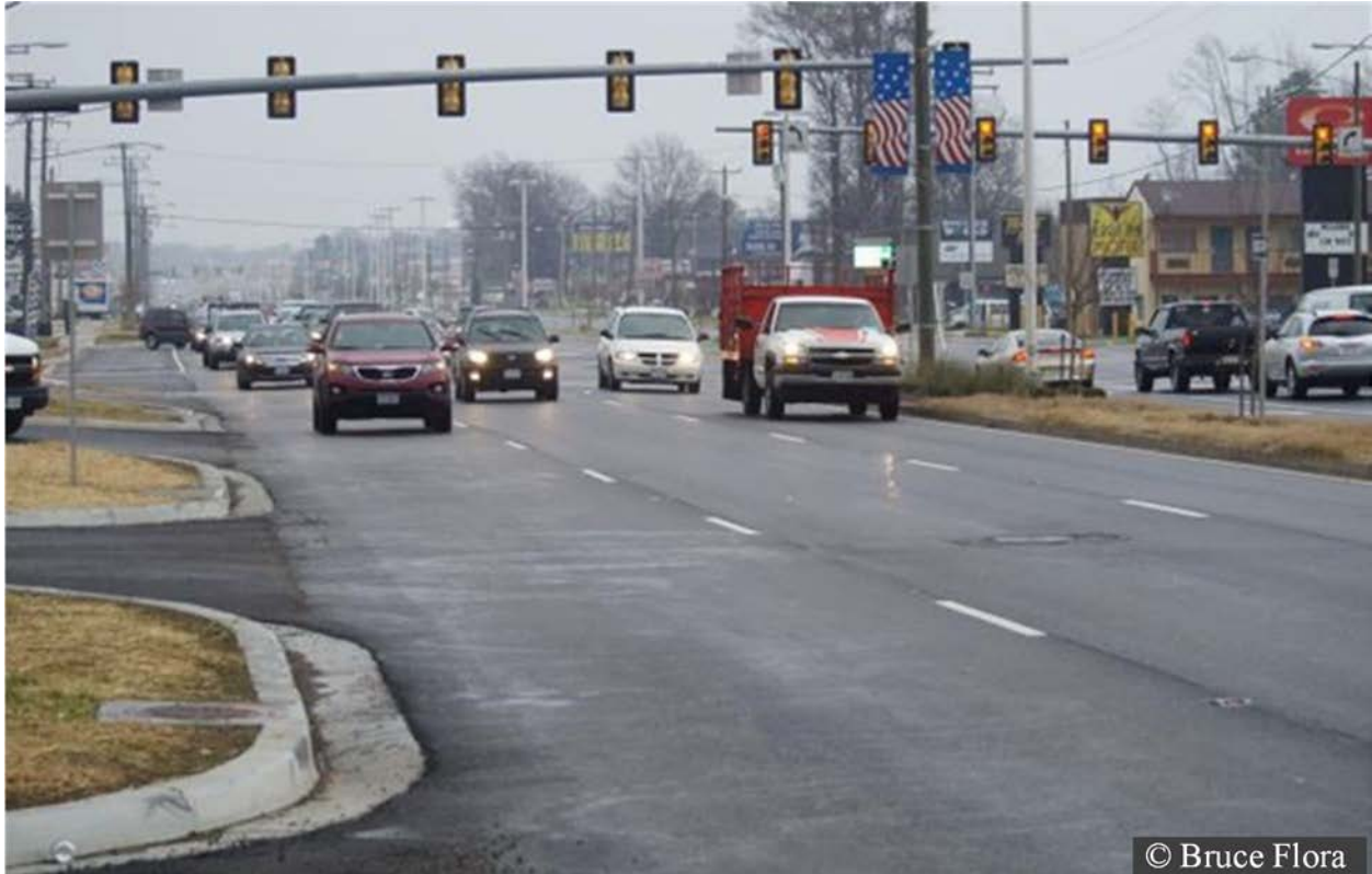
Figure 37: Photo. Route 60 after final paving.
