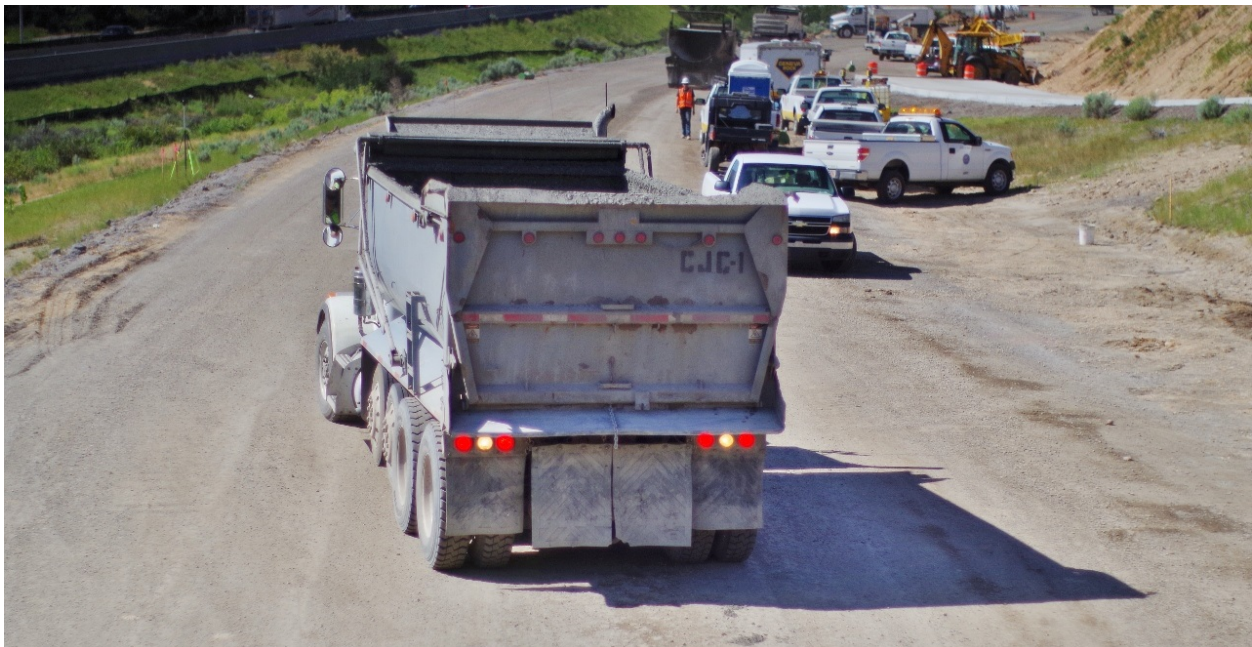
Figure 51: Photo. Stringless paving provides better access to the work area.
