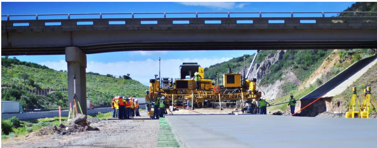
Figure 47: Photo. AMG operations need staggered, accurate control.
