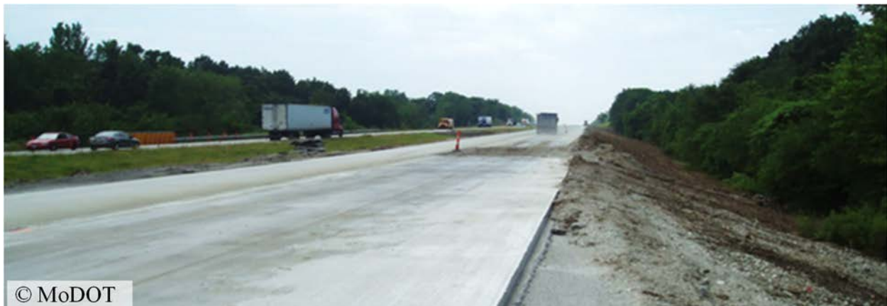
Figure 55: Photo. Construction used full closure and head-to-head traffic. (19)
