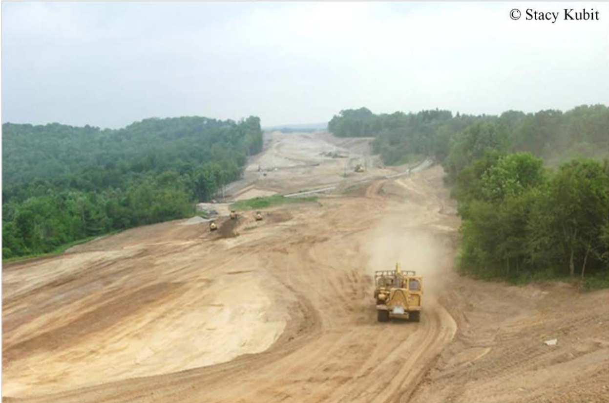
Figure 18: Photo. The original ground was covered by heavy woods.
