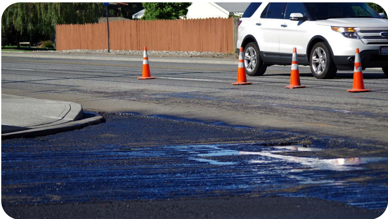
Figure 113: Photo. Urban milling and asphalt paving.
