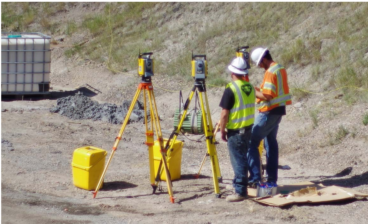
Figure 50: Photo. Three RTSs are necessary at each AMG paving setup.
