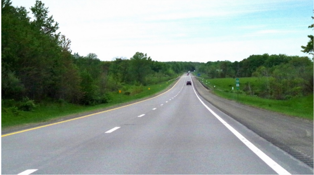
Figure 71: Photo. Good smoothness outcomes were achieved.
