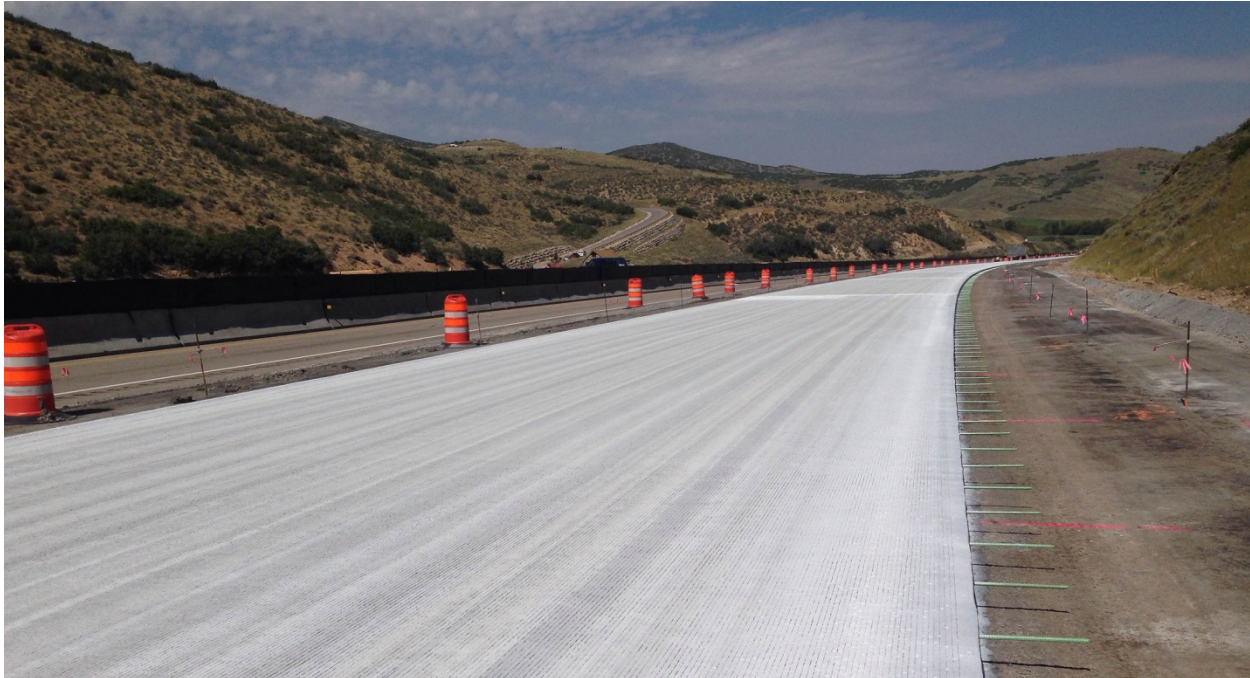
Figure 52: Photo. String line and stringless paving had good smoothness.
