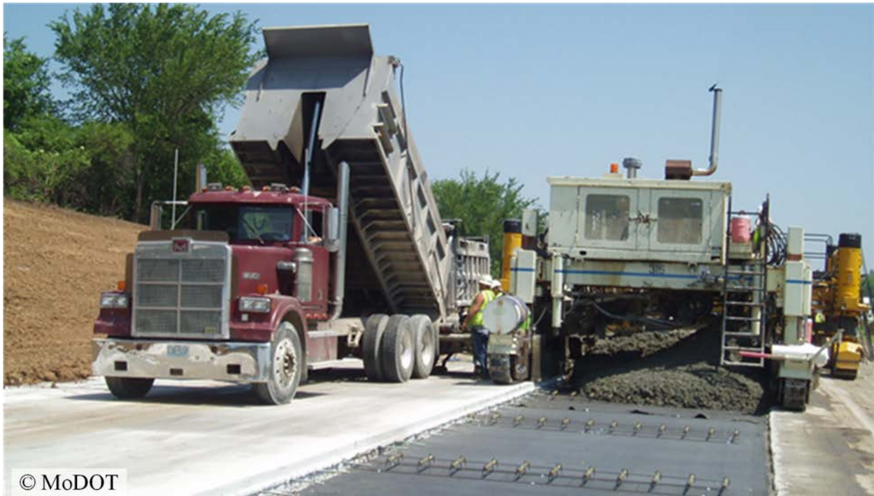
Figure 60: Photo. Dowel bar cages were placed ahead of the paver.
