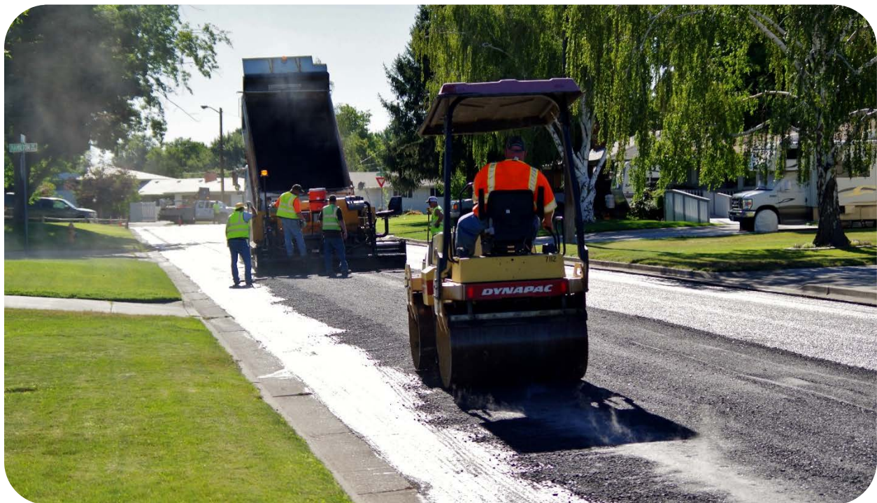
Figure 110: Photo. Asphalt paving operation for an urban mill and overlay.
