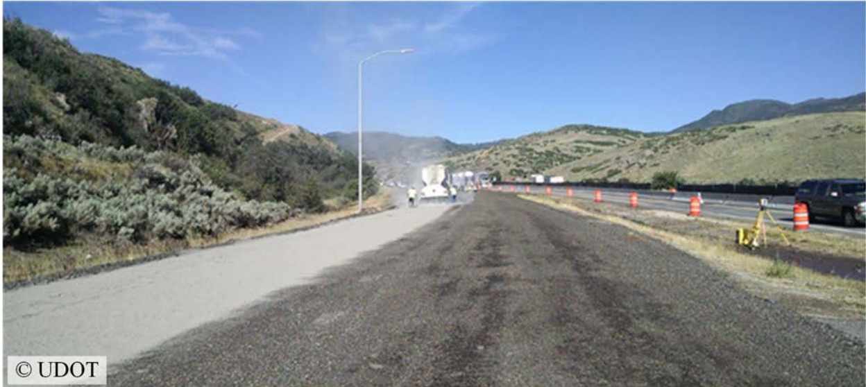
Figure 39: Photo. All CTAB operations used RTS control.
