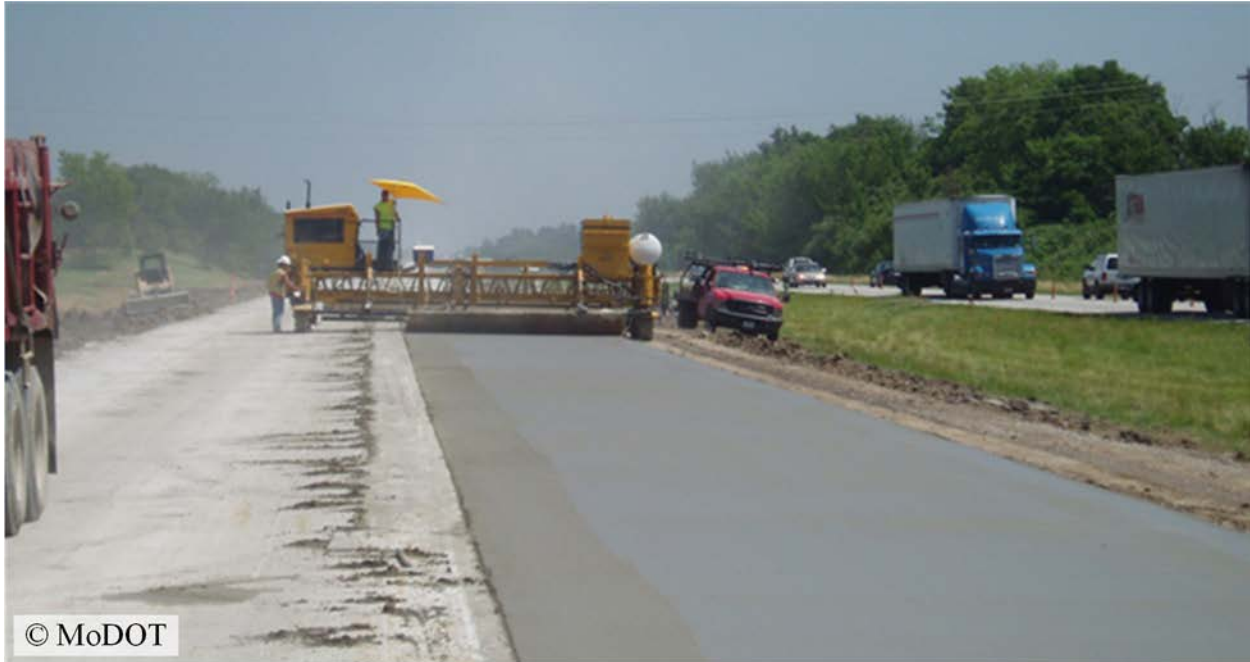
Figure 62: Photo. The work zone was close to live traffic.
