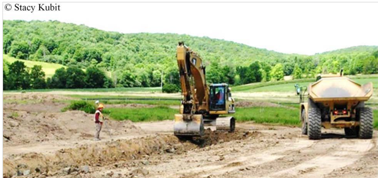
Figure 23: Photo. An inspector waits safely during excavation.
