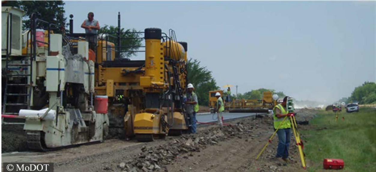
Figure 58: Photo. Concrete pavers use resection for positioning.
