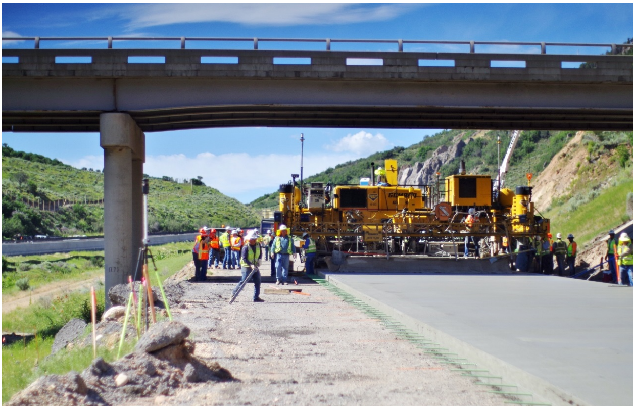
Figure 40: Photo. Tight clearances under the Tollgate Bridge.
