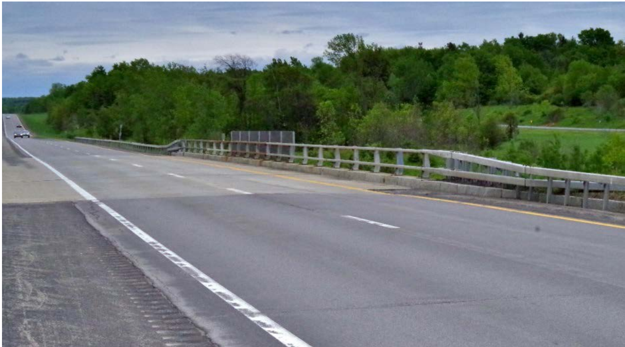
Figure 68: Photo. A bridge on US 219 looking south.
