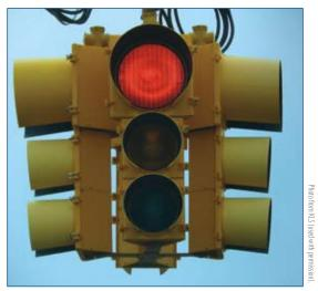
Figure 1: Relative size difference between 12-inch (top lens) and 8-inch signal lens (bottom lenses)
