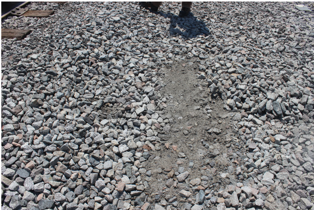
Figure B-15: Mud pumping in adjacent ballast, Signal #2
