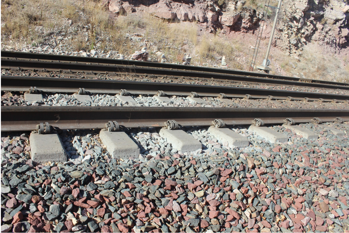
Figure D-17: Ballast churn seen on-site
