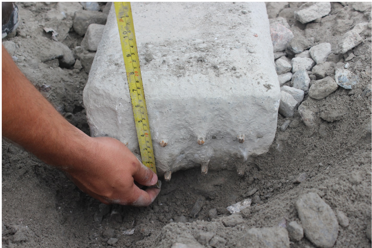
Figure C-17: One-inch abrasion on bottom of the tie. Crossing #3
