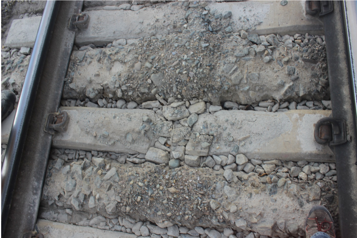
Figure E-35: Shattered tie, Tangent #7
