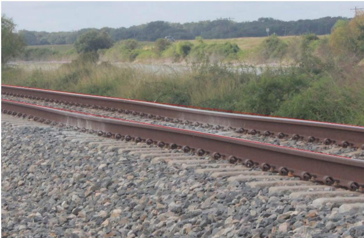
Figure 3-17: Rail surface profile variation for track built on an old concrete highway. Red lines show the more than 1.3 in. of surface profile variation measured by the ATIP geometry car approximately 2 years before the picture was taken
