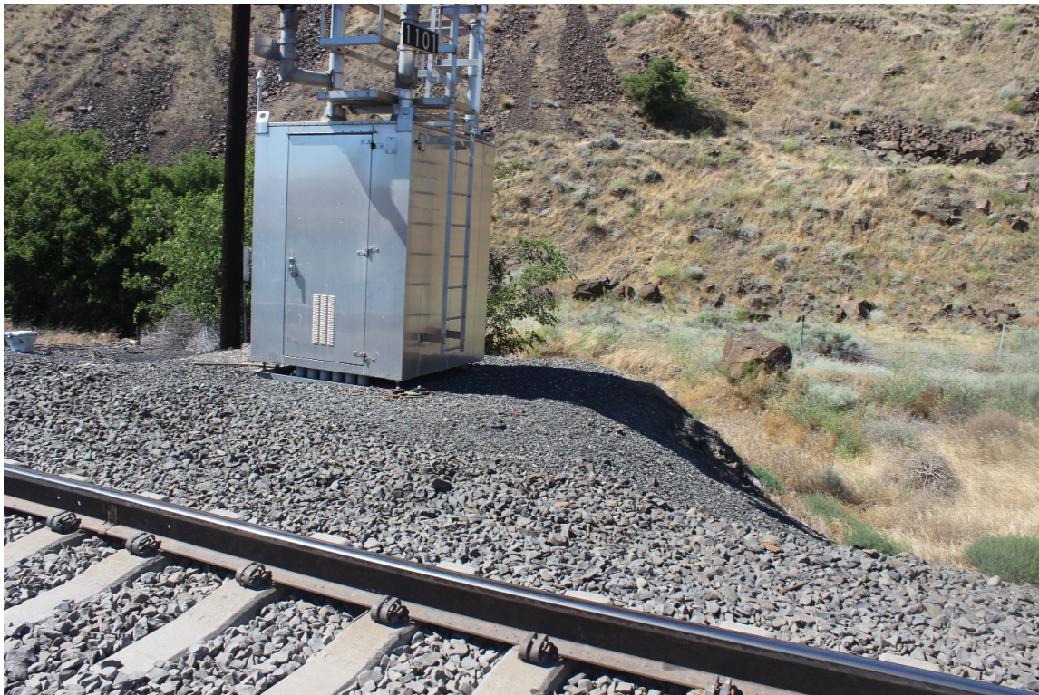
Figure E-9: Poor grading at signal, Tangent #2
