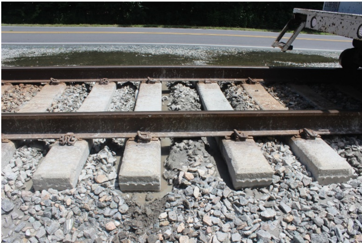
Figure 3-5: Water ponding in track, contributing to mud pumping
