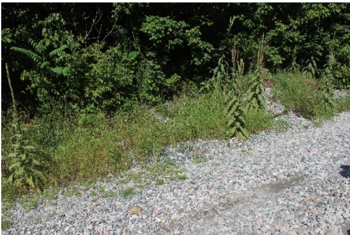
Figure E-57: Fines and vegetation adjacent to track, Tangent #11
