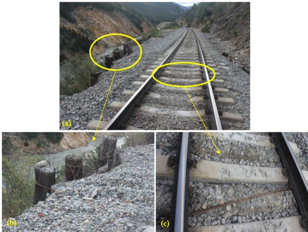
Figure E-36: Wooden piles with tie-back cables to stabilize the track, Tangent #7
