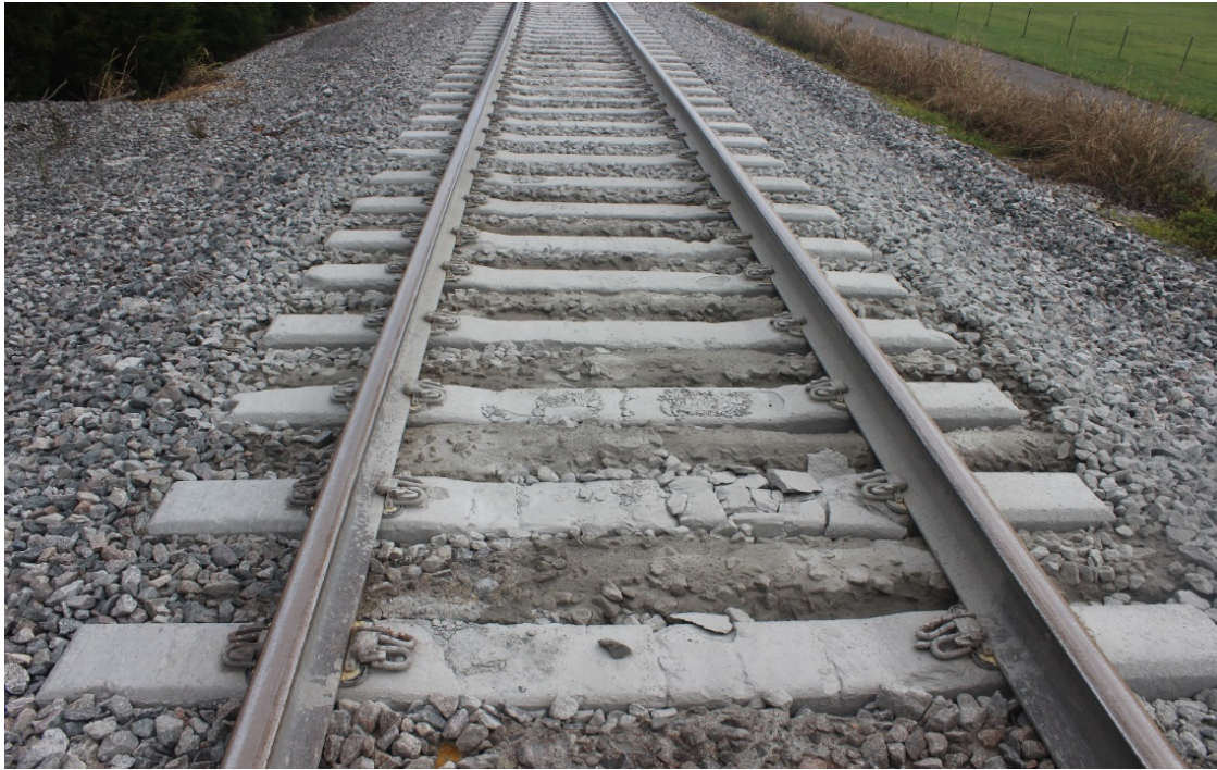
Figure 3-23: Shattered ties at mud pumping location
