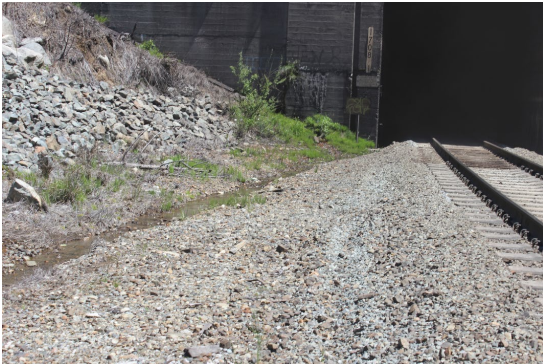
Figure 3-2: Water emanating from tunnel portal
