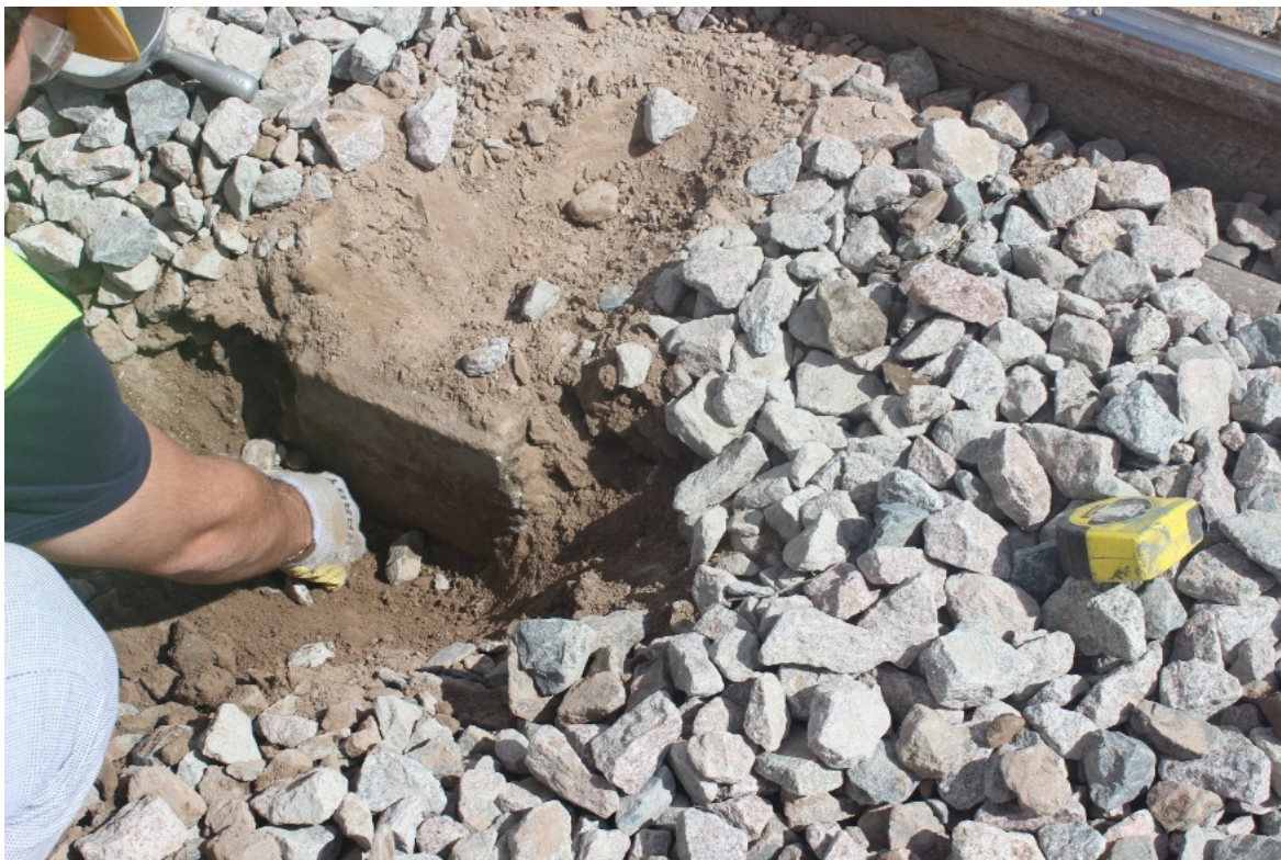
Figure E-16: Pumping due to the insufficient ballast layer thickness, Tangent #4
