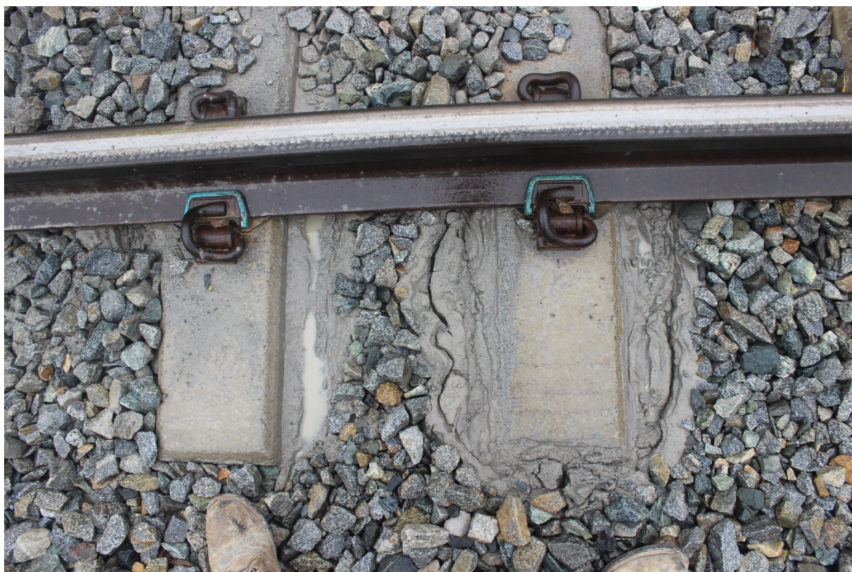
Figure E-42: Pumping produces fine particles around the tie, Tangent #8
