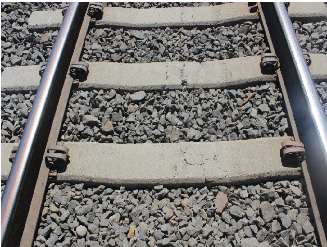
Figure 3-24: Ties with center-binding cracks in an area with good drainage, maintenance, and support conditions and very low measured bottom wear
