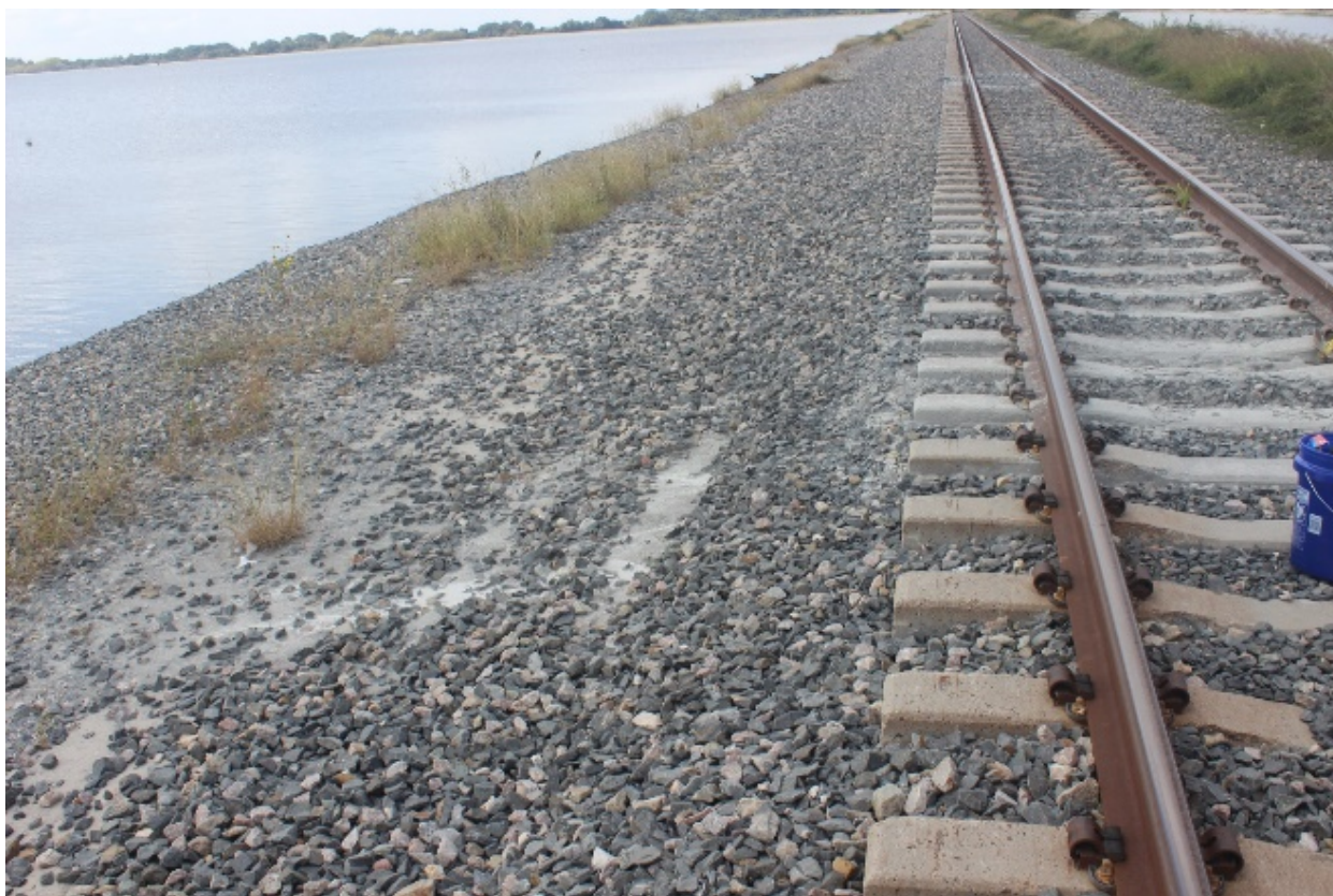
Figure A-24: Fines on the side of track, Bridge Approach #2
