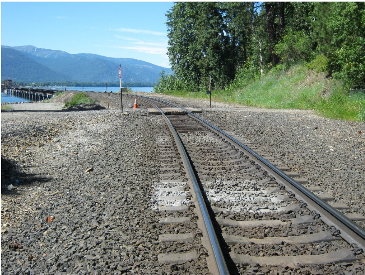
Figure C-3: Pumping area near curve, Crossing #1
