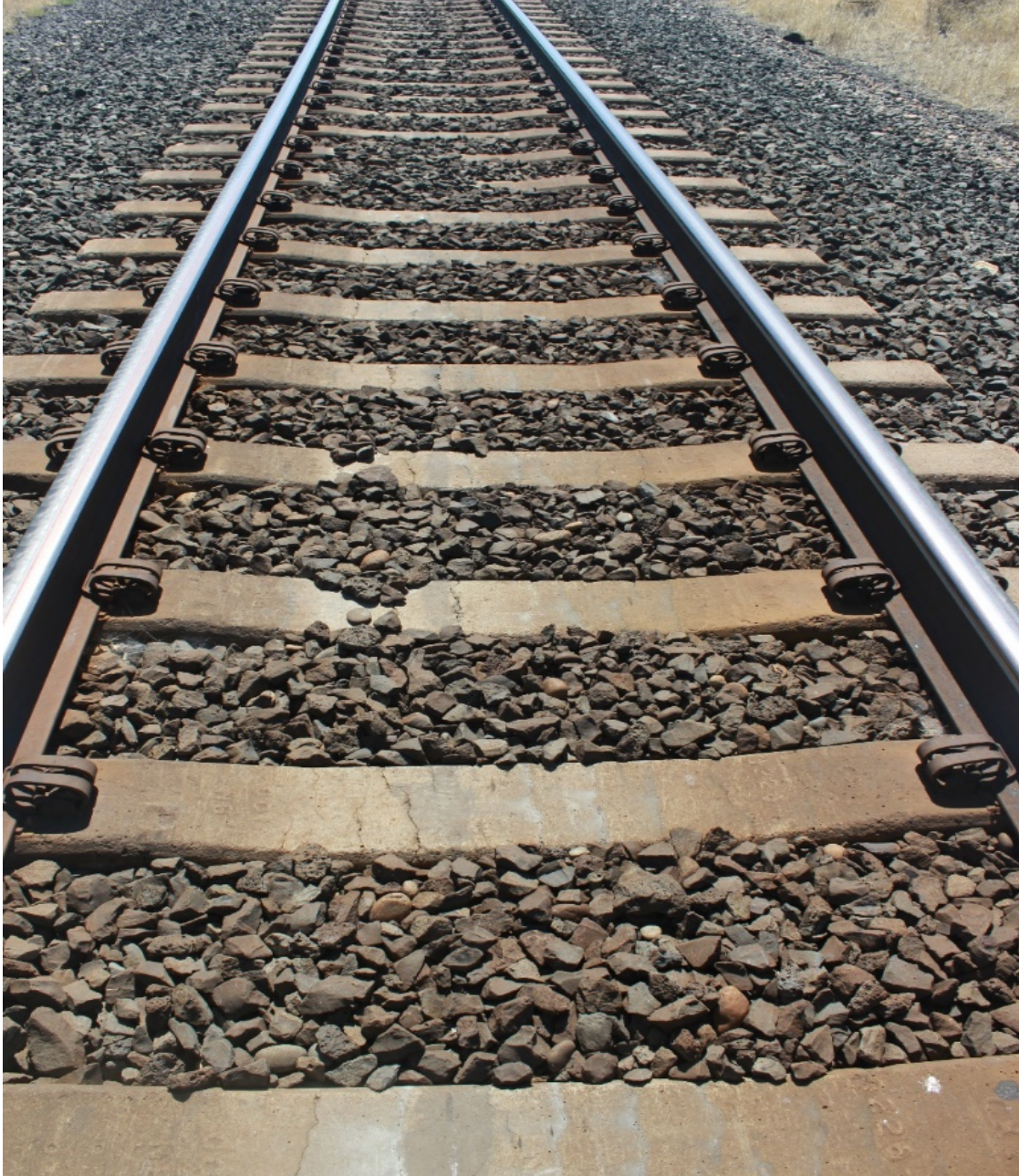
Figure D-16: Center-binding cracking, Curve #3
