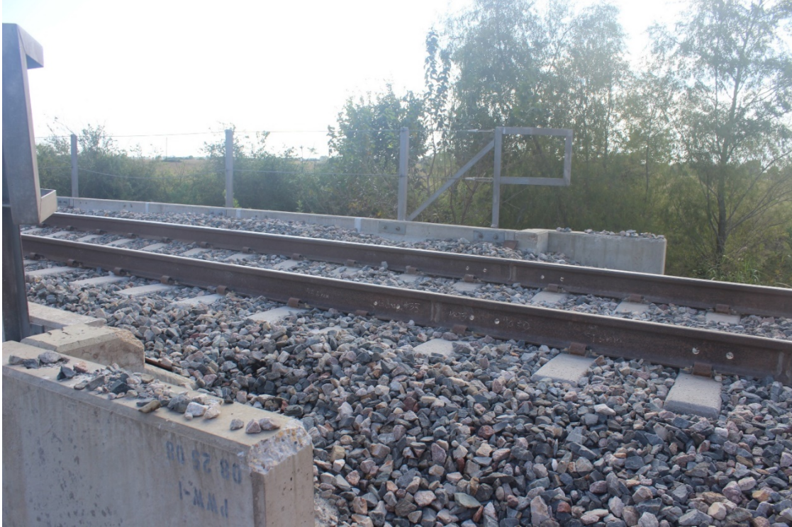
Figure A-8: Bridge #2 abutment where ballast was replaced 8 months prior to the site visit by the research team
