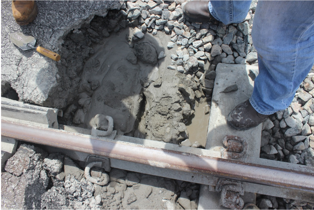
Figure 3-6: Mud spot at an asphalt crossing
