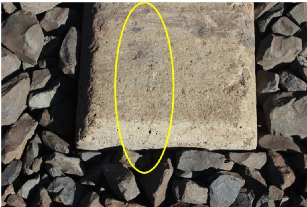
Figure D-10: Vertical splitting crack, Curve #2
