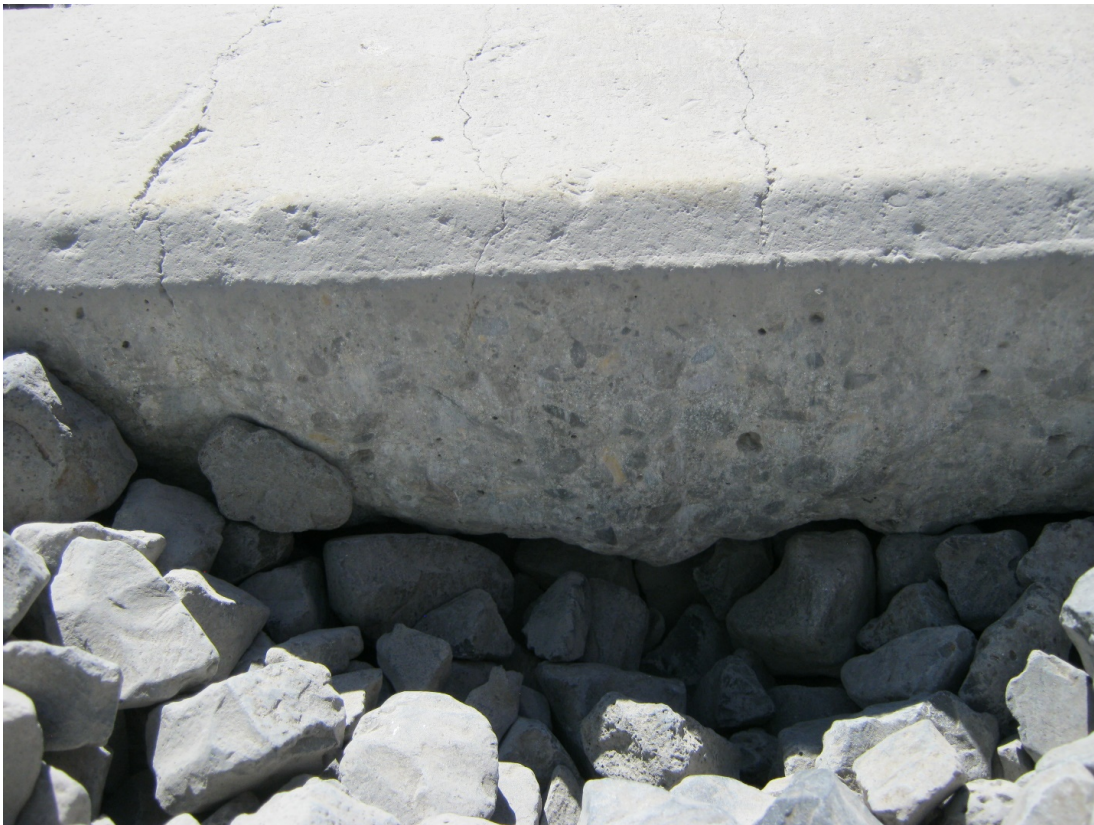
Figure E-7: Center binding cracking and tie rounding, Tangent #2
