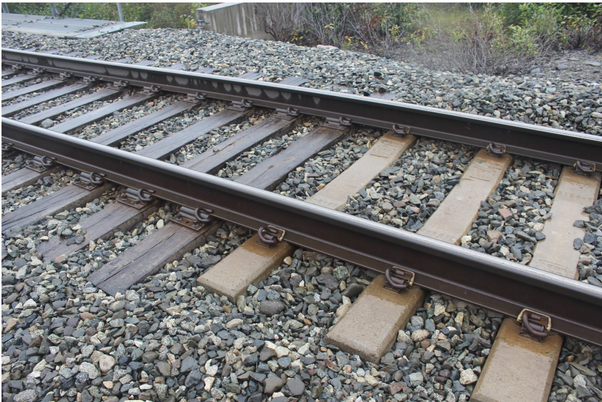
Figure A-27: Transition zone from concrete to wood ties, Bridge Approach #3
