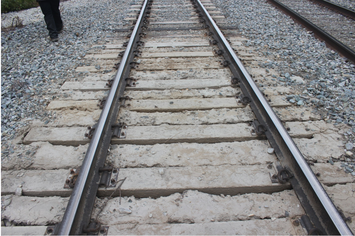
Figure E-46: Mud pumping, Tangent #9
