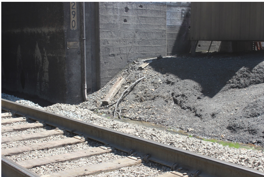
Figure A-36: Water from tunnel in ditch, tunnel approach
