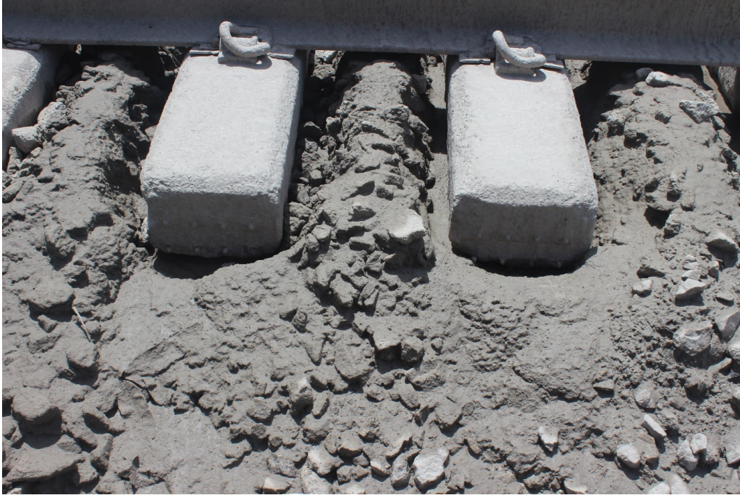
Figure B-24: Mud pumping, Signal #3
