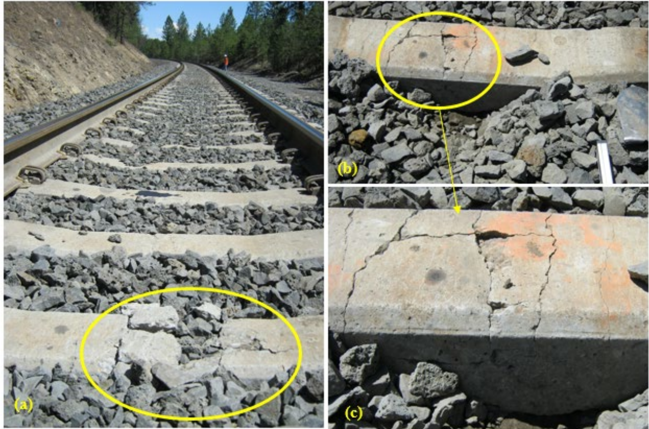
Figure D-3: Severe center binding cracking, Curve #1
