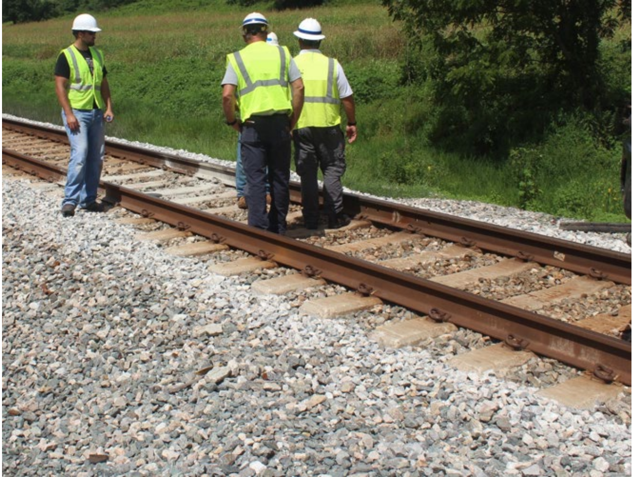
Figure C-37: Ballast fouling seen in track on four ties, Crossing #6
