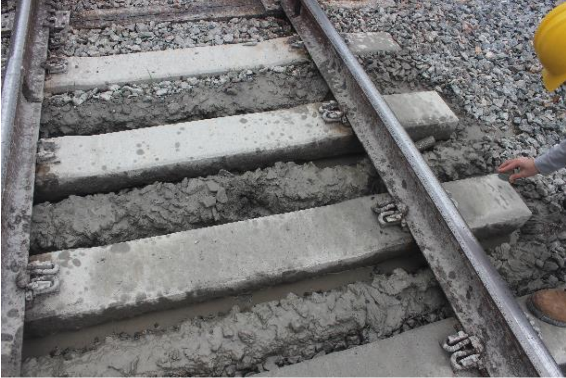
Figure C-29: Mud Pumping at Crossing#5
