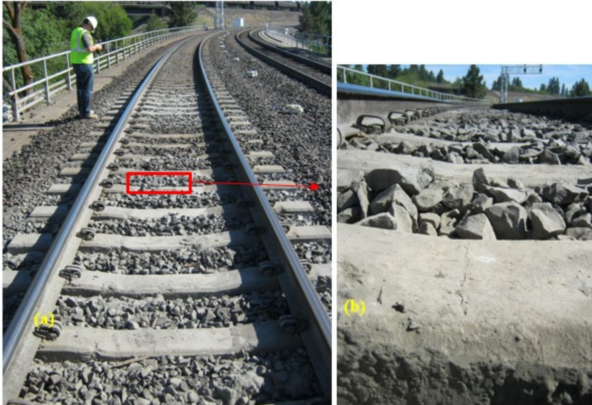
Figure A-4: Moderate binding cracking on ties, Bridge #1
