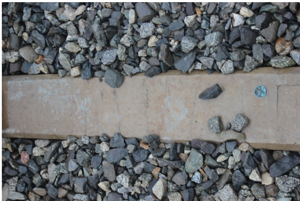
Figure A-28: Tie center cracking, Bridge Approach #3
