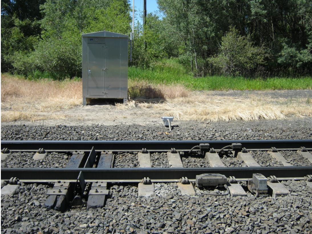
Figure B-7: Insulated joint and signal shed, Signal #1
