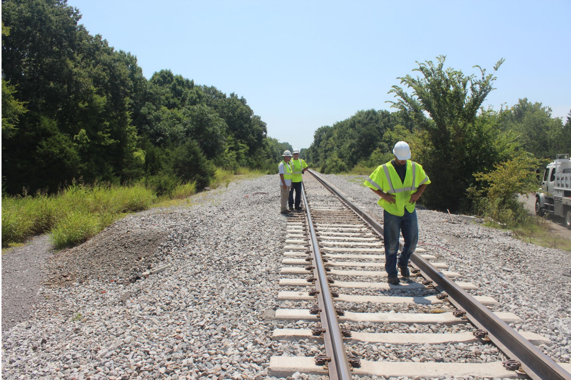
Figure 3-1: Location with concrete tie abrasion damage had grading issues at signal controls
