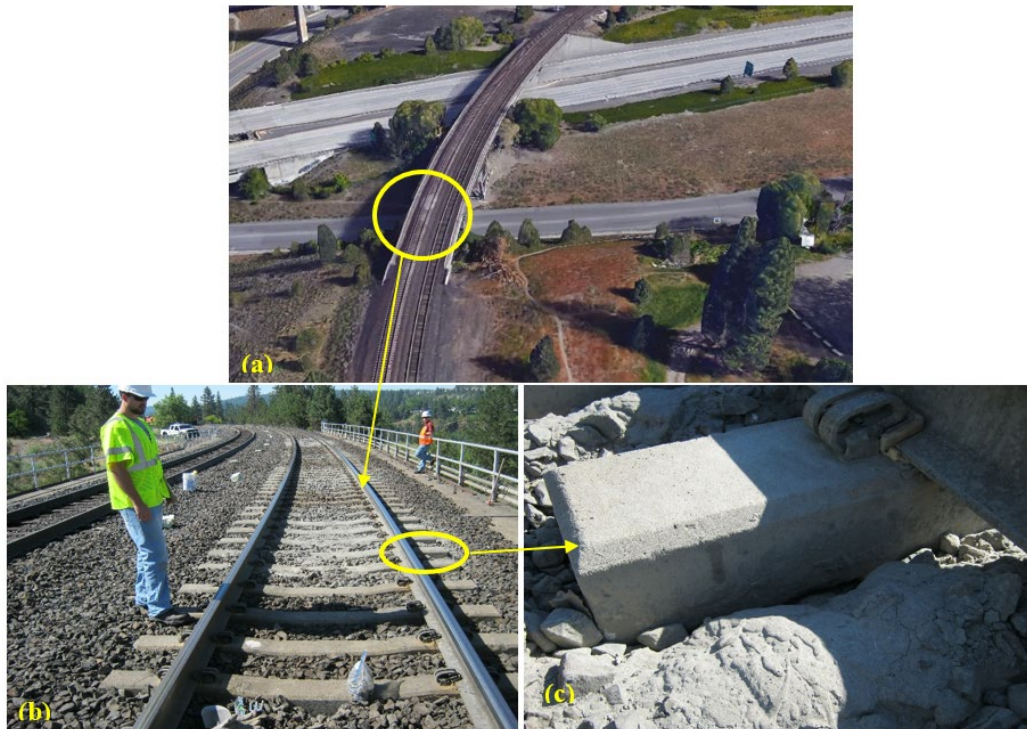
Figure A-1: Gray mud in track is visible in a) satellite image from Google Earth, b) track-level view, and c) up-close view of a concrete tie, Bridge #1
