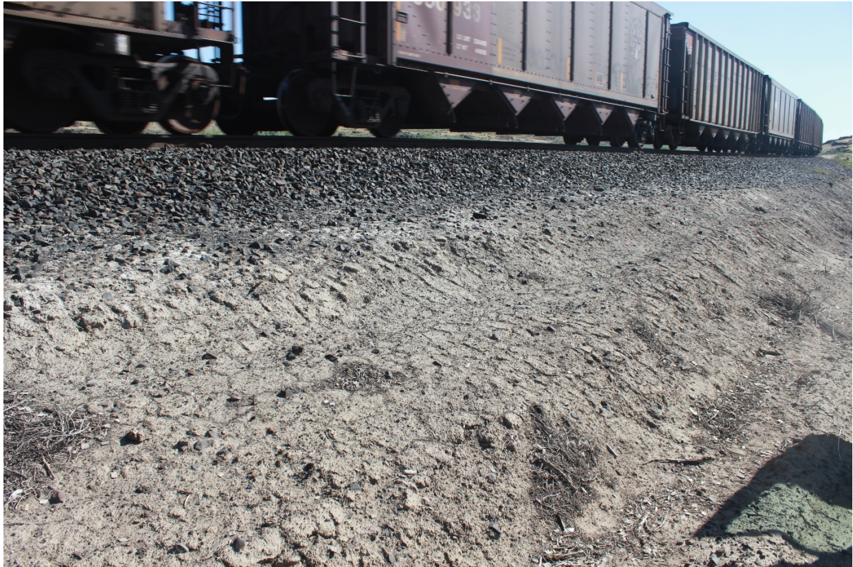
Figure D-12: Mud-flat cracking on track embankment, Curve #2
