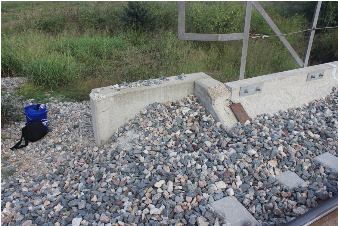
Figure A-9: Ditch in ballast to improve drainage on Bridge #2
