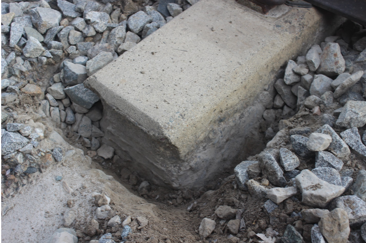
Figure E-40: Tie end wear, Tangent #7
