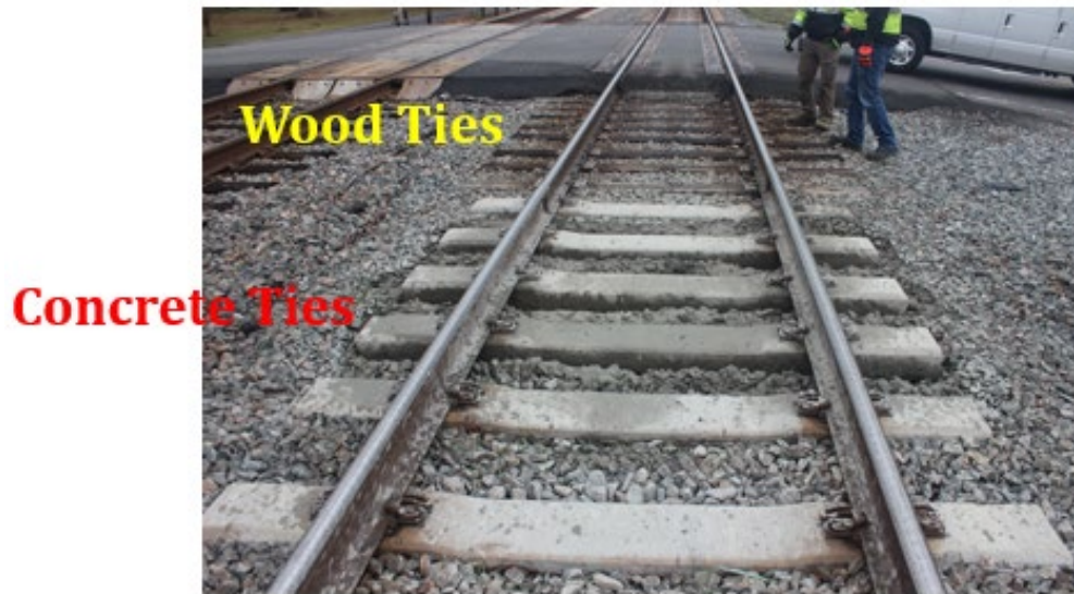
Figure C-27: Concrete-to-wood tie transition, Crossing #5
