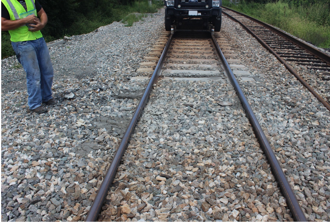
Figure C-54: Mud pumping coming up through crossing ballast and on the edge of Crossing #9
