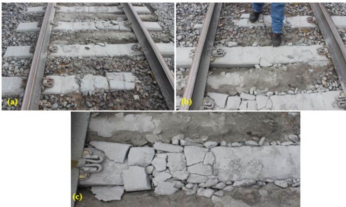
Figure C-16: Shattered ties that began as center-binding cracks, Crossing #3
