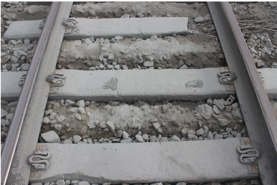
Figure C-14: Ties at locations with mud pumping with severe damage, Crossing #3
