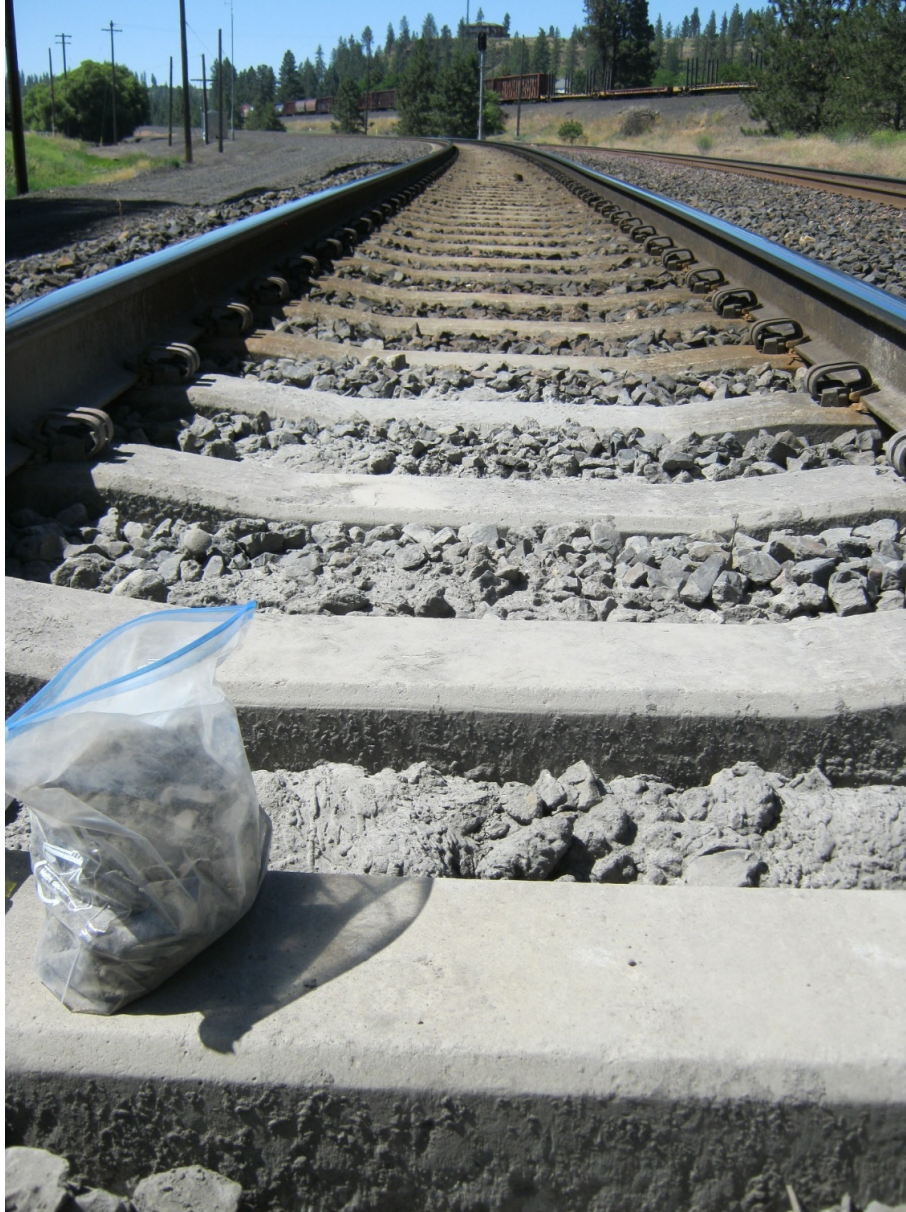
Figure B-4: Gray mud in track, Switch #1
