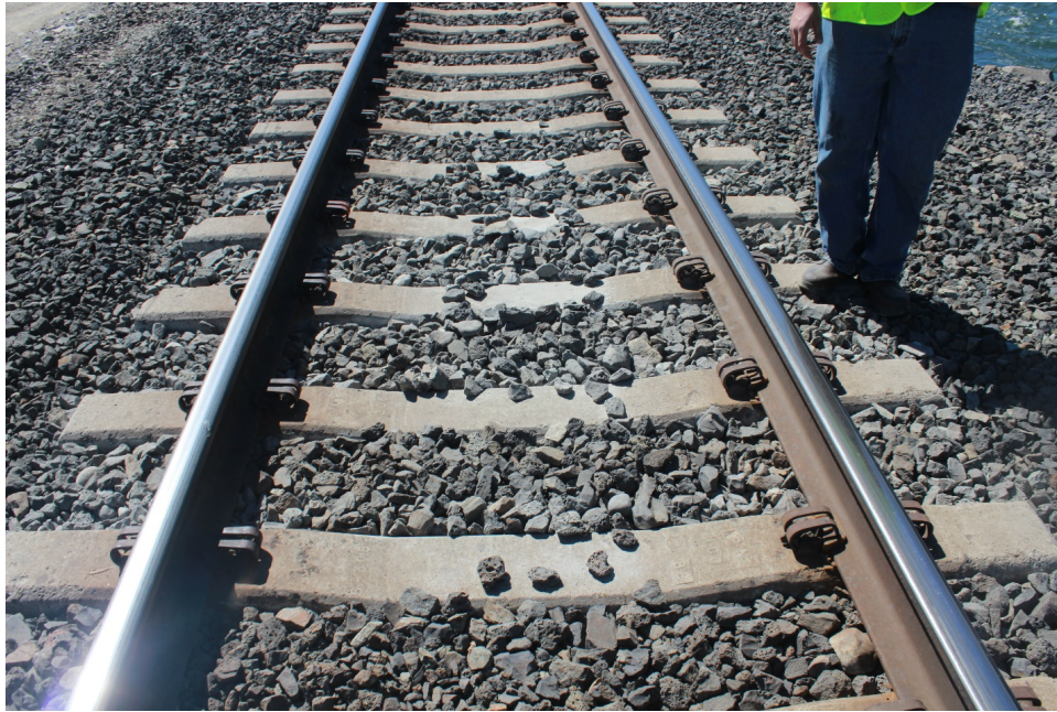
Figure C-10: Minor gray dusting of ballast particles, Crossing #2
