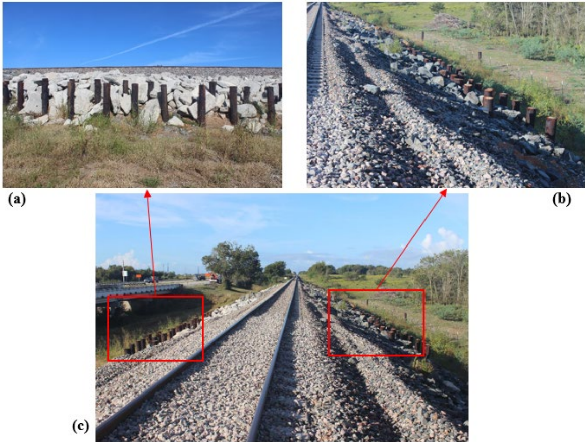
Figure A-21: Use of piles to stabilize the slope, Bridge Approach #1
