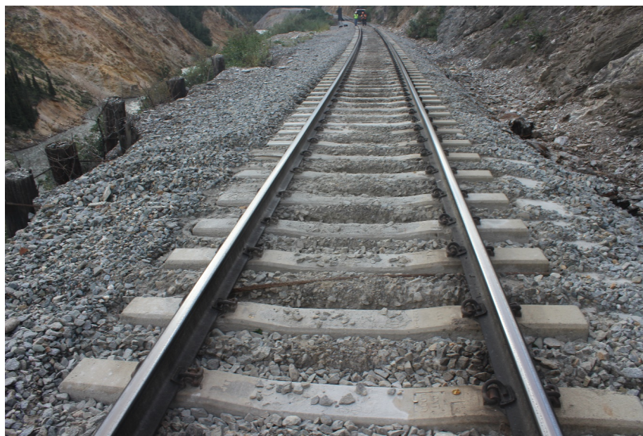
Figure E-37: Trenches dug in ballast to drain water ponding in track, Tangent #7
