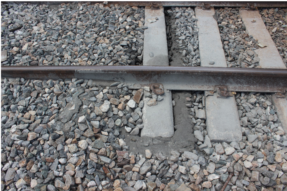
Figure C-55: Mud pumping, Crossing #9
