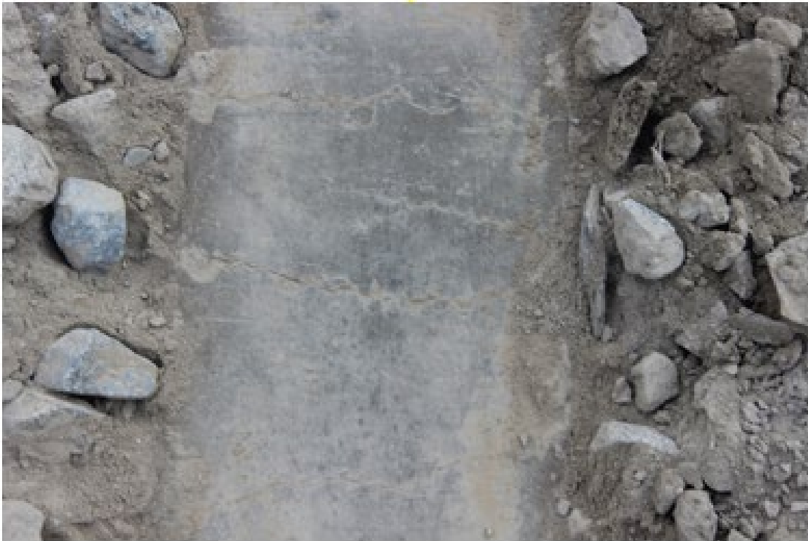
Figure E-34: Tie cracking, Tangent #7
