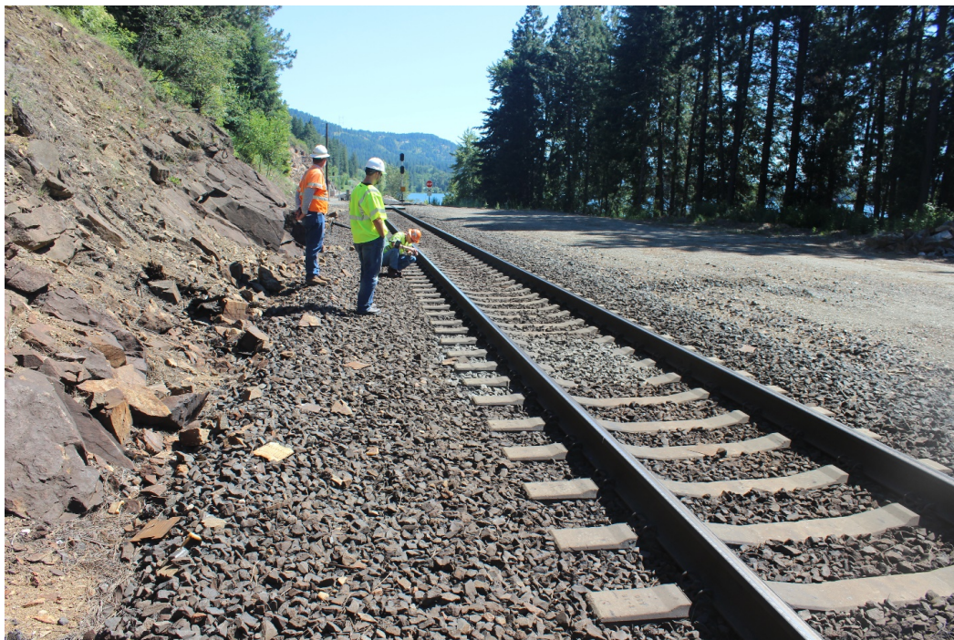
Figure C-7: Grading issues seen in some locations, Crossing #1
