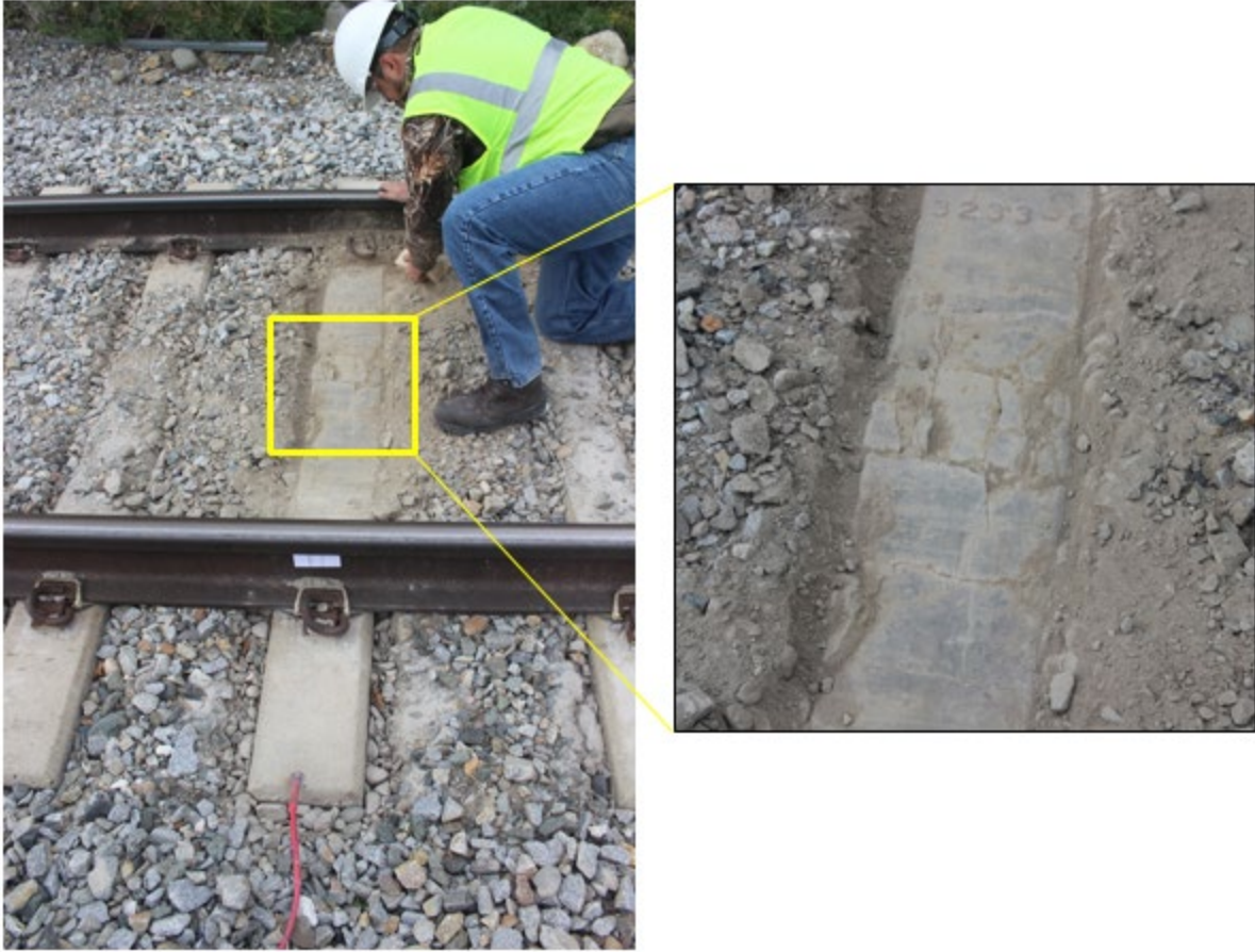
Figure E-48: Tie center binding cracks, Tangent #9
