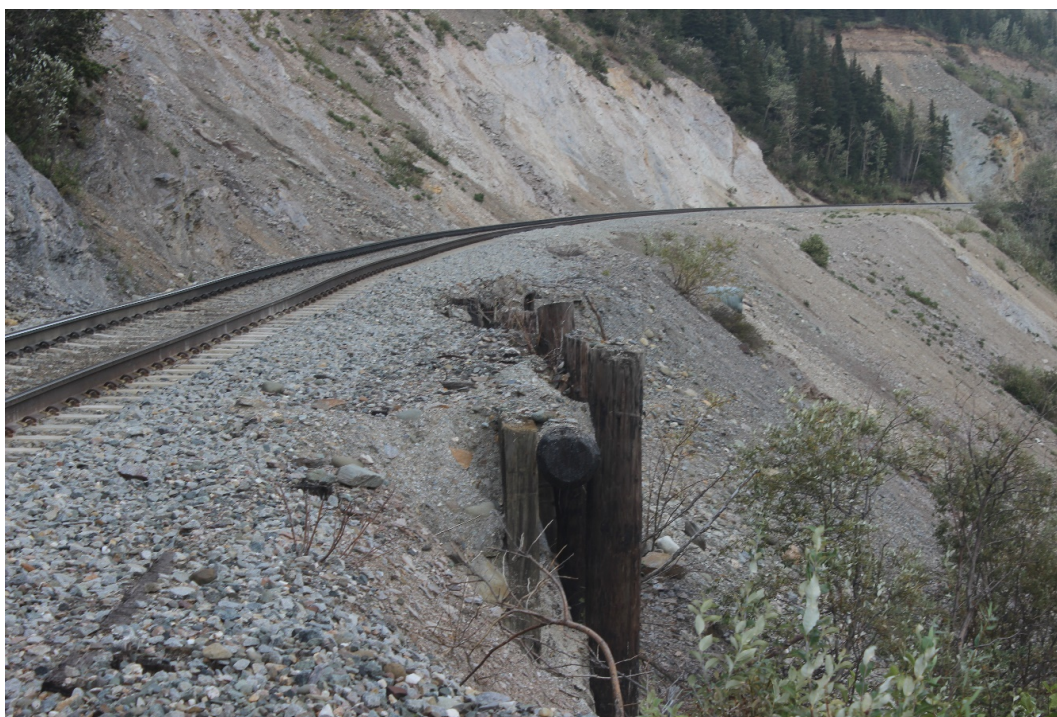
Figure E-39: Drainage pipe crossing under track, Tangent #7
