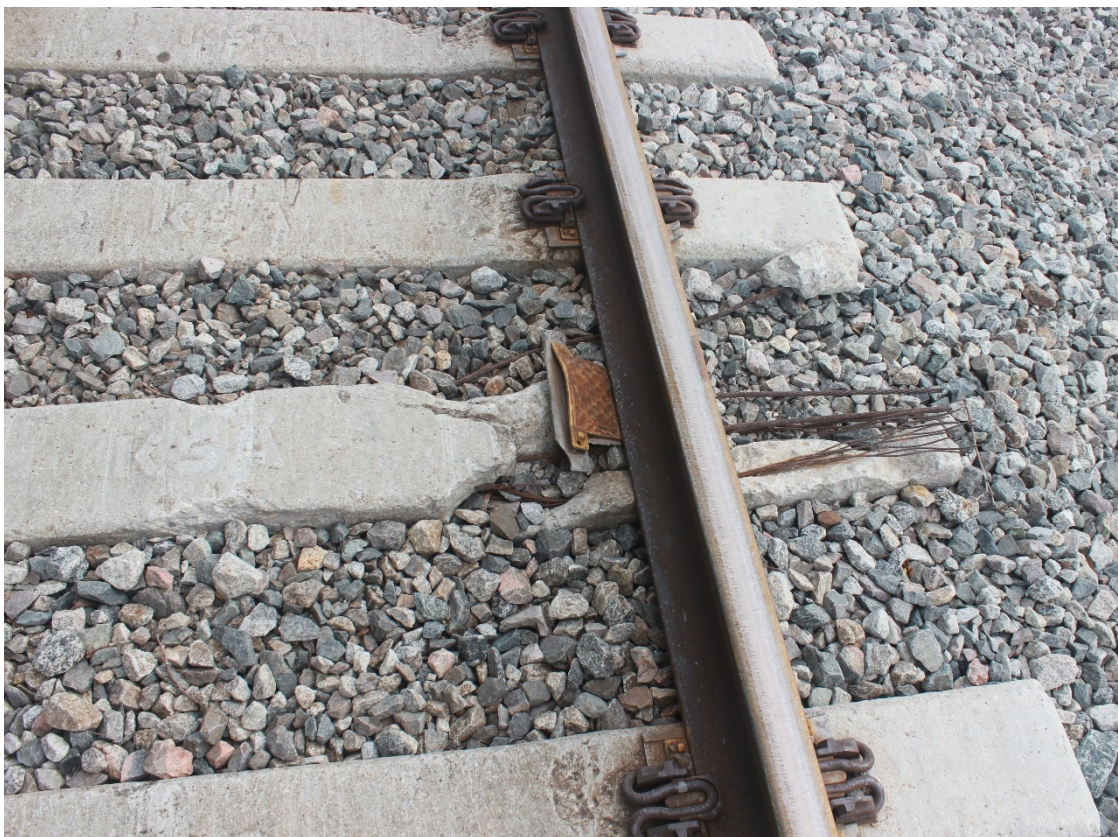
Figure C-15: Damaged tie from broken axle derailment, Crossing #3
