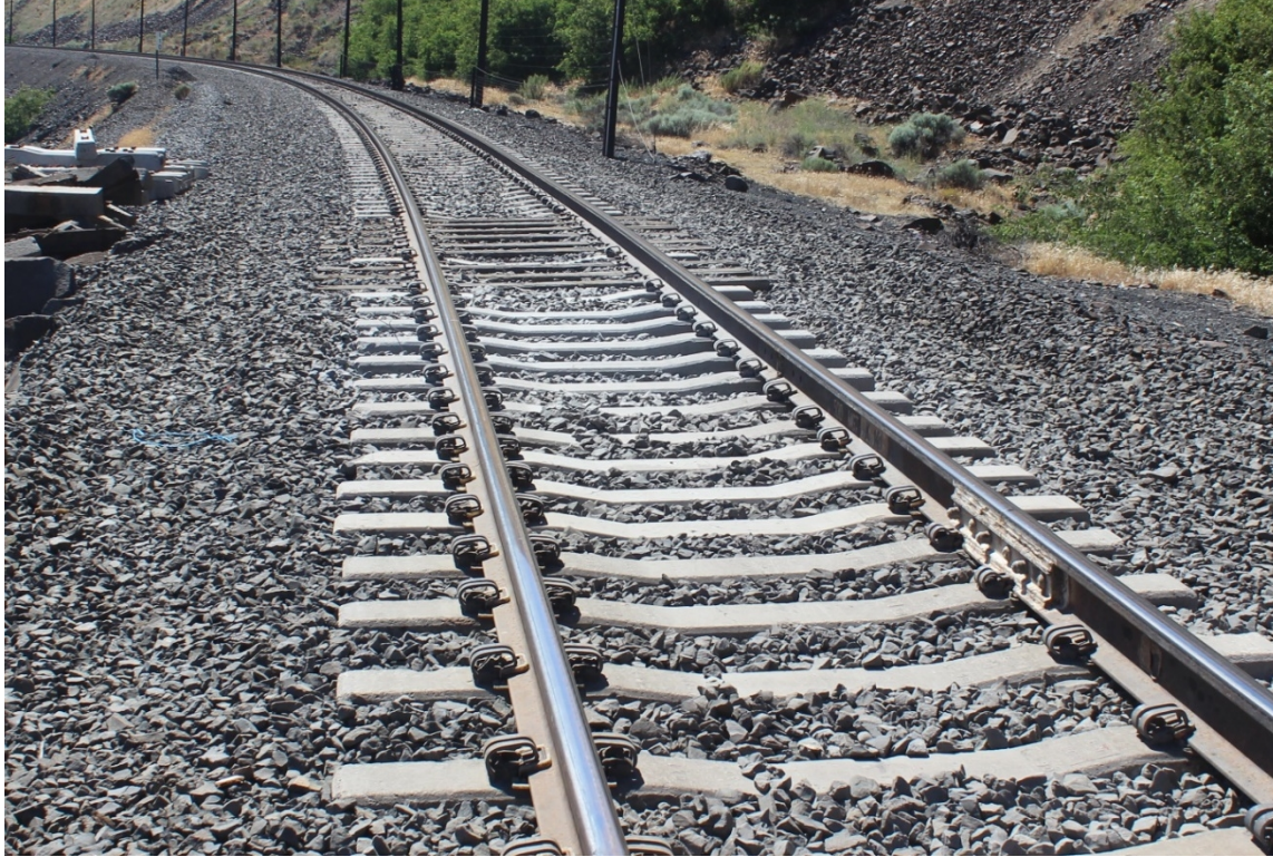
Figure E-8: Pumping on the concrete ties next to wooden ties, Tangent #2
