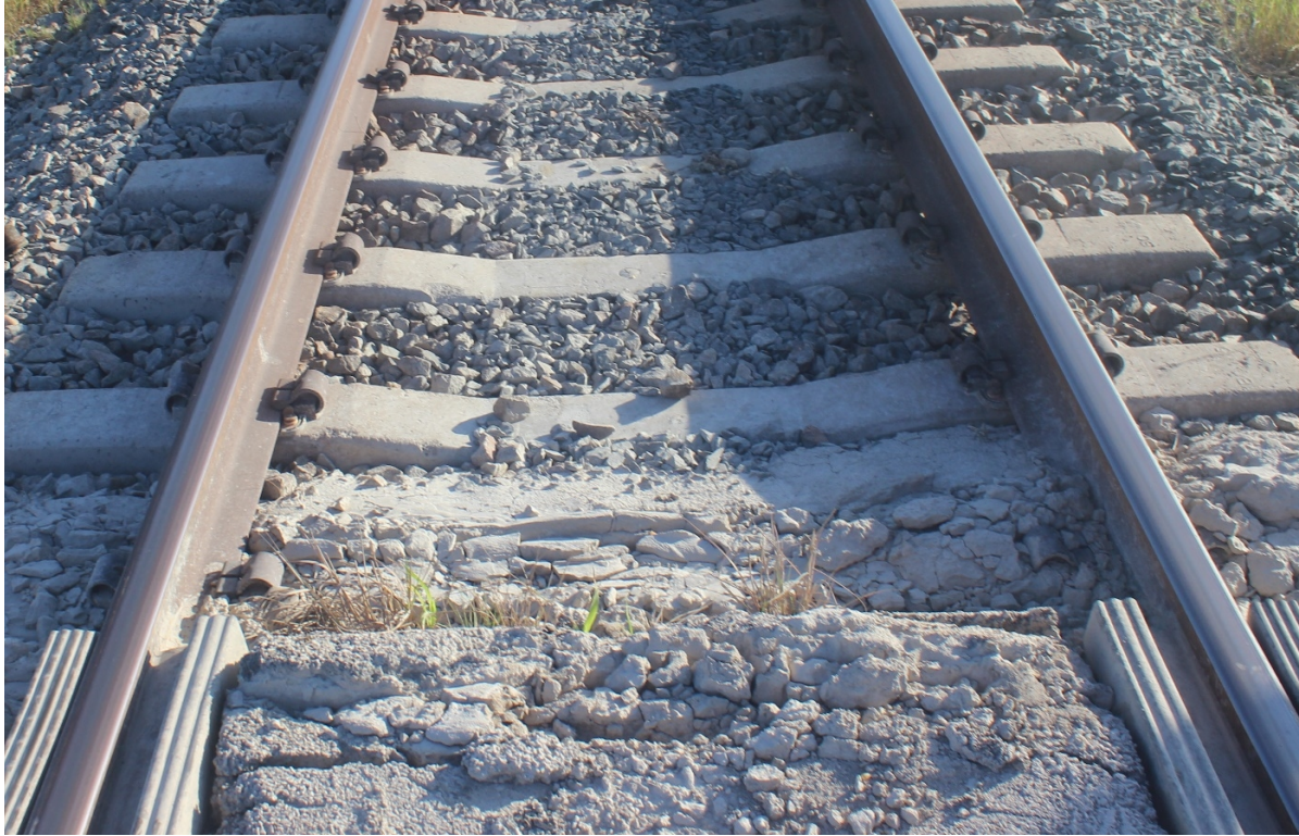
Figure C-22: Excessive pumping and vegetation, Crossing #4
