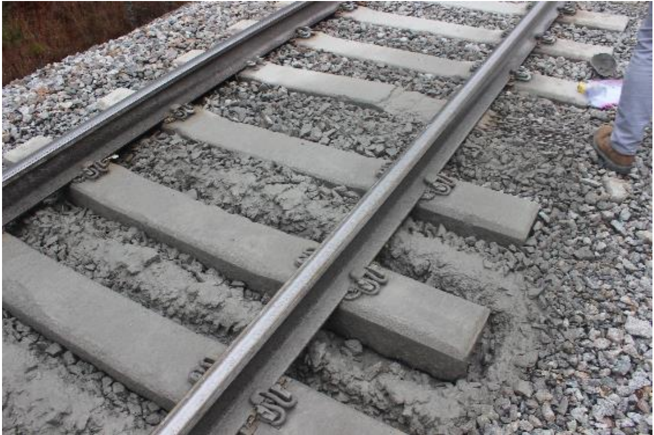
Figure E-23: Mud spot in track, Tangent #6
