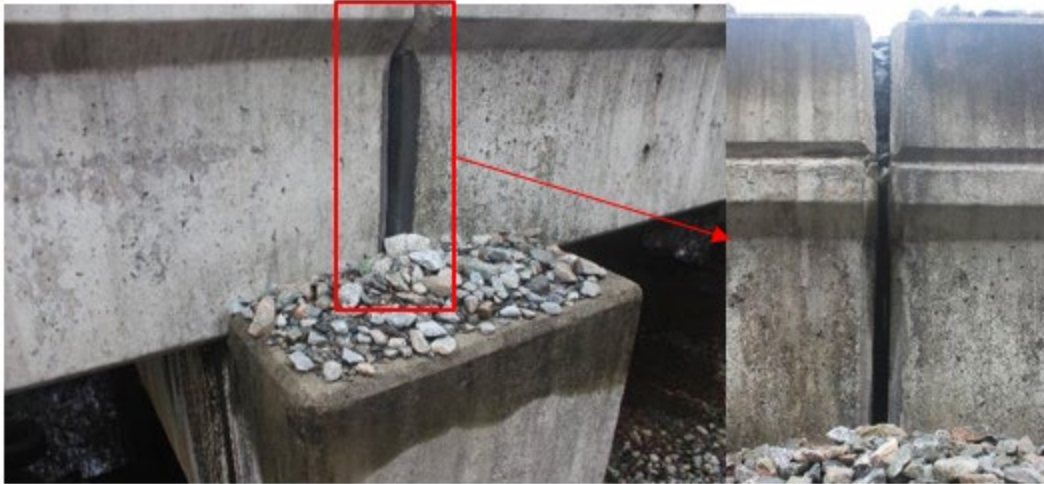
Figure A-15: Drainage issues on Bridge #3
