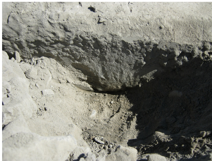
Figure A-3: Fine particles available due to tie abrasion, Bridge #1
