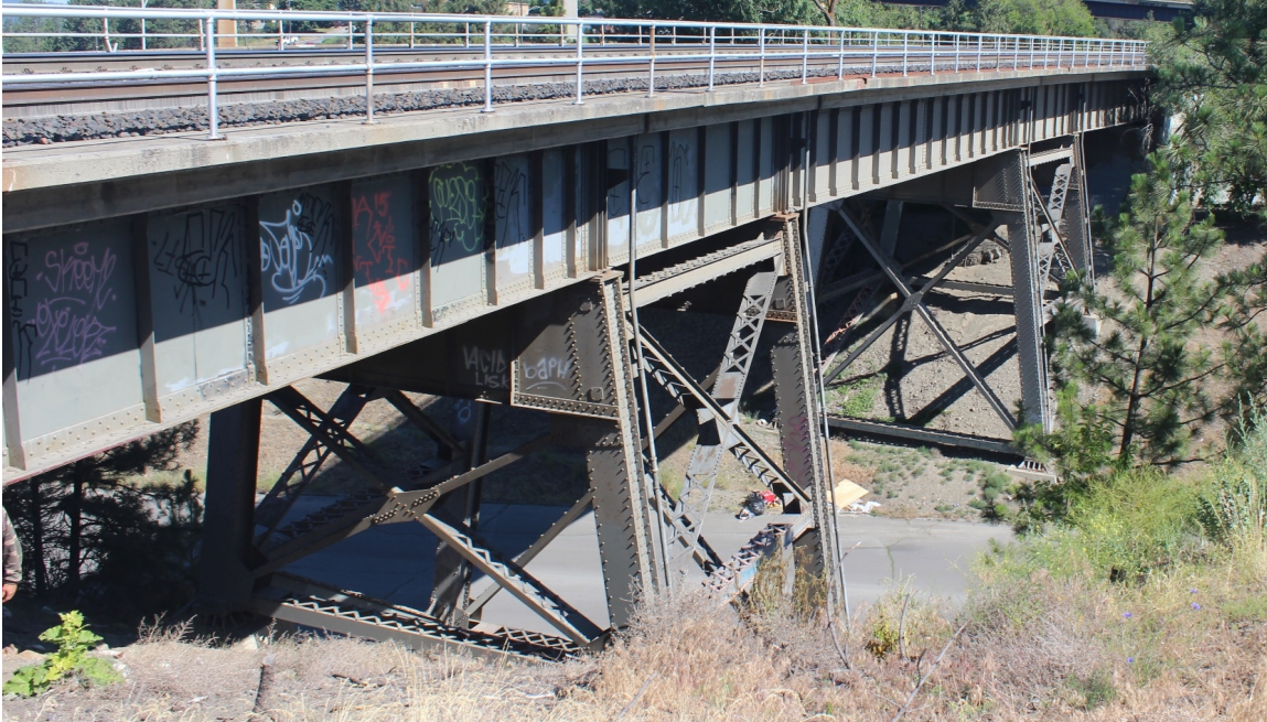
Figure A-2: Bridge superstructure and truss supports, Bridge #1
