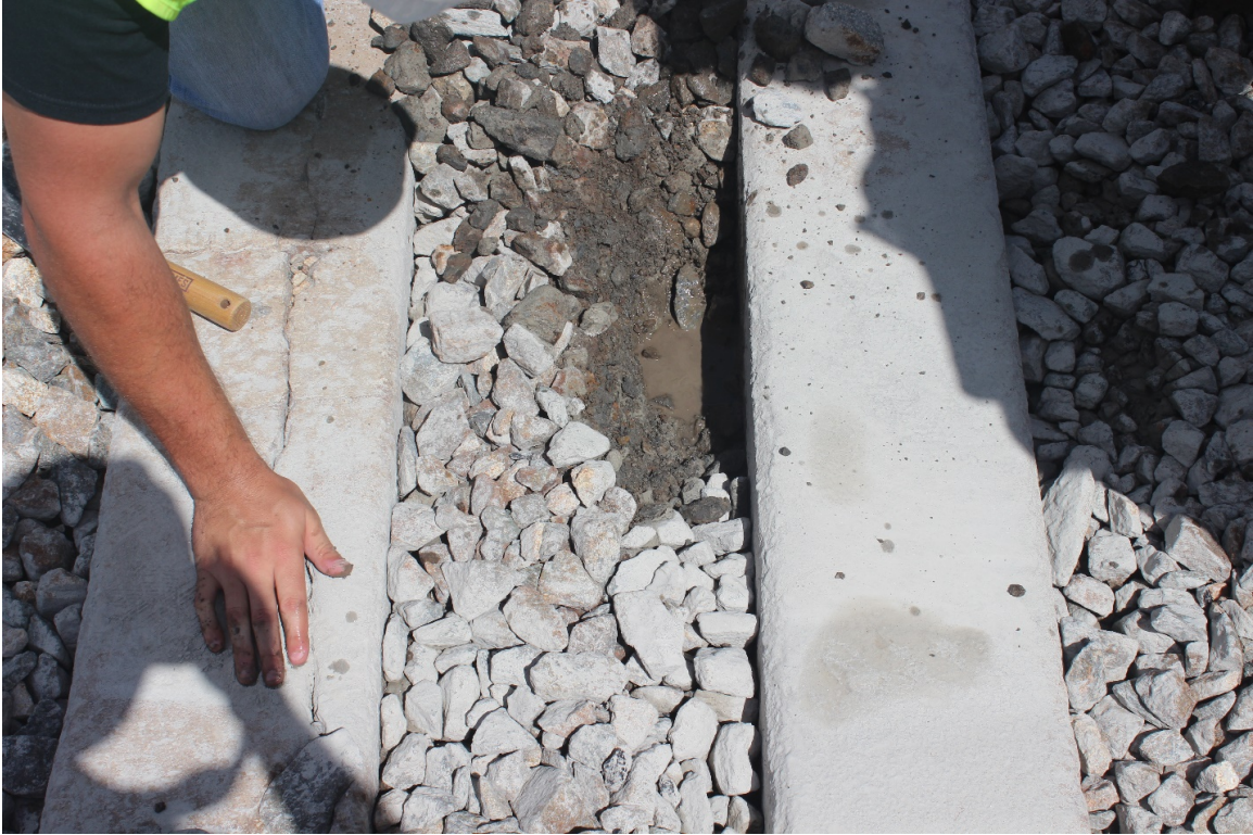
Figure C-38: Mud pumping adjacent to cracked tie, Crossing #6
