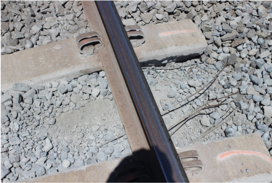
Figure 3-21: Abrasion found on sides of ties with an old tie in between, Curve #3
