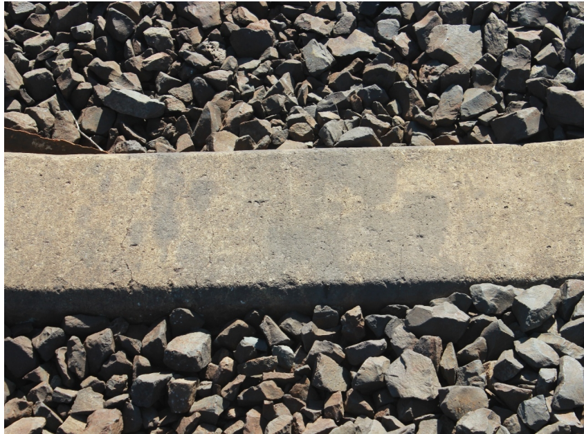
Figure D-9: Minor center-binding cracks, Curve #2
