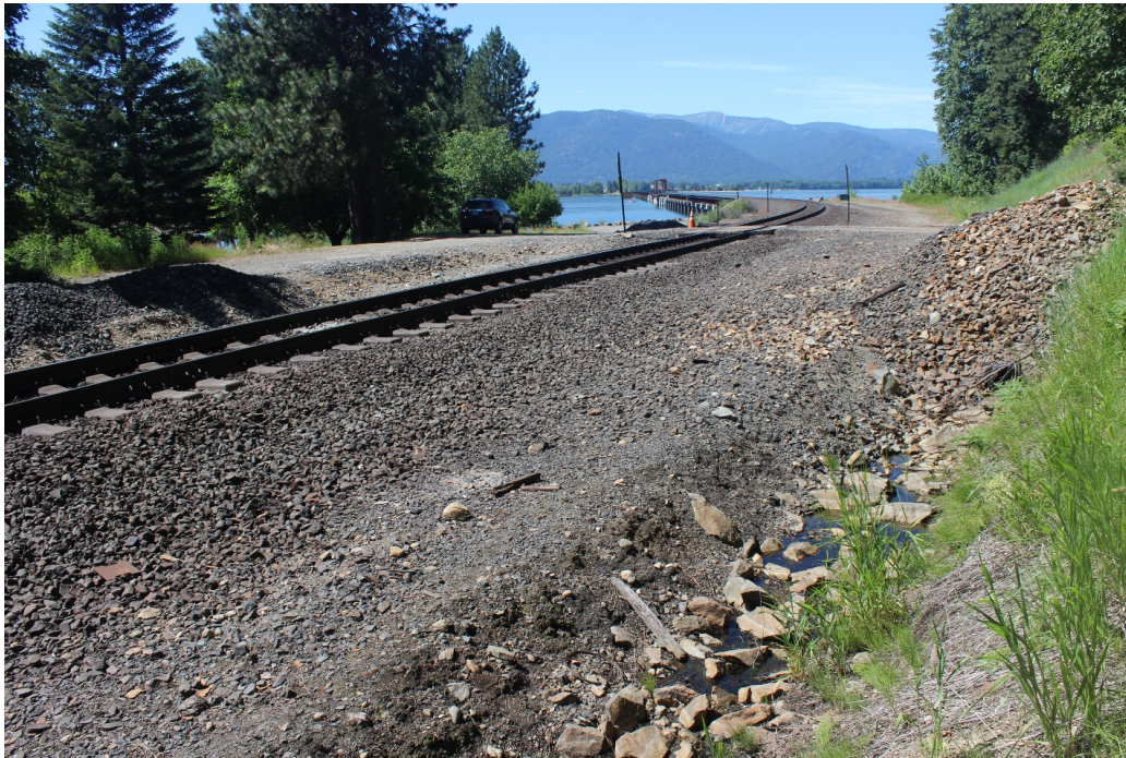
Figure C-6: Standing water and vegetation in ditch, Crossing #1
