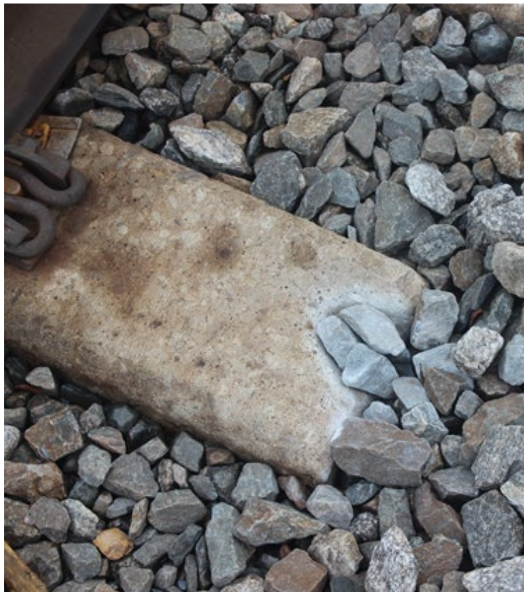
Figure E-27: Abrasion damage at unusual location, Tangent #6
