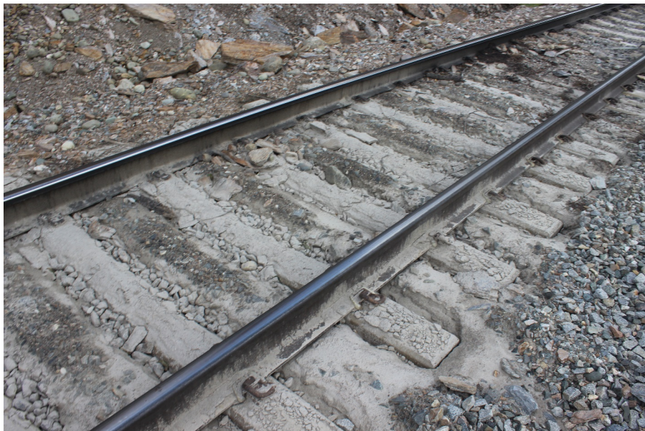
Figure E-33: Severe pumping, Tangent #7
