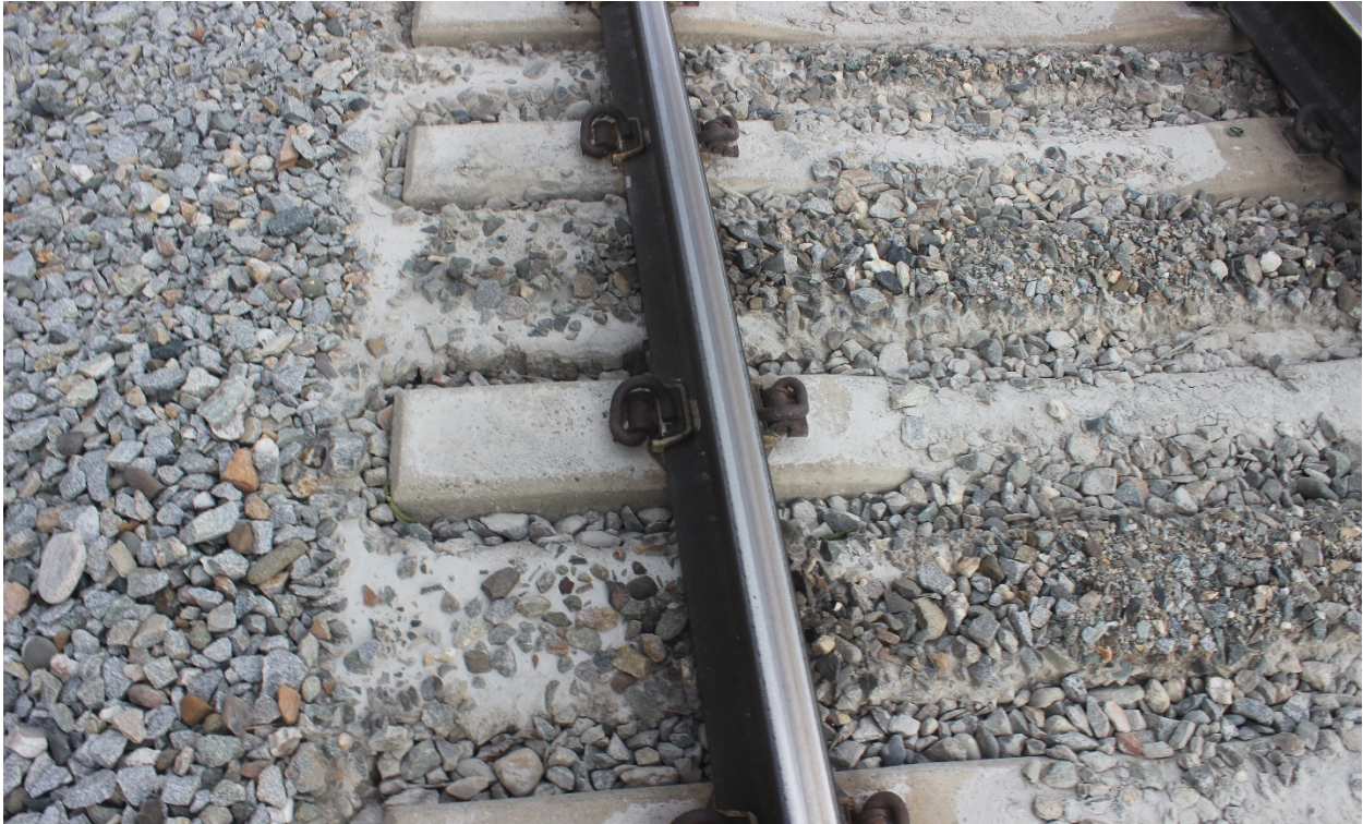
Figure D-23: Pumping seen in track, Curve #5
