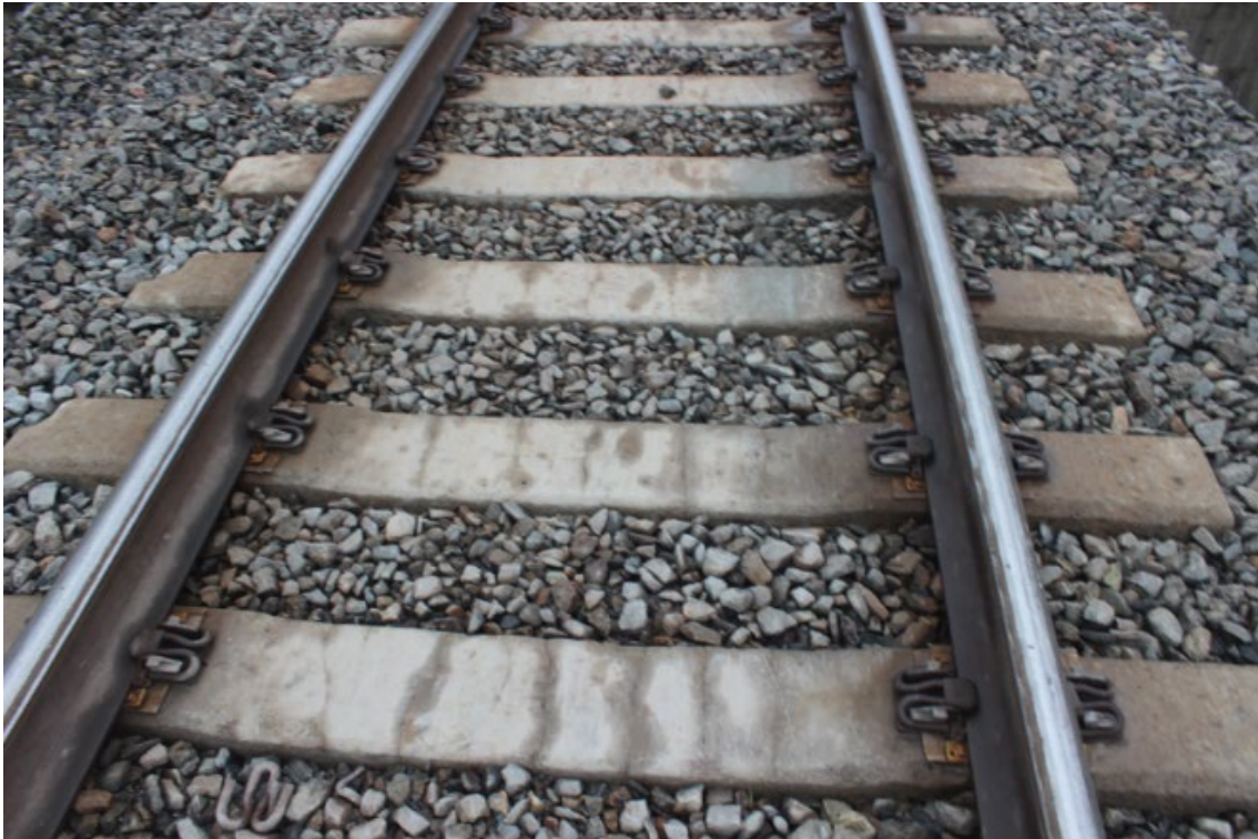
Figure A-17: Moderate center binding cracking, Bridge #3
