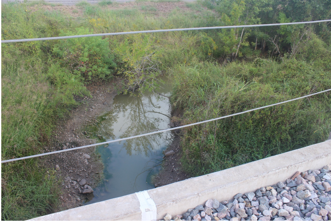
Figure A-5: Stagnant water under Bridge #2
