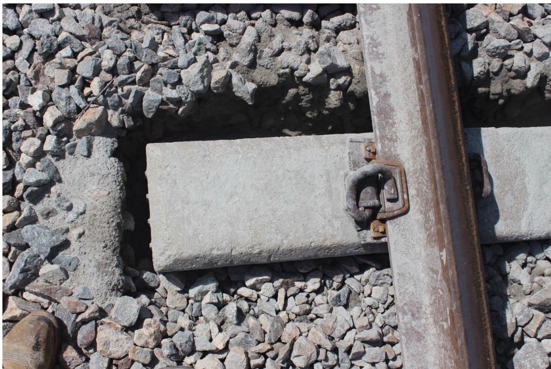
Figure E-56: Tie pumping, Tangent #11
