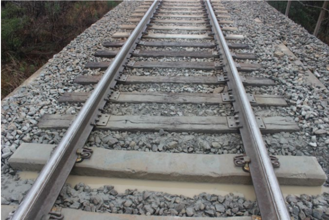
Figure 3-3: Bridge #3 section repaired with wooden ties
