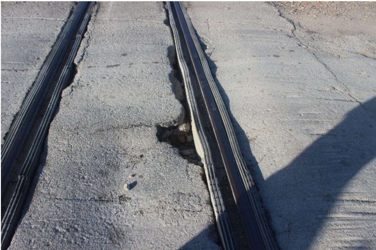
Figure C-23: Asphalt crossing defects, Crossing #4
