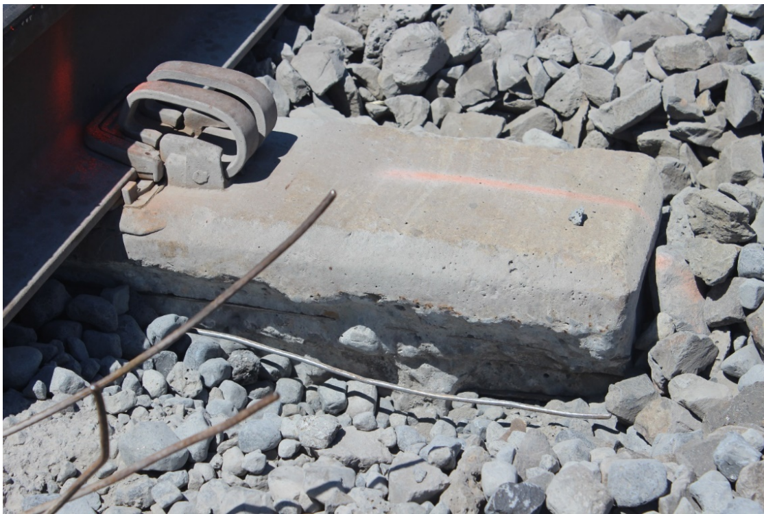
Figure 3-22: Close-up view of tie with side abrasion, Curve #3
