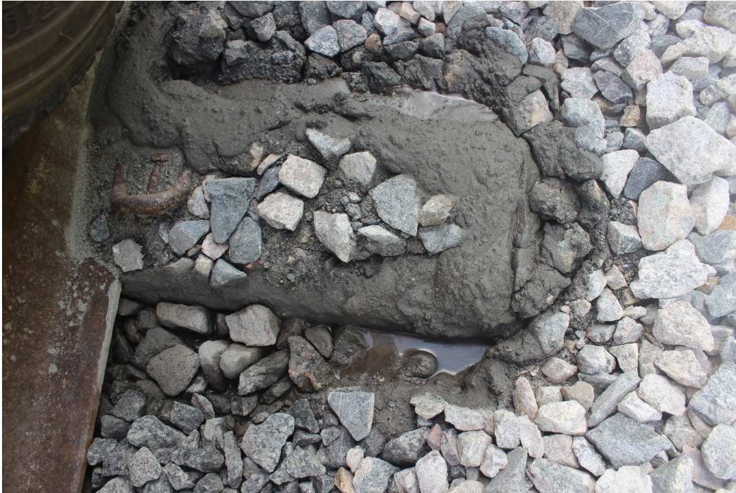
Figure C-46: Asphalt pieces are present in the fouled ballast, Crossing #8
