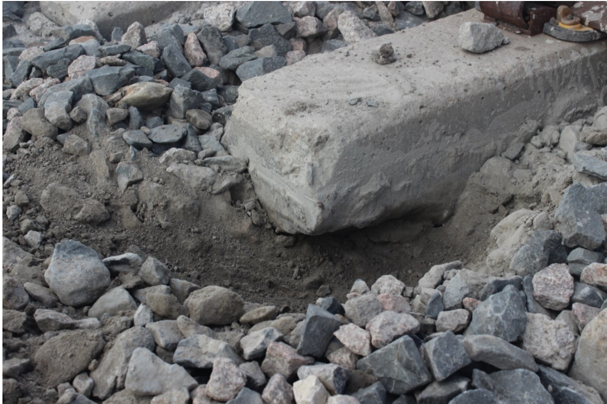
Figure A-23: Rounding of tie bottom, Bridge Approach #2
