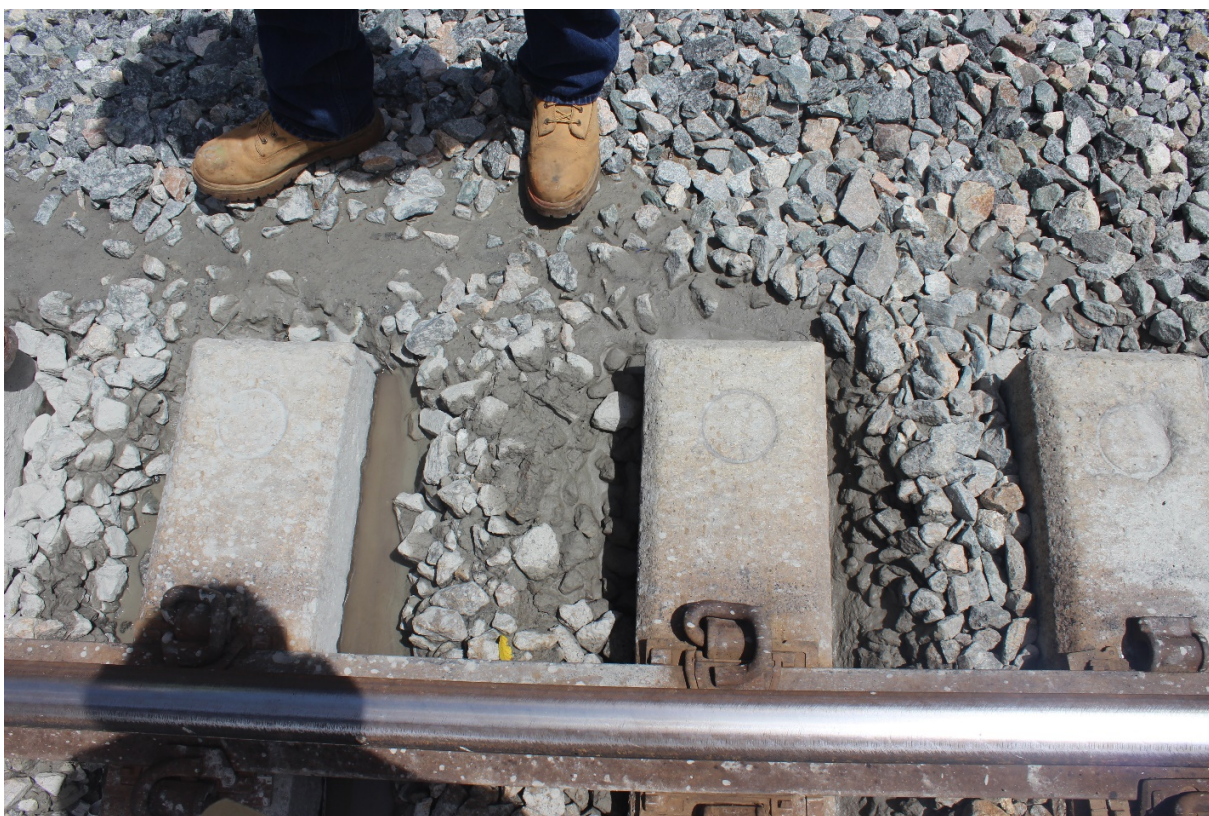
Figure E-54: Fine particles and water in track, Tangent #10
