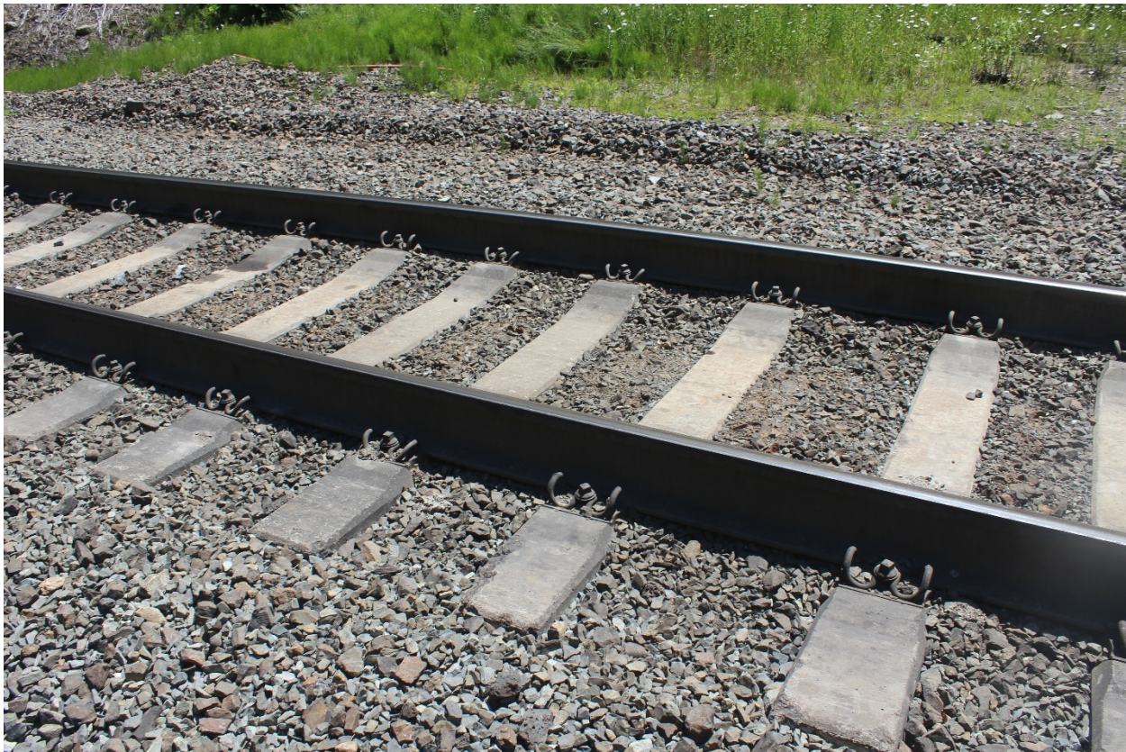
Figure A-35: Ballast fouling in track, tunnel approach
