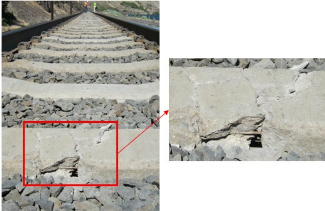
Figure E-3: Severe center binding cracking and exposed reinforcements, Tangent #1
