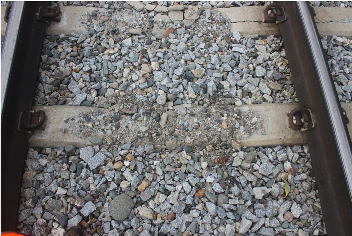
Figure E-47: Damaged ties, Tangent #9
