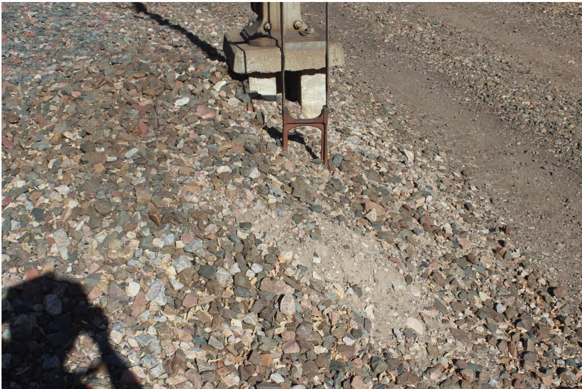
Figure D-18: Fines on the side of the track
