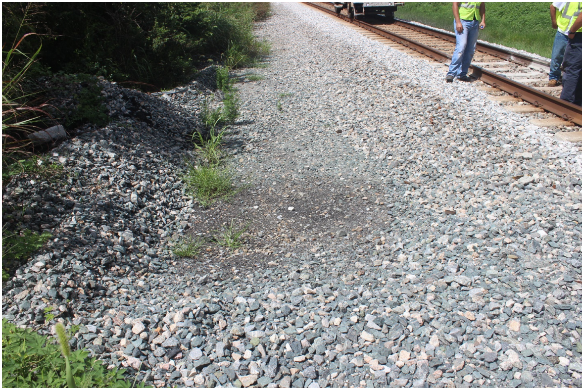
Figure C-39: Fines seen on the ballast shoulders, Crossing #6
