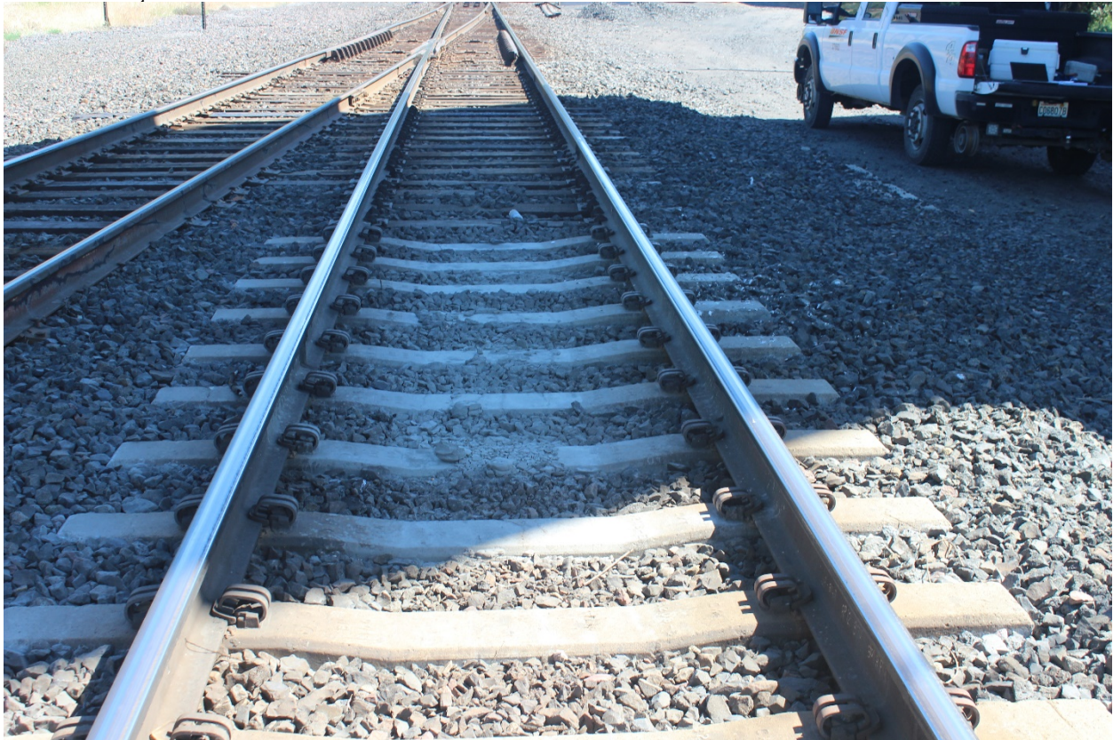
Figure B-2: Fouled ballast immediately after wood-to-concrete tie transition, Switch #1
