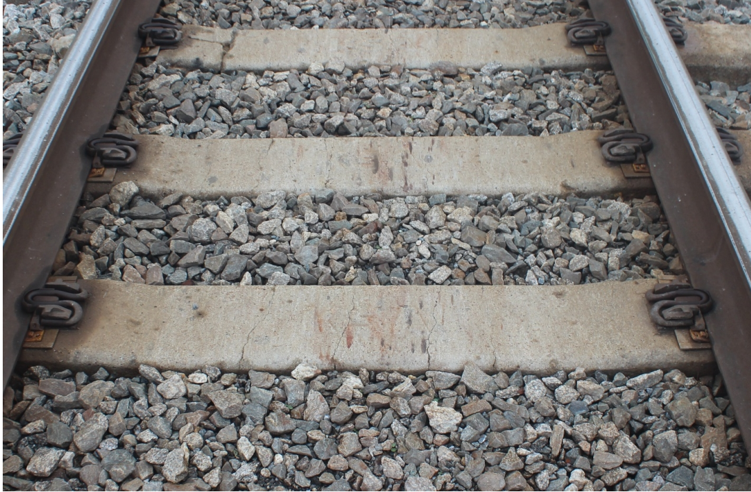
Figure E-26: Center-binding cracking in ties near the fouled ballast location, Tangent #6
