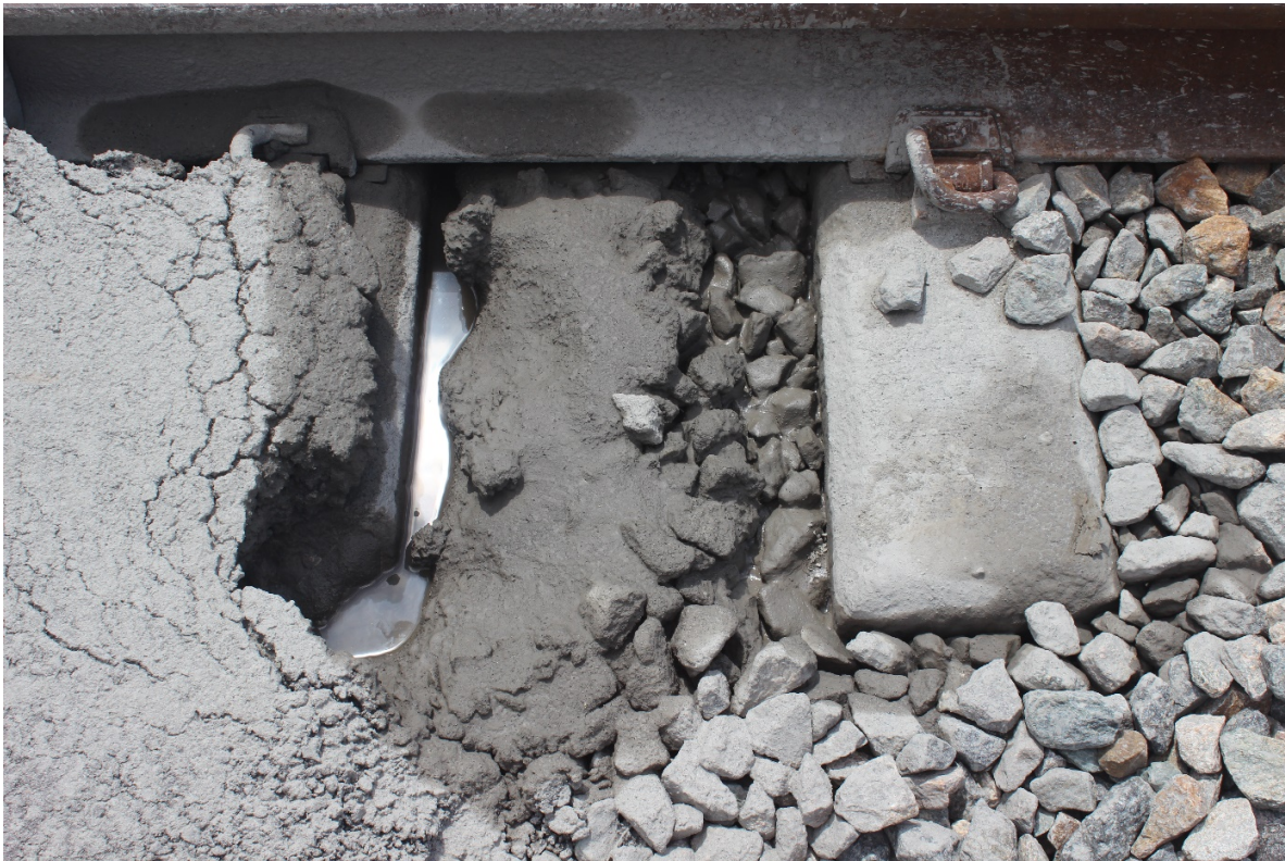
Figure C-43: Ballast fouling adjacent to Crossing #7
