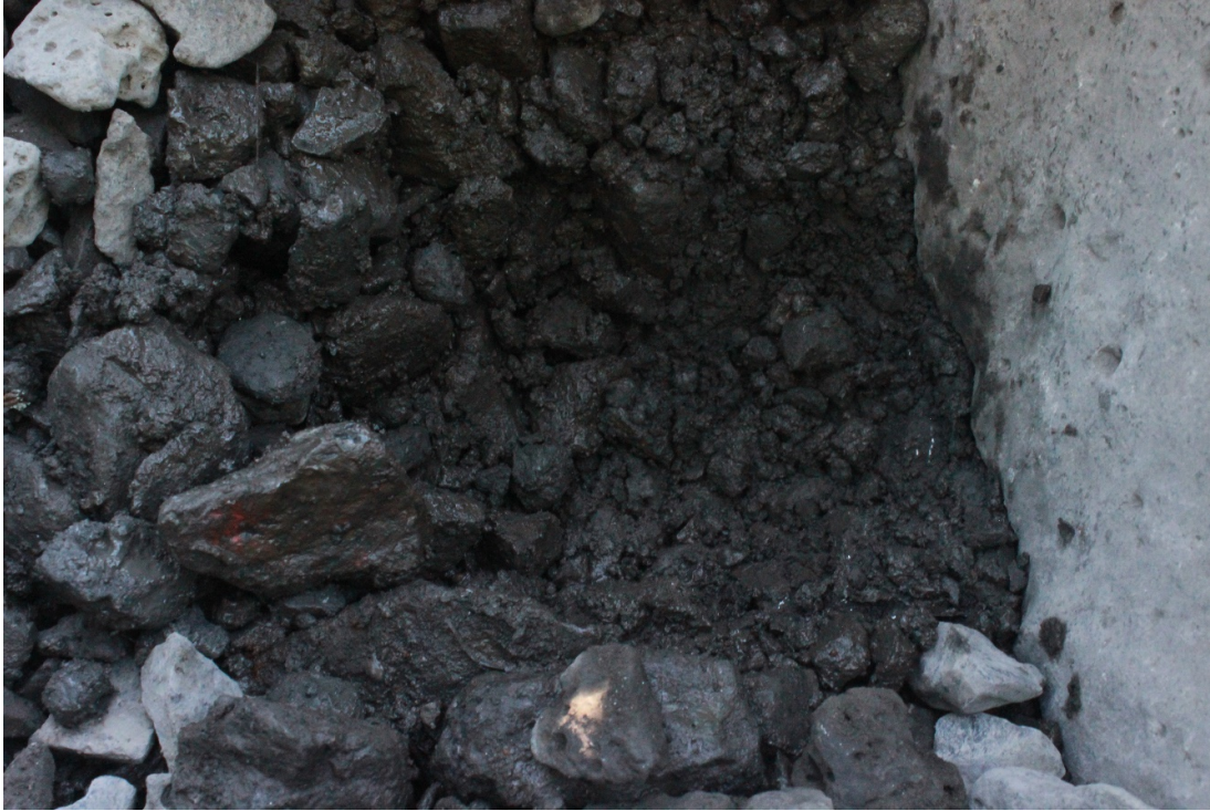
Figure C-4: Ballast fouling and beginning of concrete tie wear, Crossing #1
