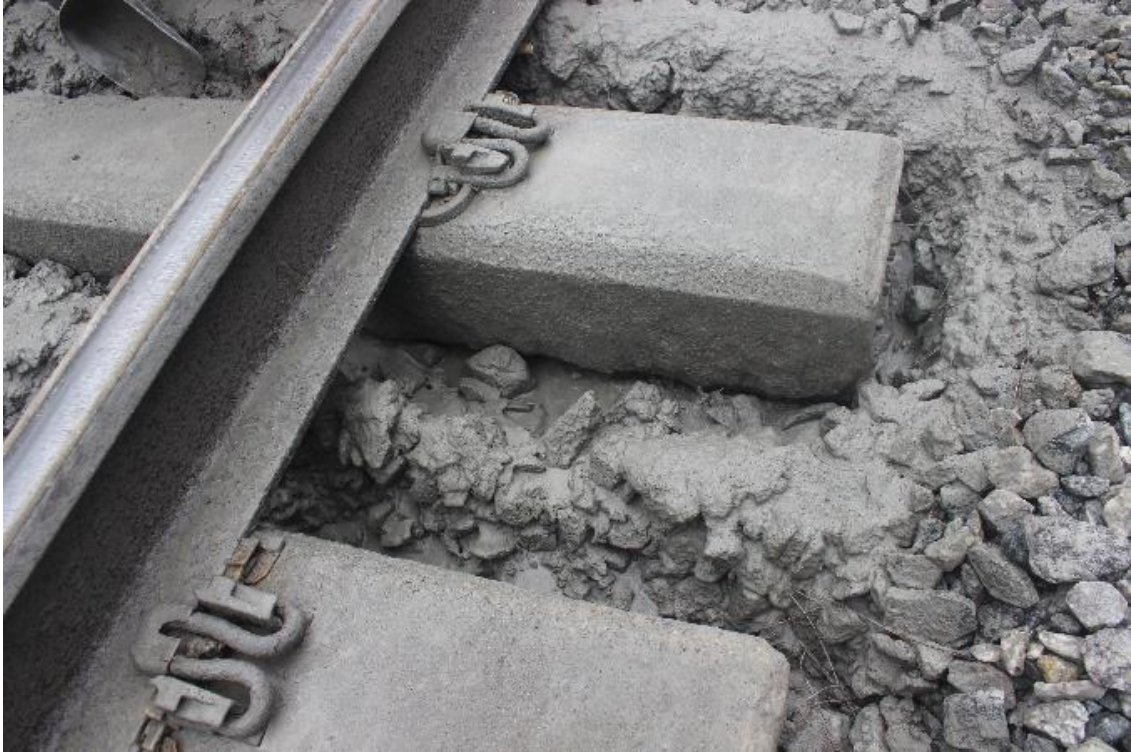
Figure E-24: Pumping in track, Tangent #6
