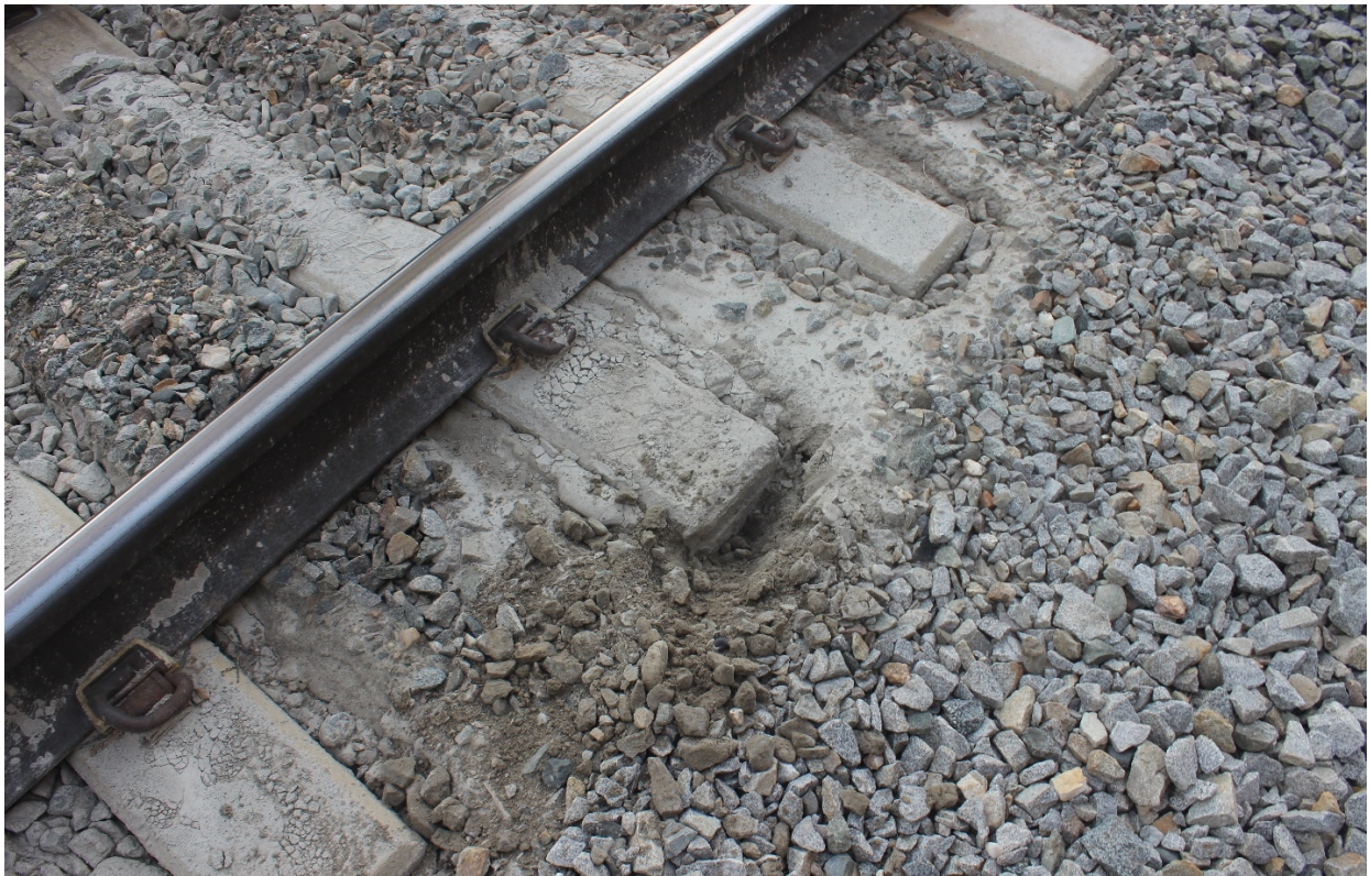
Figure D-24: Fine particles seen at the track surface, Curve #5
