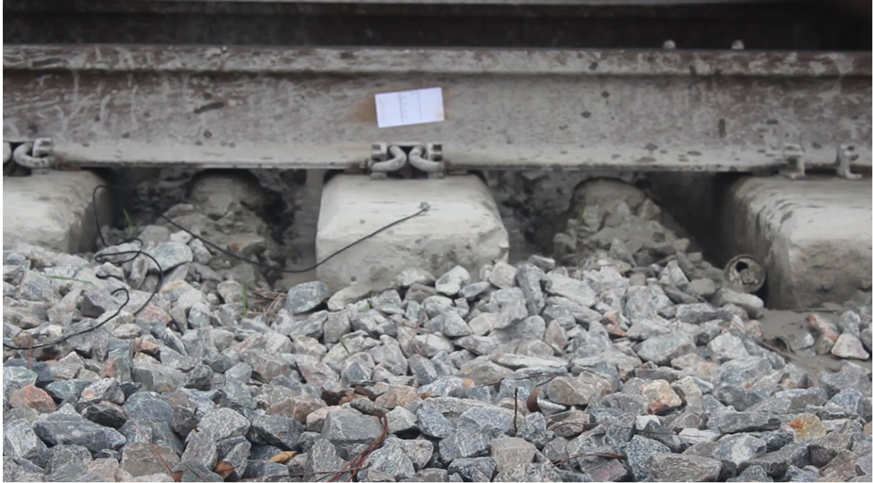
Figure C-33: Track video screenshot with tie at low position during train pass, Crossing #5
