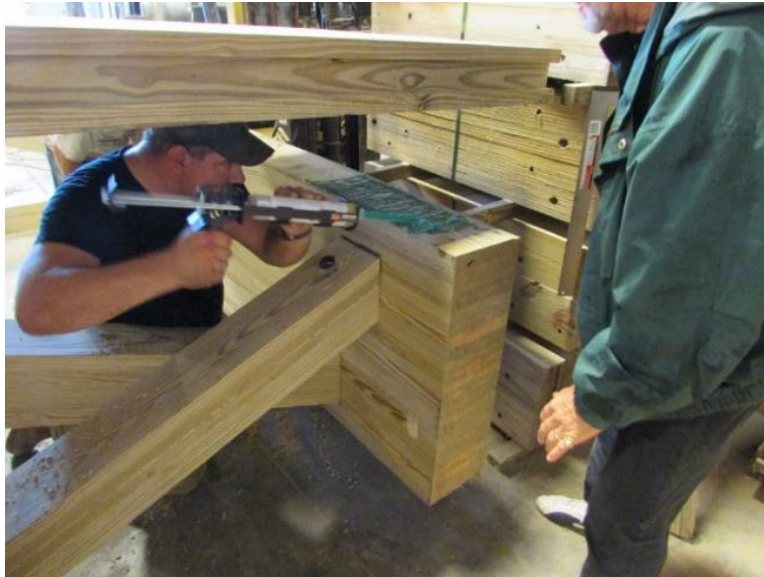
Figure 3.23 Epoxy Deck-to-Stringer Connection
