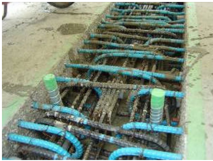
(a) Photograph of Longitudinal Joint
