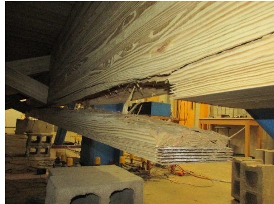
(b) Failure of West Girder
