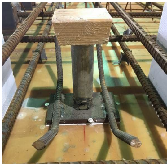
Figure 5.3 Leveling Bolt Construction Detail
