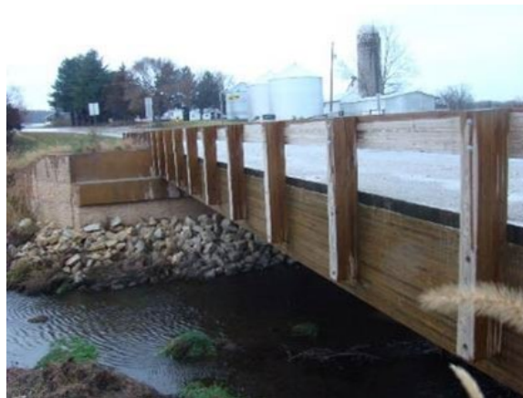
Figure 3.16 Glulam Timber Bridge in Buchanan County, Iowa
