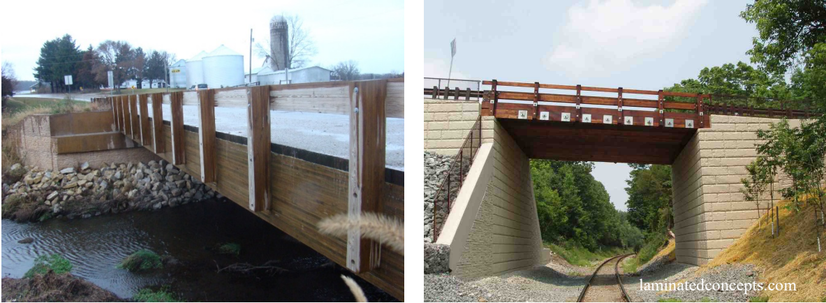
Figure A.16 Timber Railing for Timber Bridges
