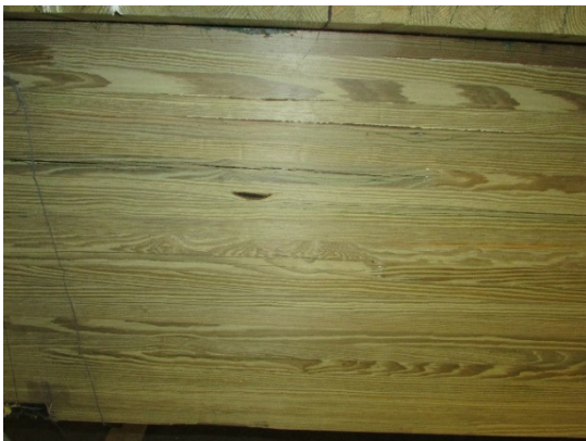
(e) Condition of East Girder at Mid-span
