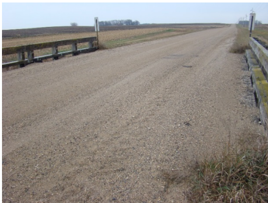
(c) Aggregate Overlay
