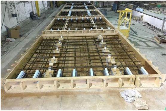
(a) Panel Formwork
