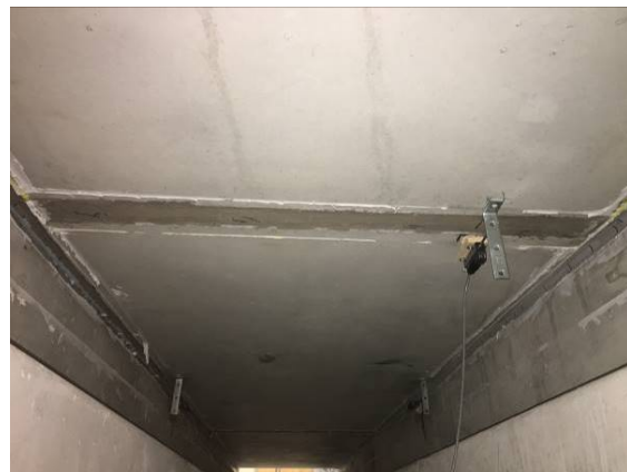
(b) Joint Latex Modified Concrete – Deck Underneath
