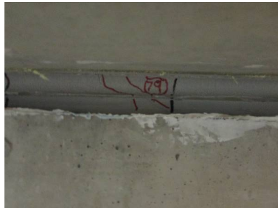
(b) 14-ft South of Mid-Span (Girder B)
