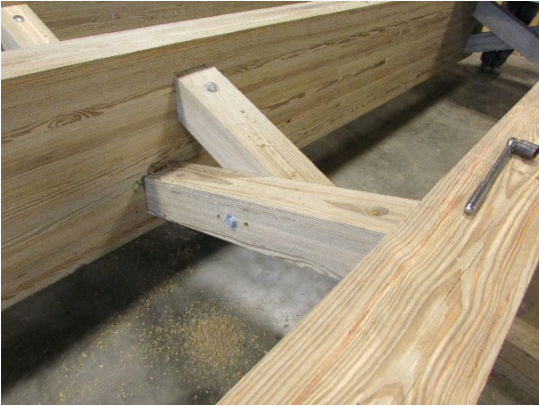
(a) Installation of Cross Braces
