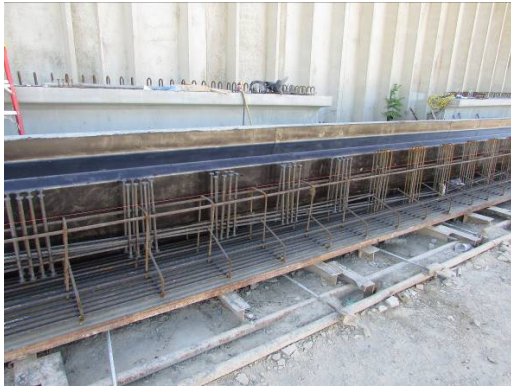
(a) Placement of Bars and Prestressing Strands
