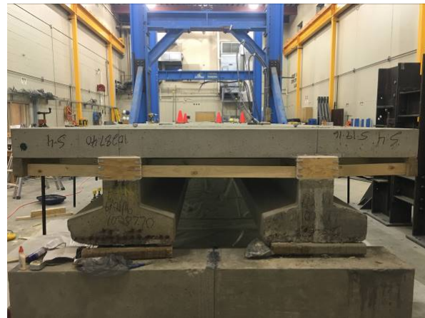
Figure 4.12 Grout Haunch Region Formwork
