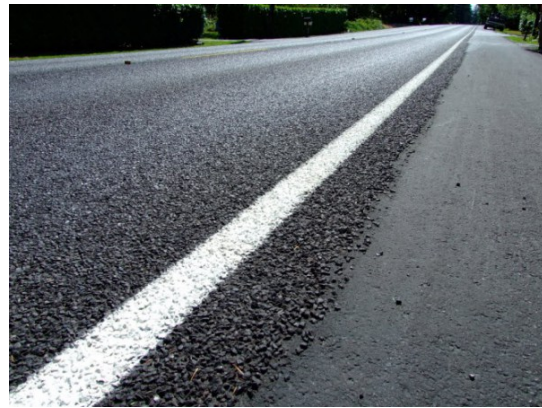
(b) Asphalt Chip Seal (after Gruen-Wald 2011)
