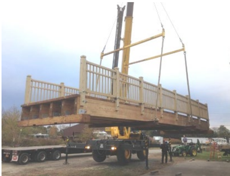
Figure 3.32 Erie Canal Bridge Being Placed in Port Byron, NY, in 2014 (laminatedconcepts.com)
