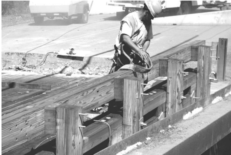
Figure 3.30 Railing on a Glulam Bridge (laminatedconcepts.com)
