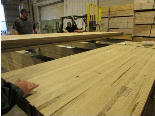
(e) Placement of Second Panel
