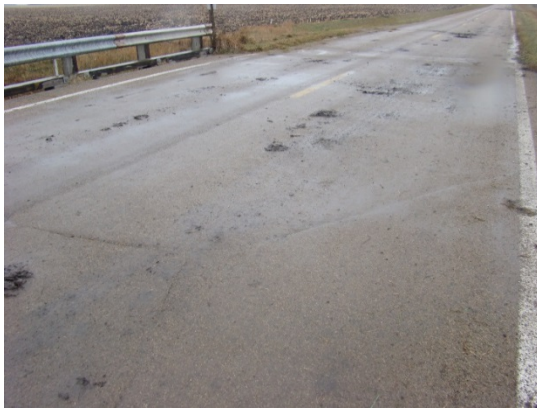
(a) Asphalt Overlay
