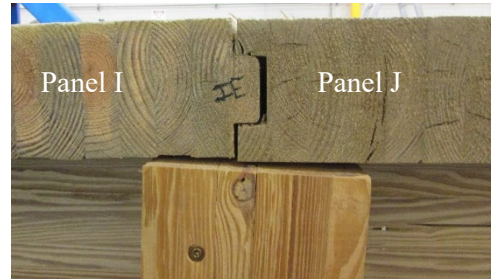
(c) Panel I-to-J Connection at 250,000 Cycles
