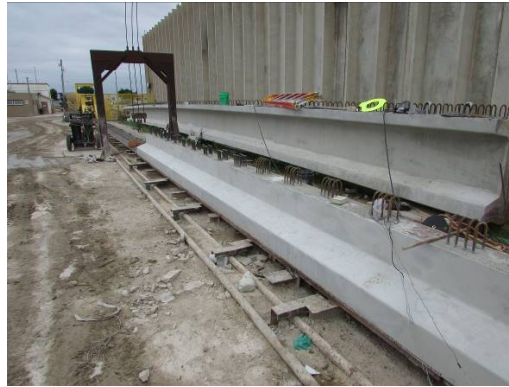
(b) Formwork Removal
