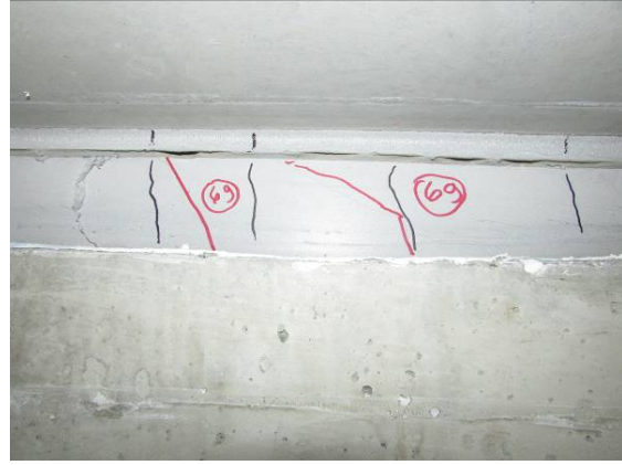
(b) 14-ft South of Mid-Span (Girder A)
