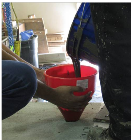
(a) Pouring in Hidden Pockets
