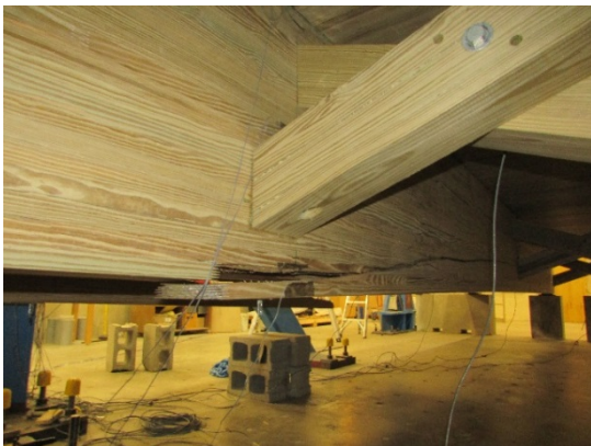
(c) Failure of Interior Girder
