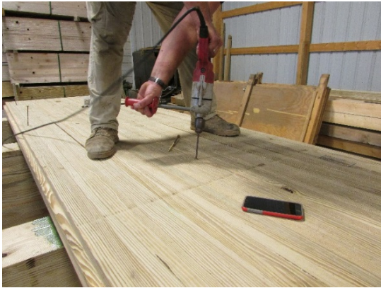
(c) Drilling GRK Screws
