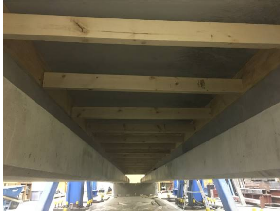
Figure 5.4 Grouted Haunch Region Formwork Installed between Girders
