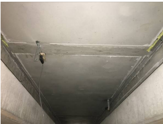
(a) Joint with Non-Shrink Grout – Deck Underneath
