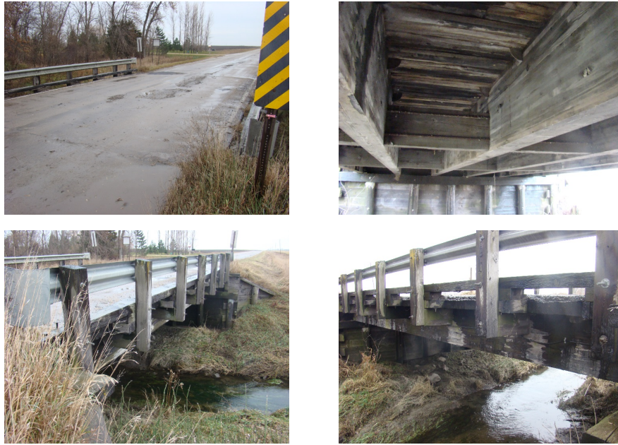
Figure 3.28 Glulam Timber Bridge No. 9967 in Faribault County, Minnesota
