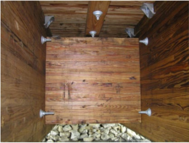
(a) Solid Glulam Diaphragm, (after Hosteng, 2013)
