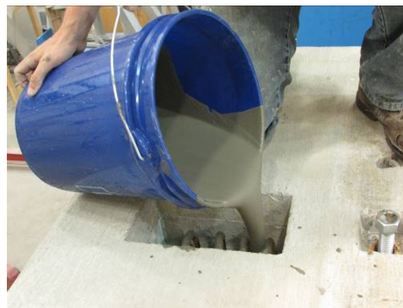
(b) Pouring in Open Pockets
