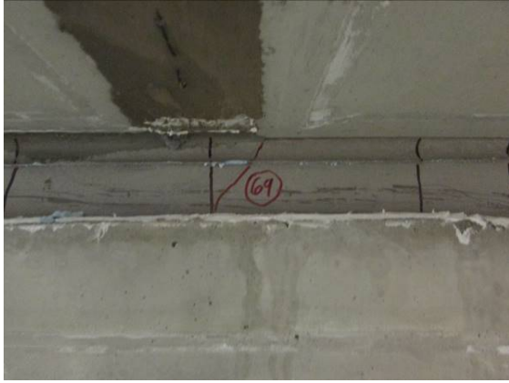
(a) 14-ft North of Mid-Span (Girder A)
