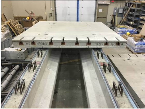
Figure 4.10 Installation for Full-depth Deck Panels on Precast Girders
