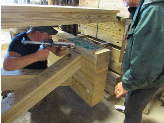
(b) Placement of Epoxy between Girder and Deck
