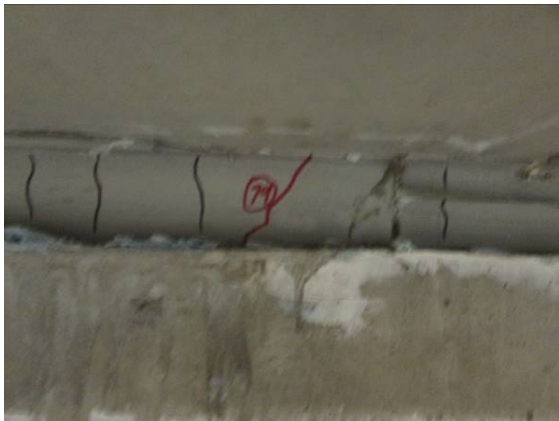
(a) 16-ft North of Mid-Span (Girder B)
