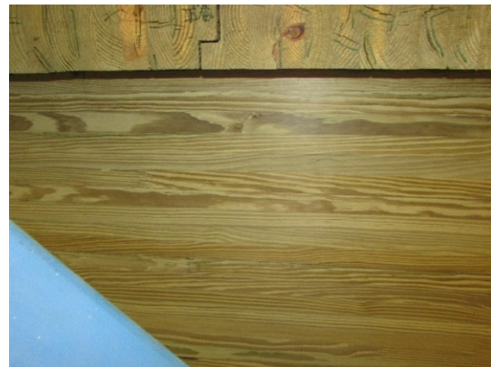
(f) Condition of East Girder at Mid-span
