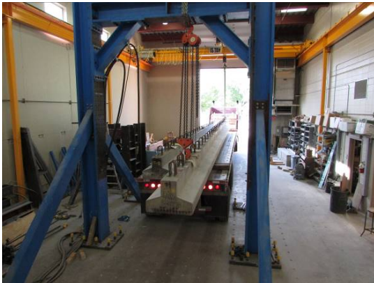
(a) Girder Unloading
