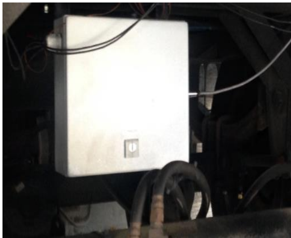
f. Signal Conditioning/Power Distribution Box on Trailer.
