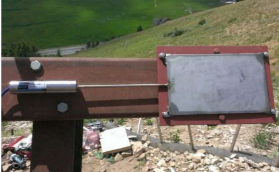
Figure 7 Pressure cell 16 mounted on uppermost crossbeam
