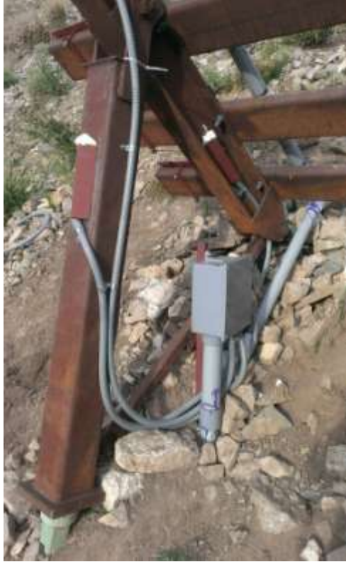
Figure 12 Photograph of SSS strut and girder with vibrating wire strain gage
