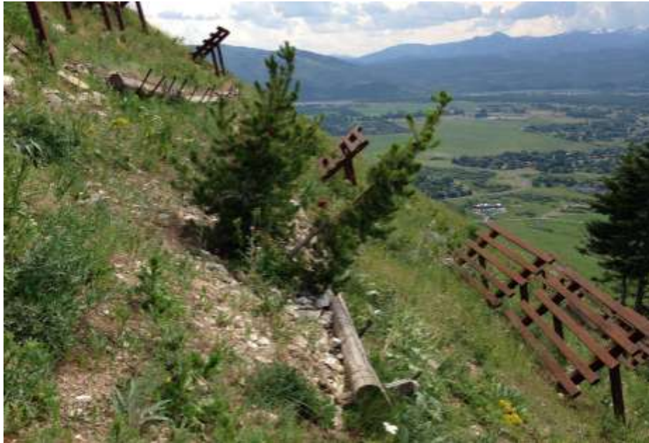
Figure 69 Re-growth of evergreens with failed landscape bench
