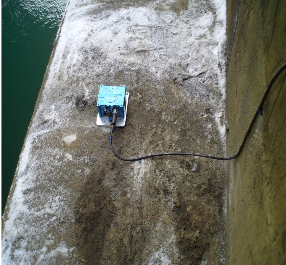
Figure 2 – CX1 Sensor Mounted on Bridge Pier
