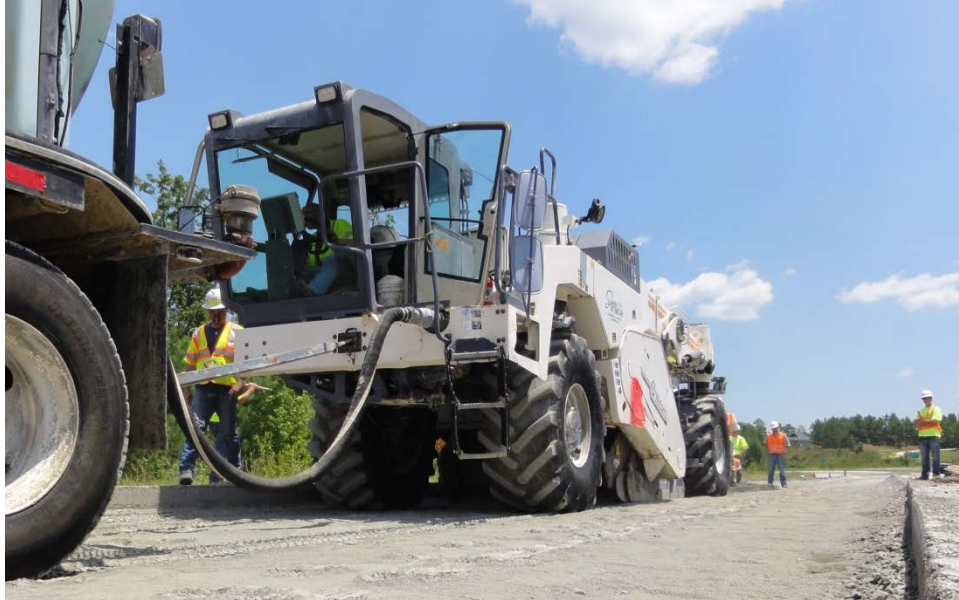
Figure 1. Reclaimer Used for Full Depth Reclamation
