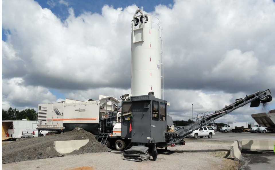
Figure 2. Cold Central Plant Recycling Plant
