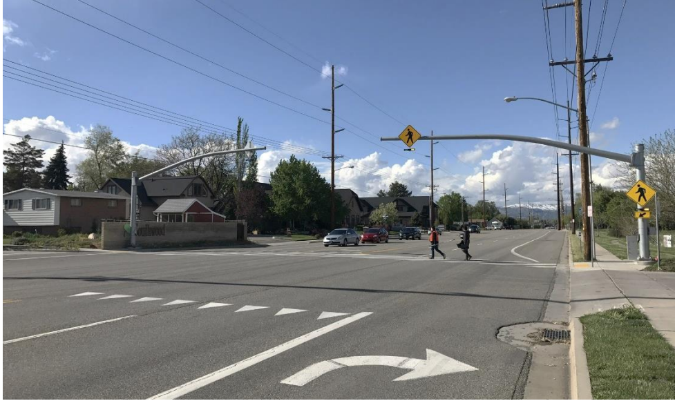
Figure 2.5 ORRFB crosswalk in Murray, Utah.
