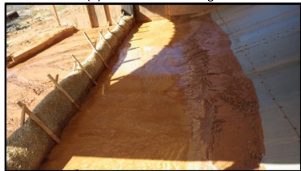
(f) Excel Straw Log sediment deposition
