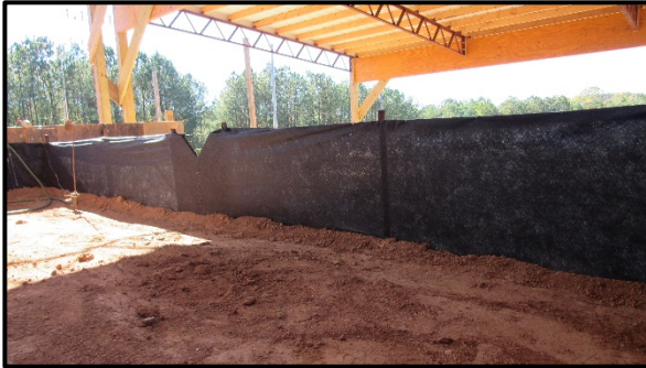
(a) upstream vantage point
