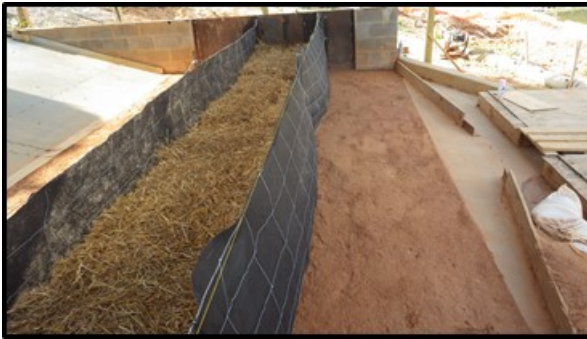
(a) SRB installation
