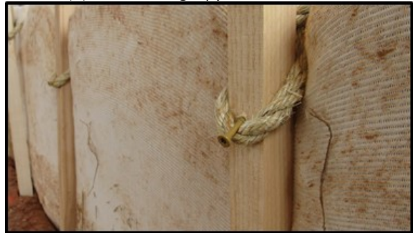
(f) rope installation – wood screw catch
