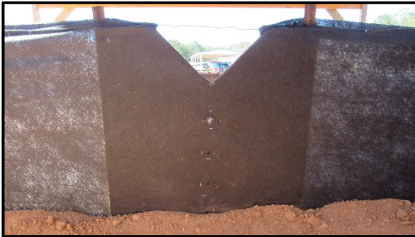
(c) front of weir
