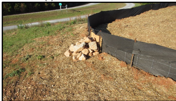
(g) field installation - downstream
