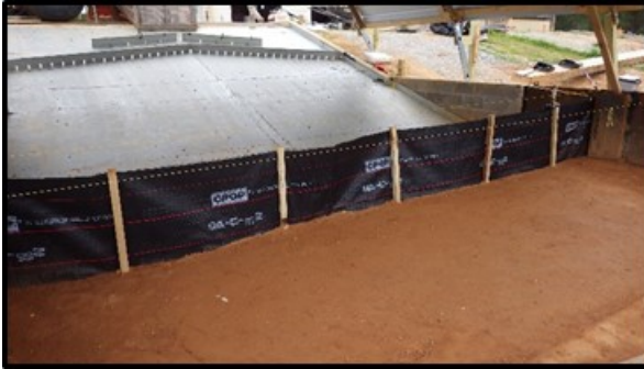
(a) system installation
