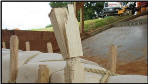
(e) rope installation - broken notched stakes
