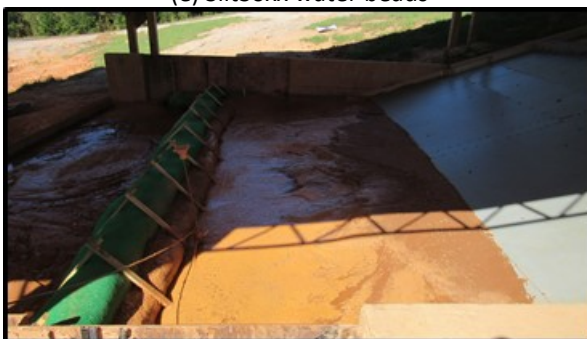
(g) SiltSoxx sediment deposition
