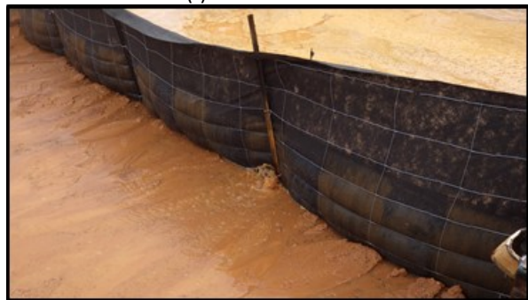
(h) undermining of modification 2
