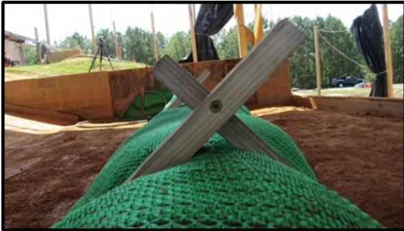
(c) modified teepee installation – wood screw
