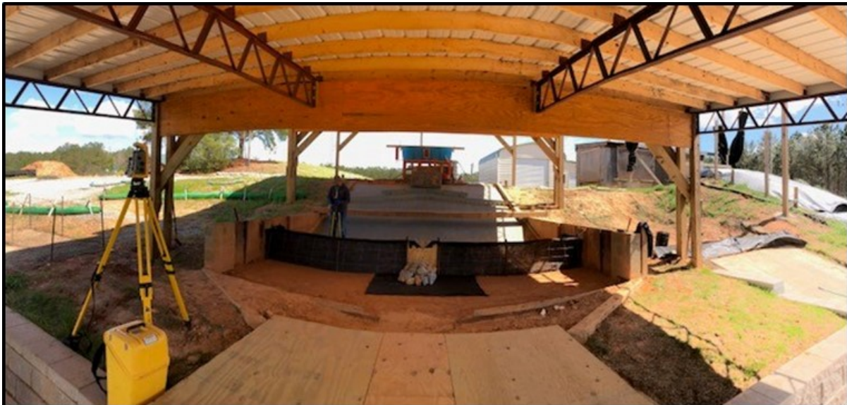
Figure 11. Robotic total station setup and survey.
