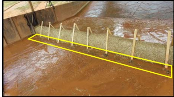
(b) sediment-laden flow - fabric underlay installation
