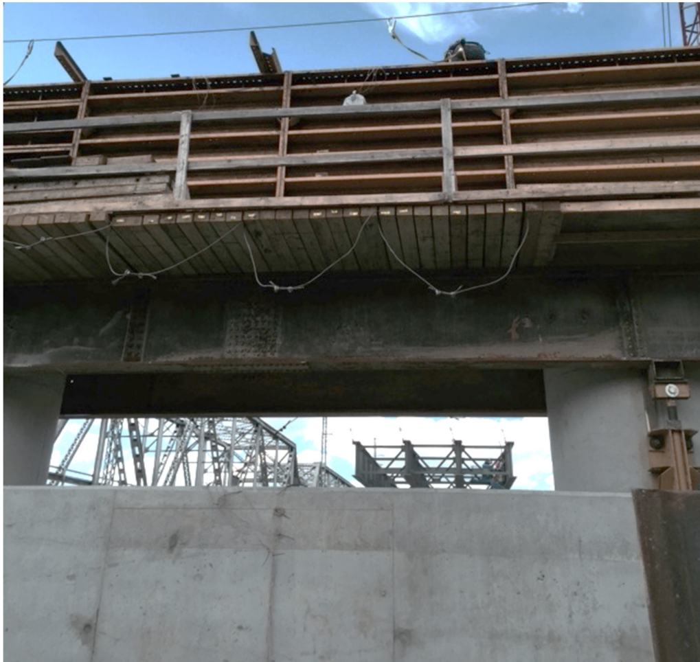
Figure 5-20: Scottsboro bent cap under construction
