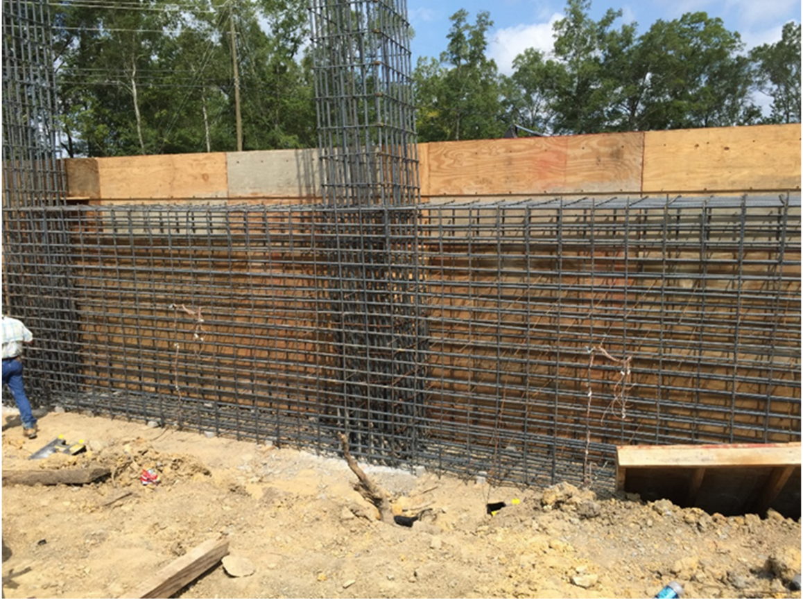
Figure 5-6: Harpersville crashwall under construction
