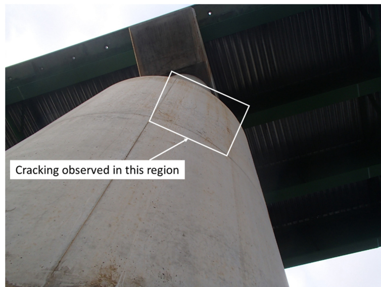
Figure 5-18: Scottsboro pedestal cracks observed at top of pedestal (unreachable)
