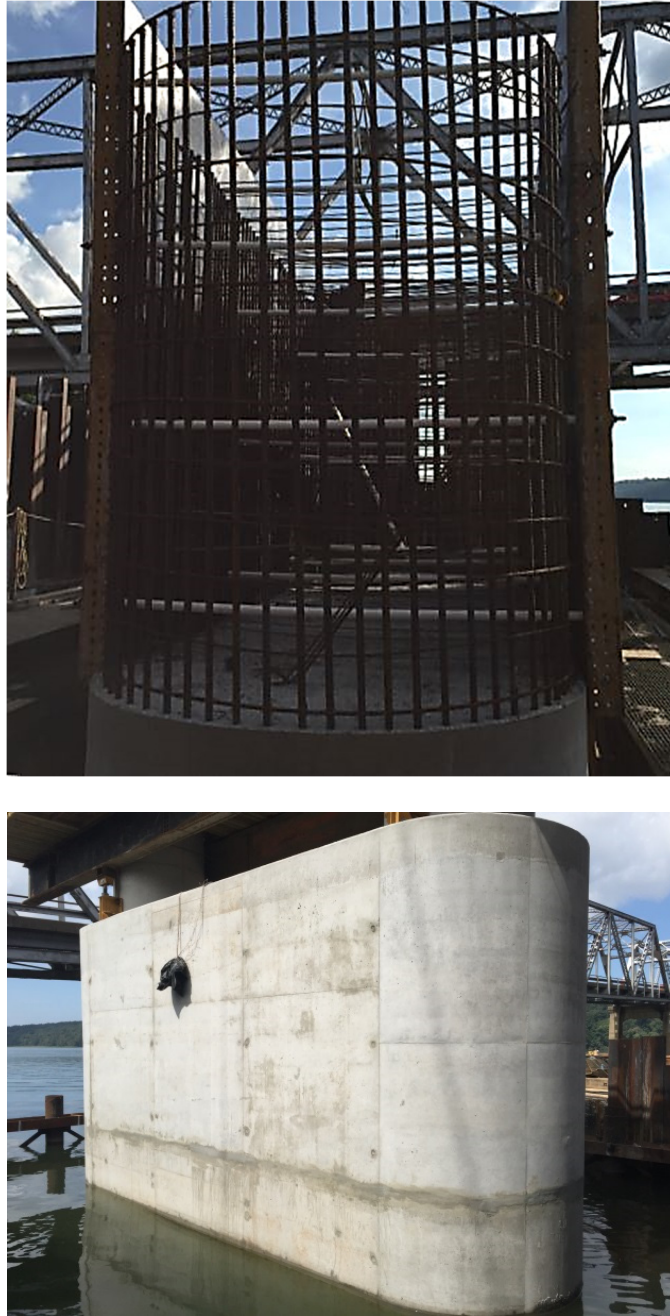
Figure 5-11: Scottsboro pedestal prior to placement (top) and post construction (bottom)
