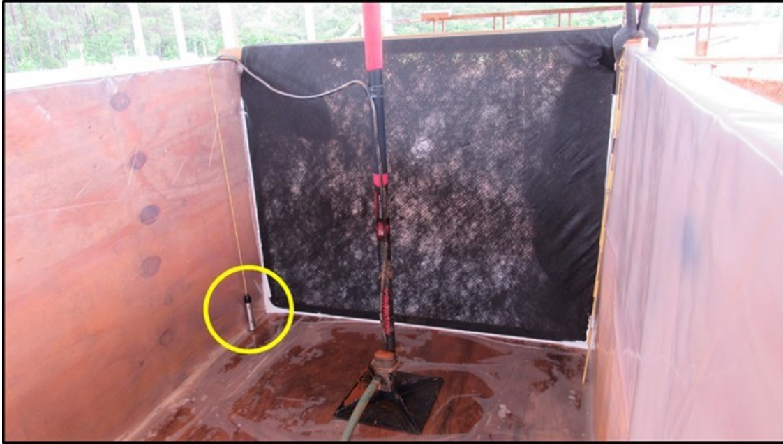
Figure 7. Upstream water level logger installation location.
