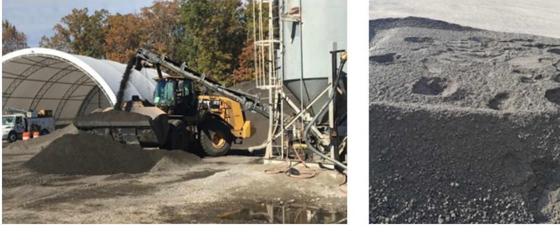
Figure 1. Processed CCPR Mixture: (Left) loader collecting the processed mixture; (Right) the processed mixture pile. CCPR = cold central plant recycling.
