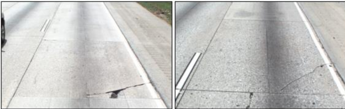
Figure 2.7 Examples of corner break
