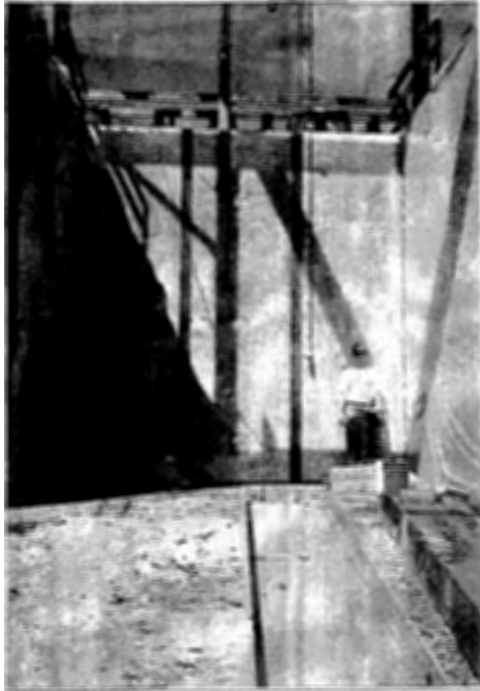
Figure 3.4 Photograph of front wall
