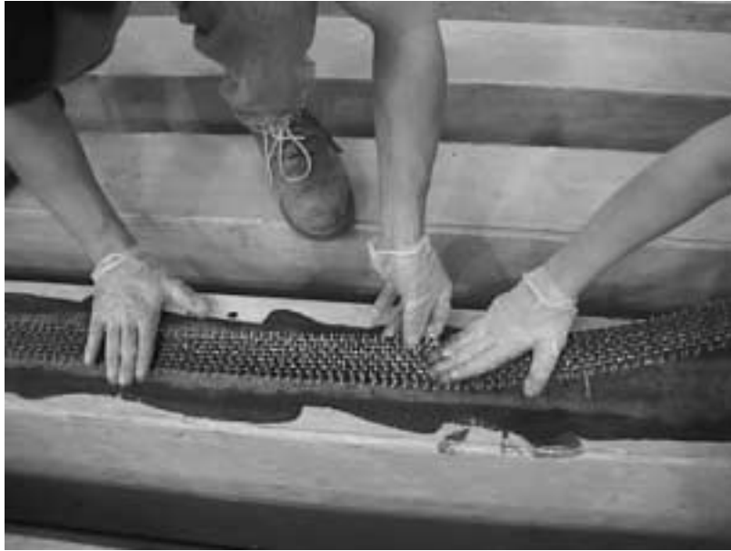
Figure 4.5 Composite System C: Woven Unidirectional Carbon Fibers
