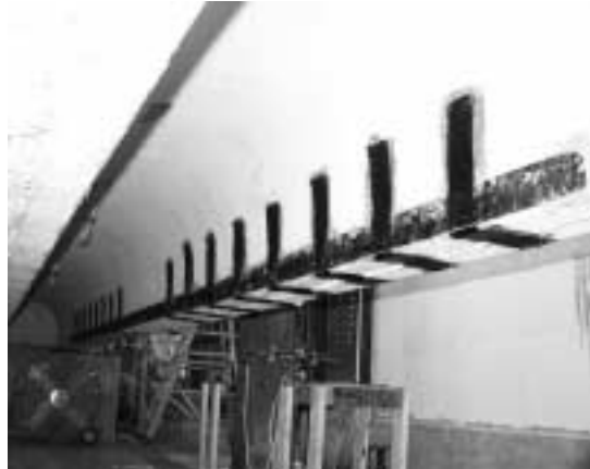
Figure C.3 Application of Woven Straps Around CFRP Pultruded Plates
