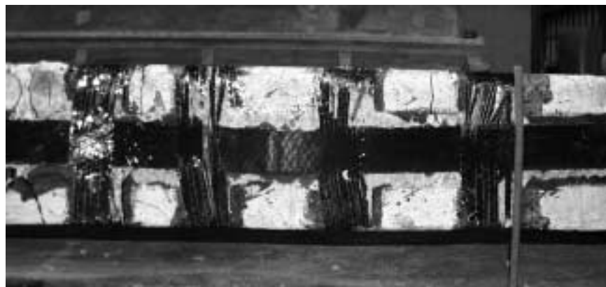
Figure 8.2 View of Tension Face of Specimen A-F2 after Debonding
