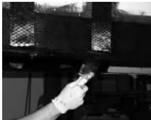
f) Coating sheets with epoxy
