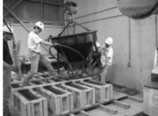
(c) Placing concrete in forms
