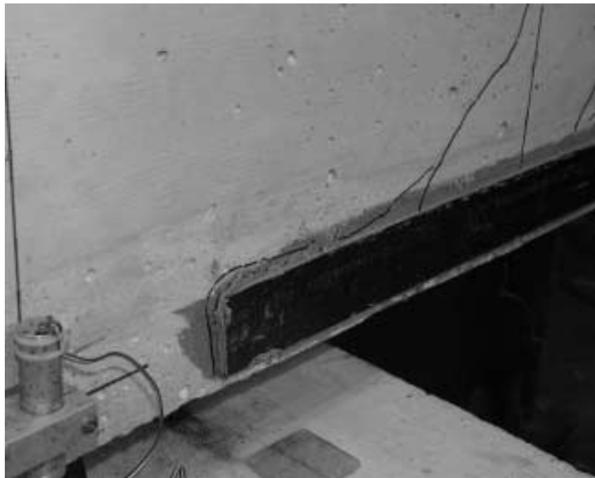
Figure 6.17 Debonding at the End of the CFRP Composite Plate in Specimen D4
