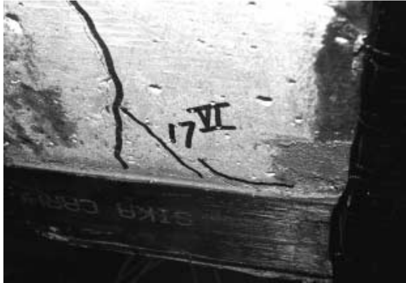
Figure 8.10 Local Debonding of CFRP Plate on Specimen D-F2 during Fatigue Cycling
