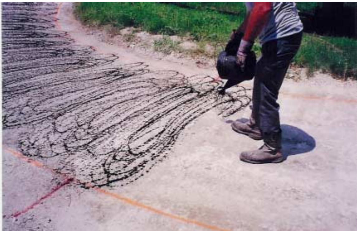
Photograph 5.13 Application of The Primer Coat.
