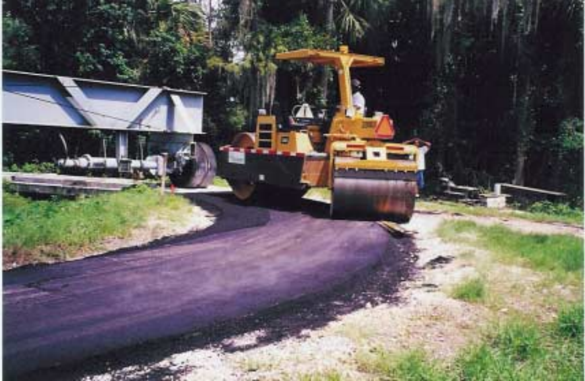
Photograph 5.16 Asphalt Compaction.
