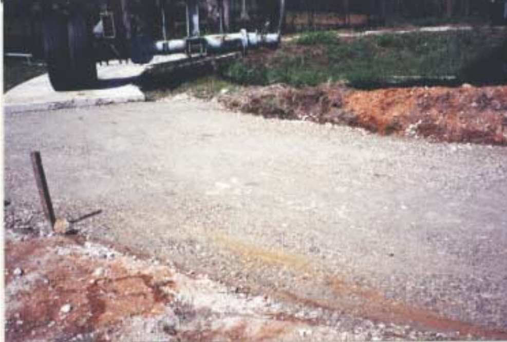
Photograph 5.7 Finished RCA Base Course (Sections 1 & 2).
