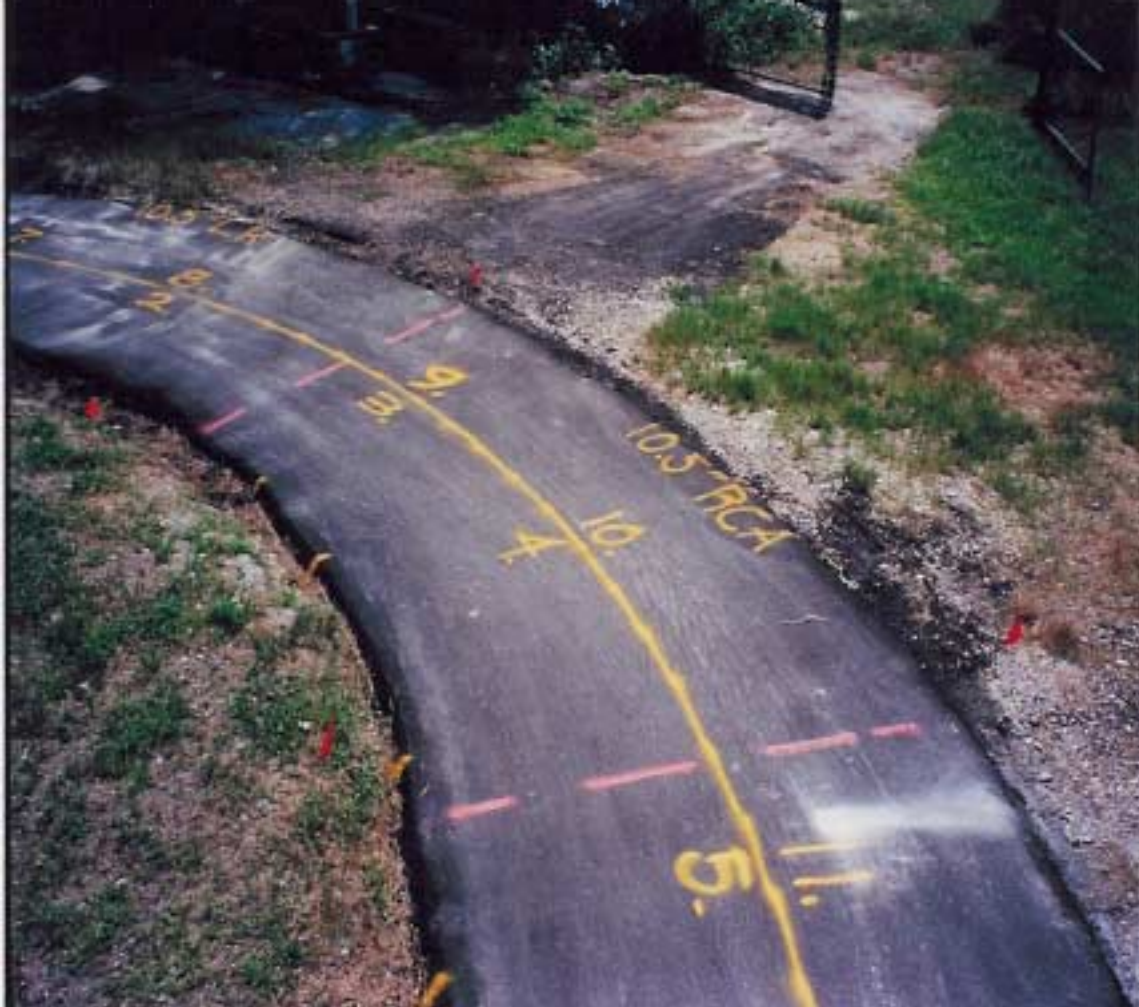
Photograph 5.18 Test Section Identification.
