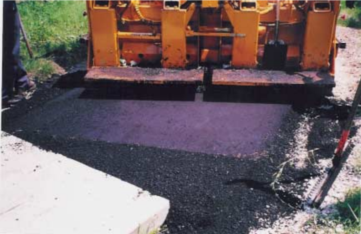
Photograph 5.14 Asphalt Layout by Paver.
