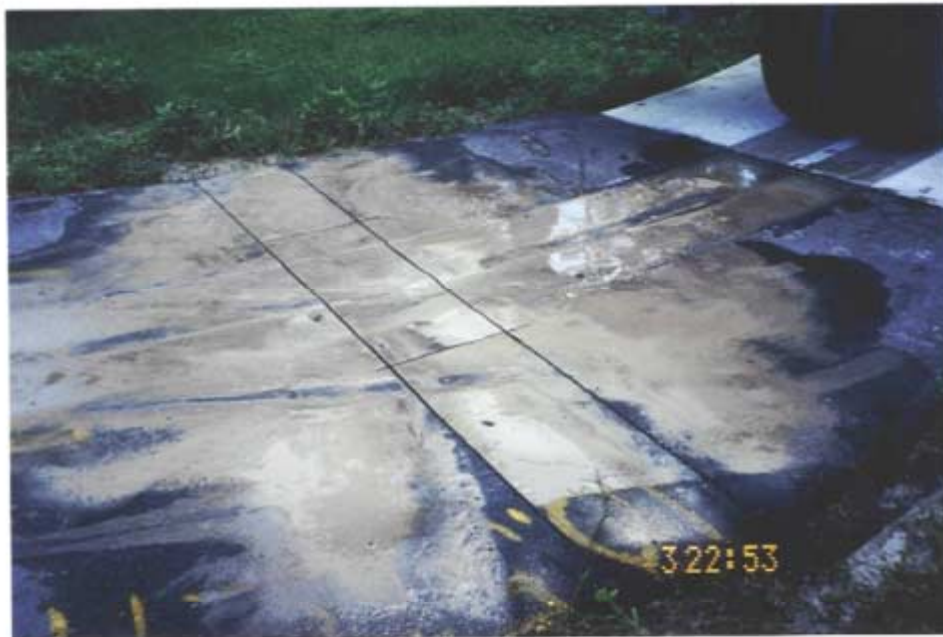
Photograph 6.3 Saw Cut of Pavement Sections
