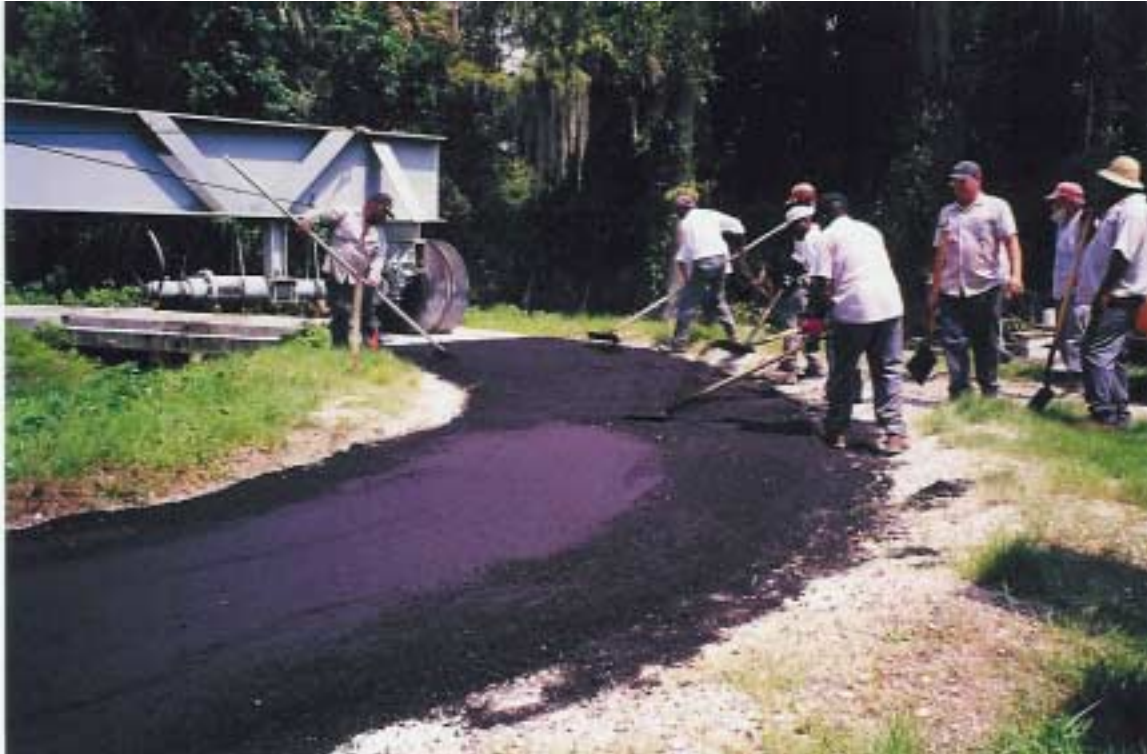
Photograph 5.15 Spreading Asphalt.
