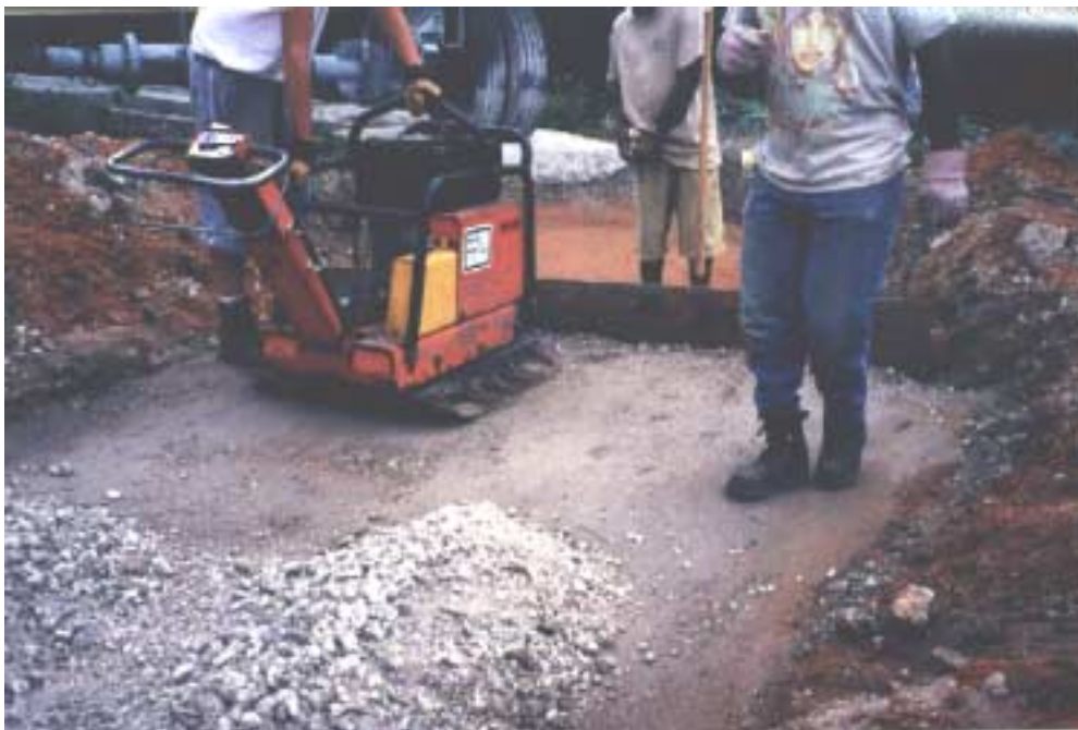
Photograph 5.6 Compacting RCA Base Course.
