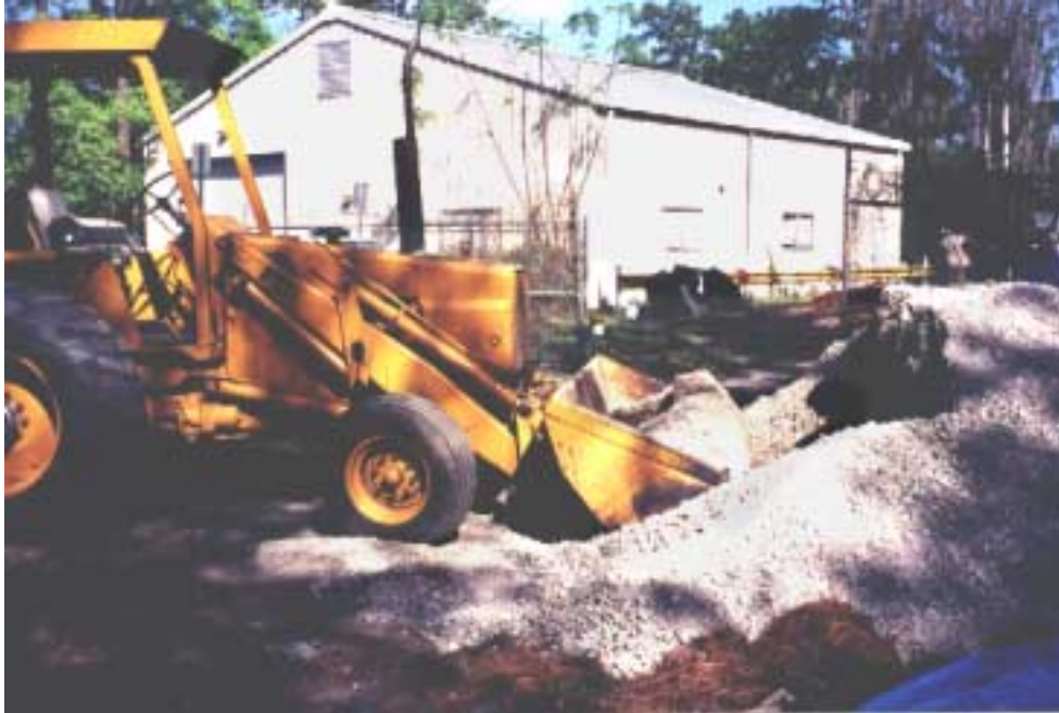
Photograph 5.3 Placement of RCA by Backhoe.
