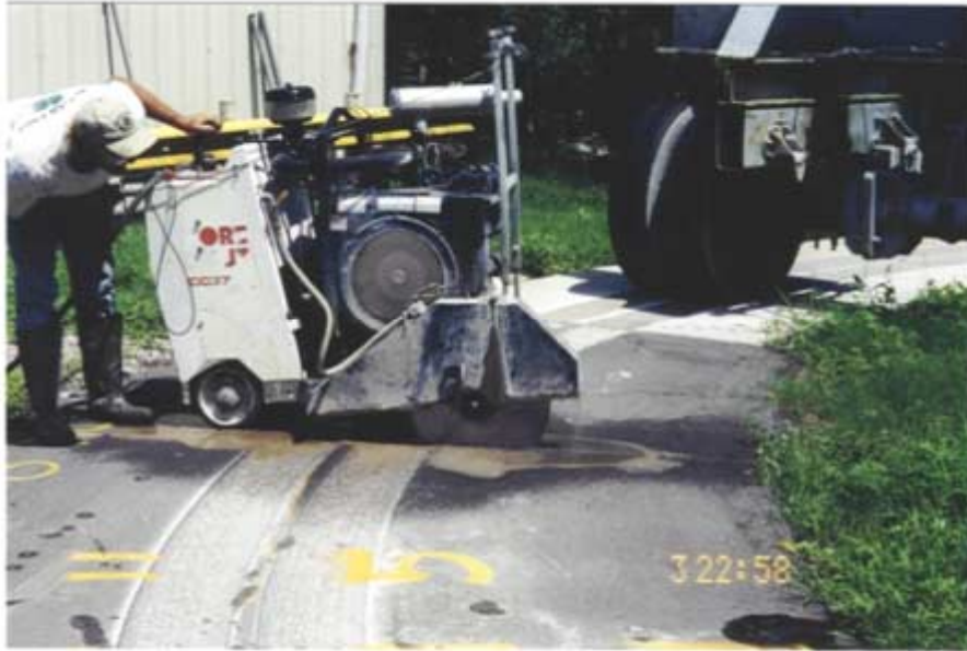
Photograph 6.2 Saw Cut Machine
