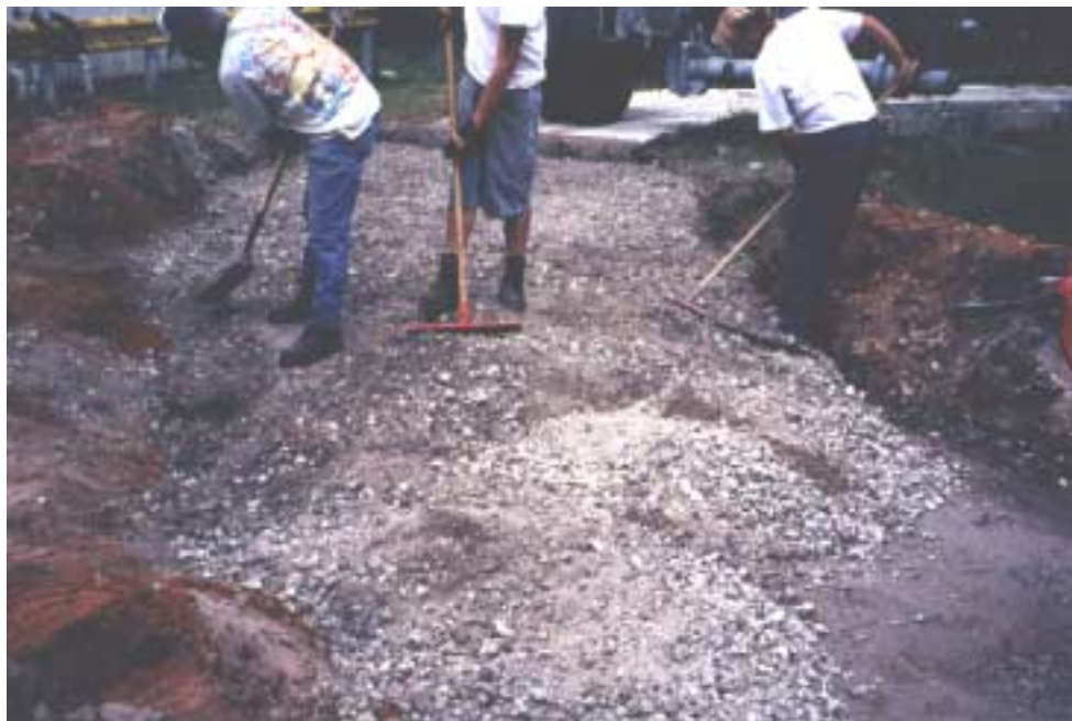
Photograph 5.4 Spreading of RCA.
