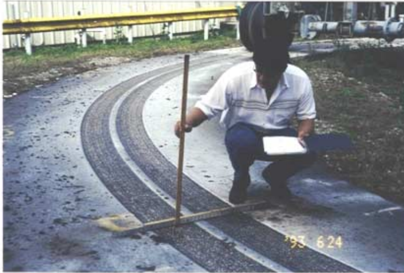
Photograph 5.19 The Rutting Measurements in Test Sections.
