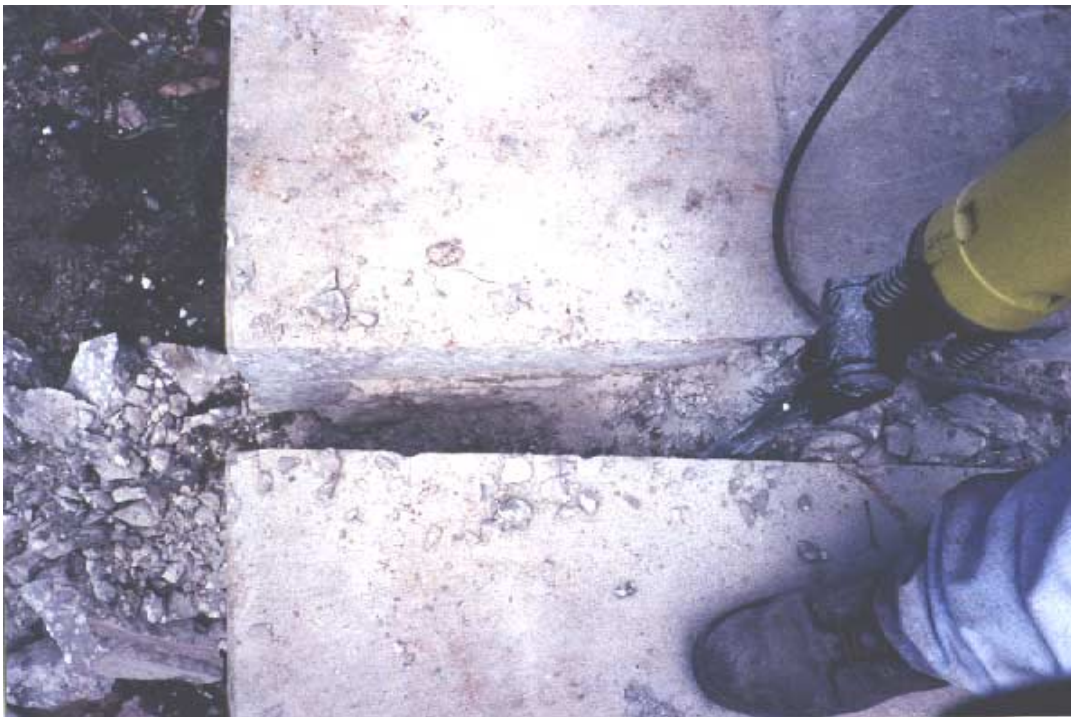
Photograph 5.2 Concrete Slab Section being cut using a Jack Hammer.
