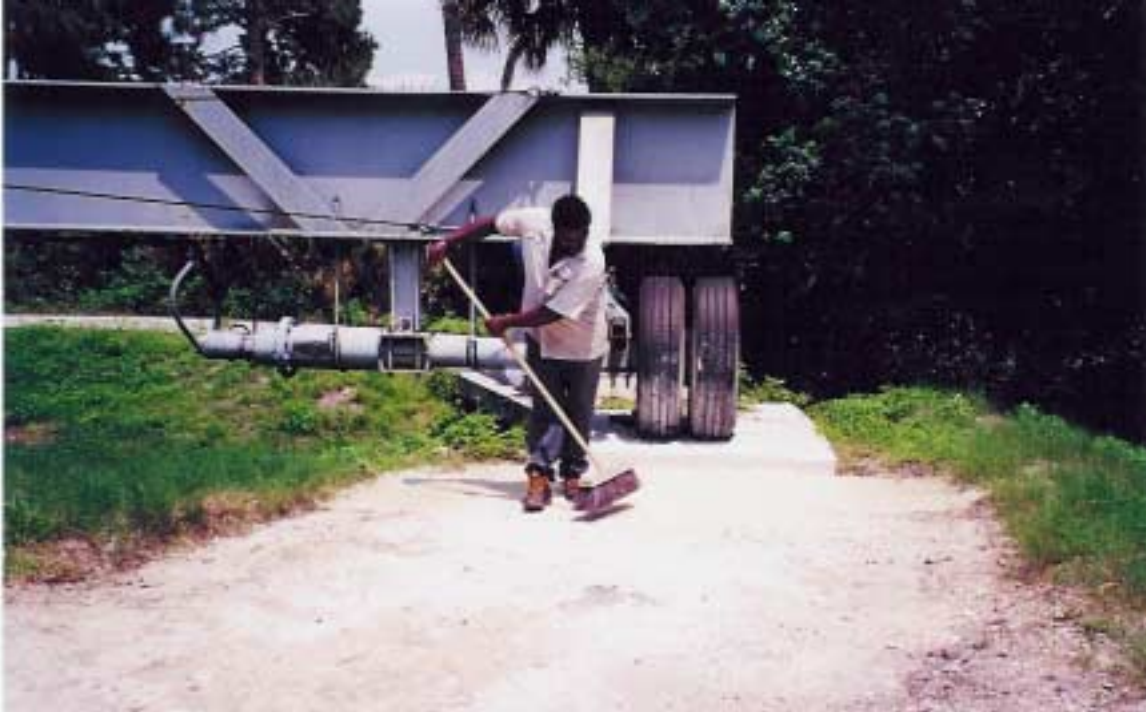
Photograph 5.12 Base Course Surface Cleaning.
