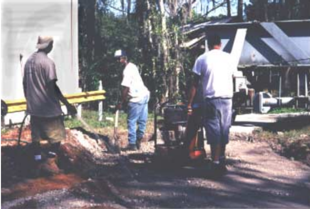
Photograph 5.5 Watering of Material During Compaction.
