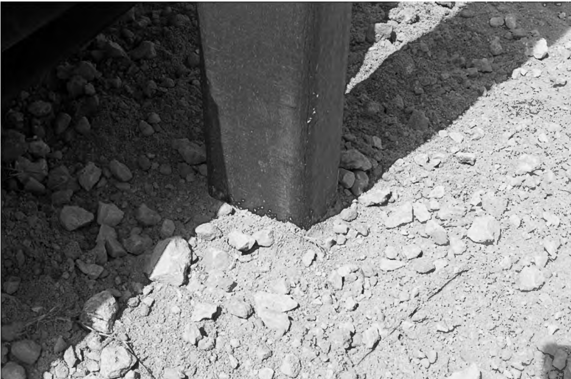
Figure 39. Recycled Plastic Sign Support Before Test 414588-3.
