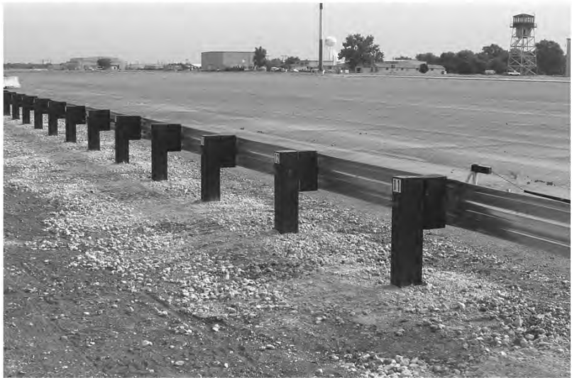
Figure 48. Plastic Post W-Beam Guardrail Installation Before Test 414588-1.
