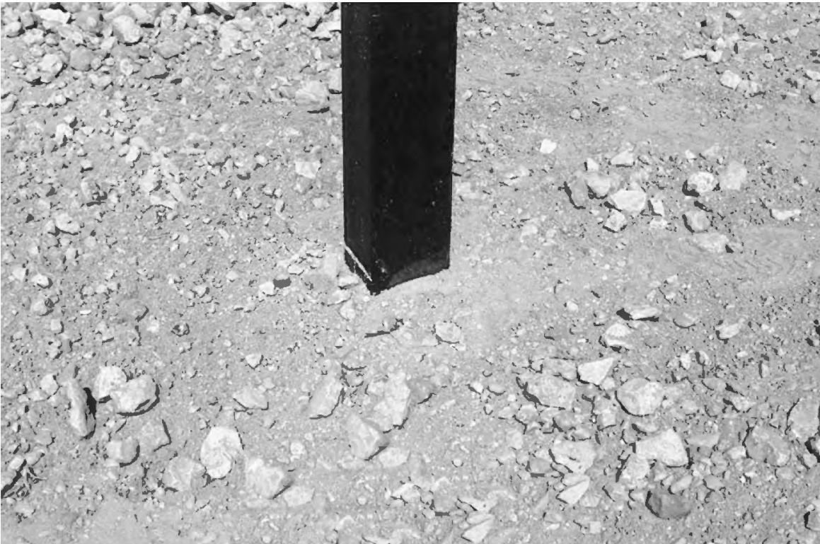
Figure 25. Recycled Plastic Sign Support Before Test 414587-4.
