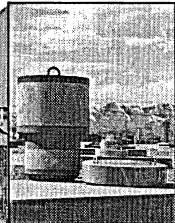
CPP-749 Dry Well Storage Area
