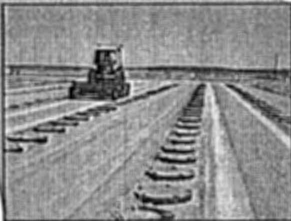
ANL-W Radioactive Scrap and Waste Facility
