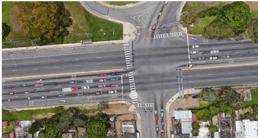
Figure 3.3 - Plan view of the intersection PR-2 and Nenadich street. Source: Google Maps
