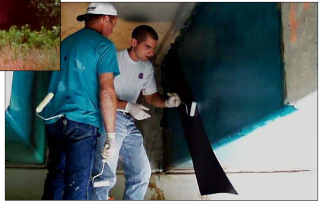
Photographs show: the bridge type that can benefit from CFRP retrofit, the typical nature of concrete beam cracking, and the application of the advanced composite laminates.
